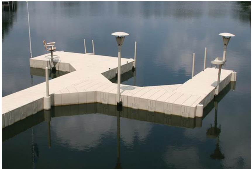
Figure 4.12 Dock Installed by Northwood Dock and Service
