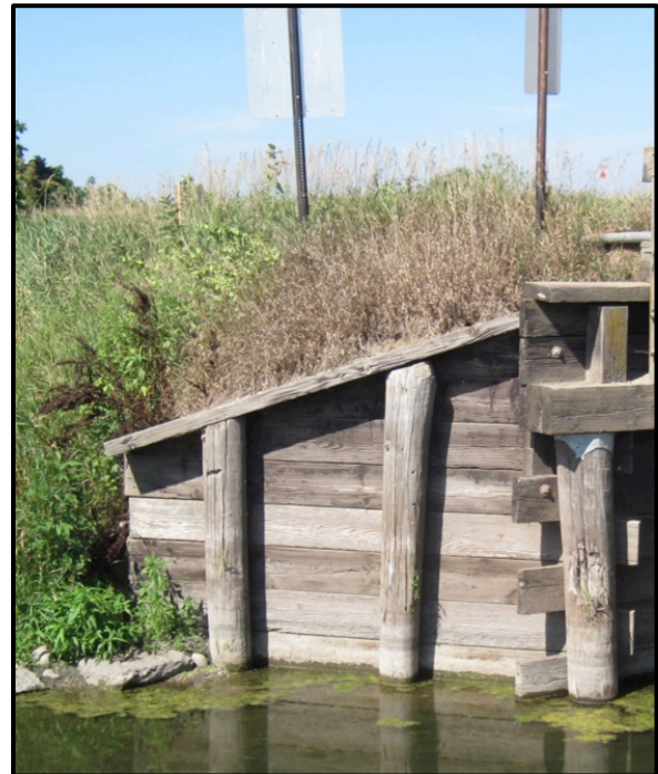
Figure 1.8. Timber piling, piling and cap board forming a timber wingwall.
