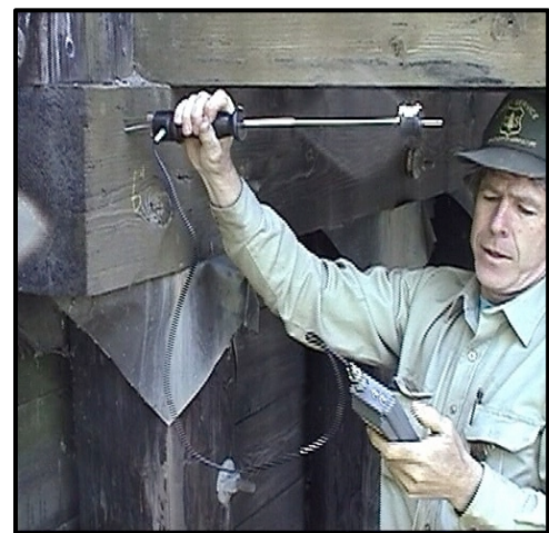
Figure 4.4. A pin style moisture meter is used to determine moisture content of timber elements.
