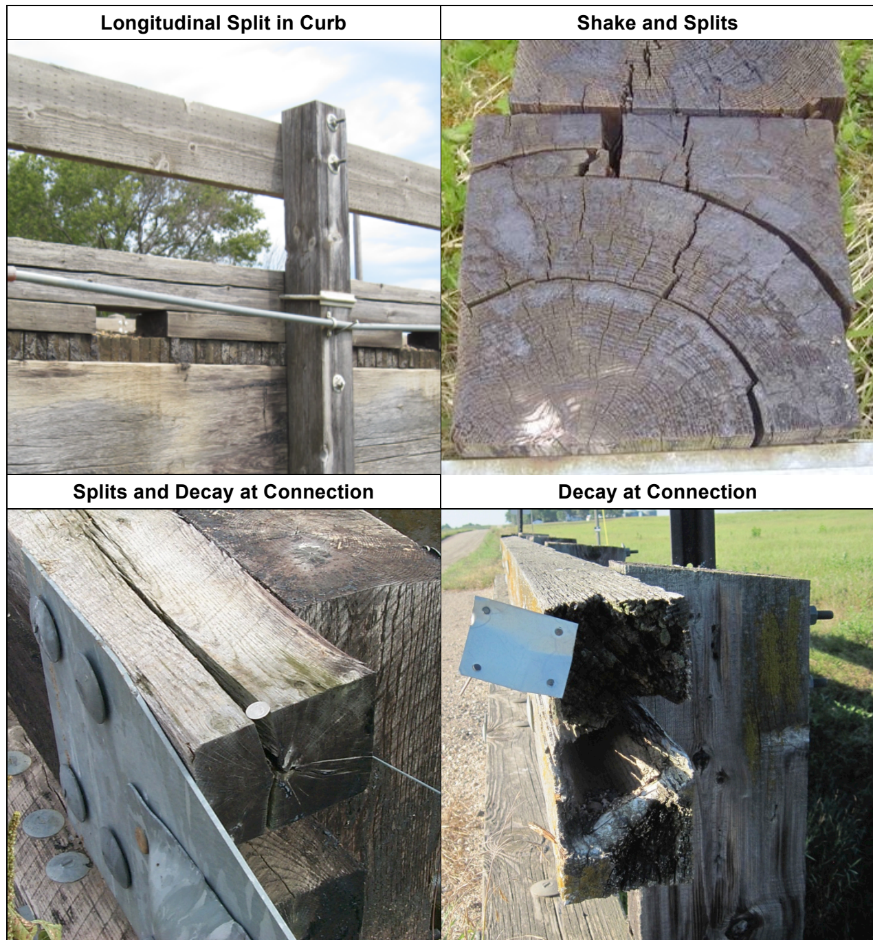
Figure 7.4. Examples of deterioration of timber railing components.
