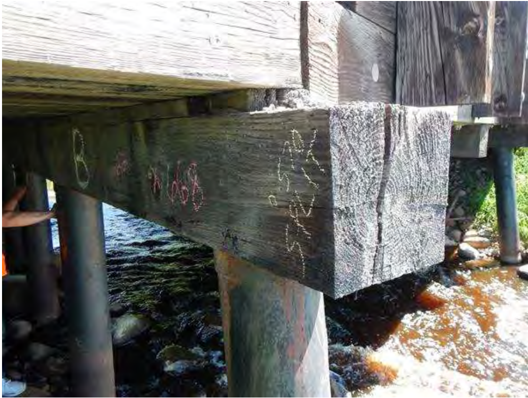
Photo 7 - Pier 1 - South End - Through split extending 36"
