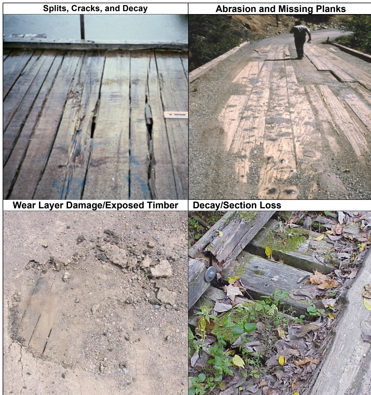
Figure 7.3. Deterioration of timber decks and slabs.
