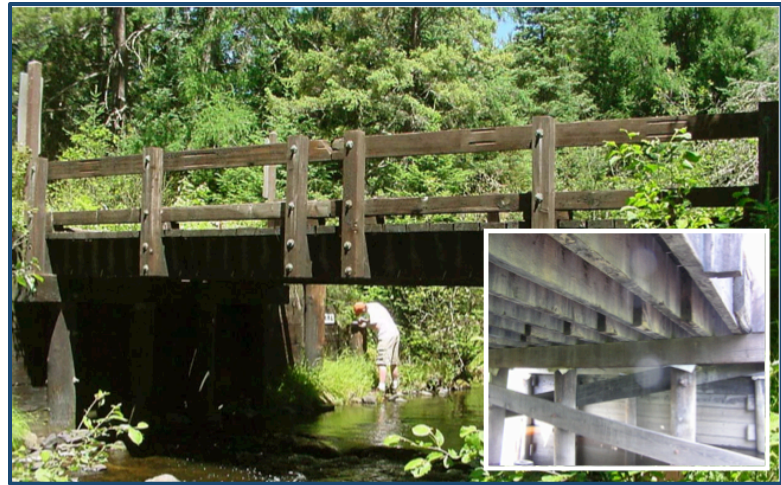
Figure 1.1 Typical solid-sawn beam style timber bridge.
