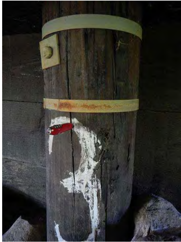
Photo 11 - W. Abut. Pile 3
