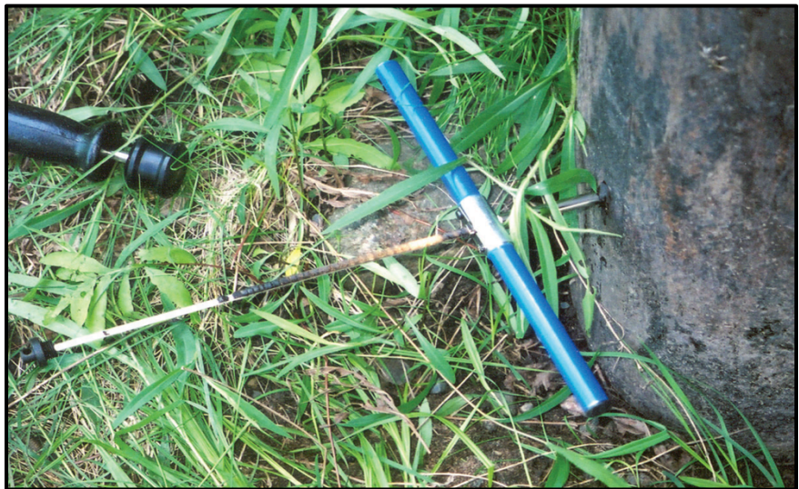
Figure 6.1. An increment core can be used to conduct inspections of timber bridge elements. This image shows an extracted core from an in-service timber pile ready for examination.
