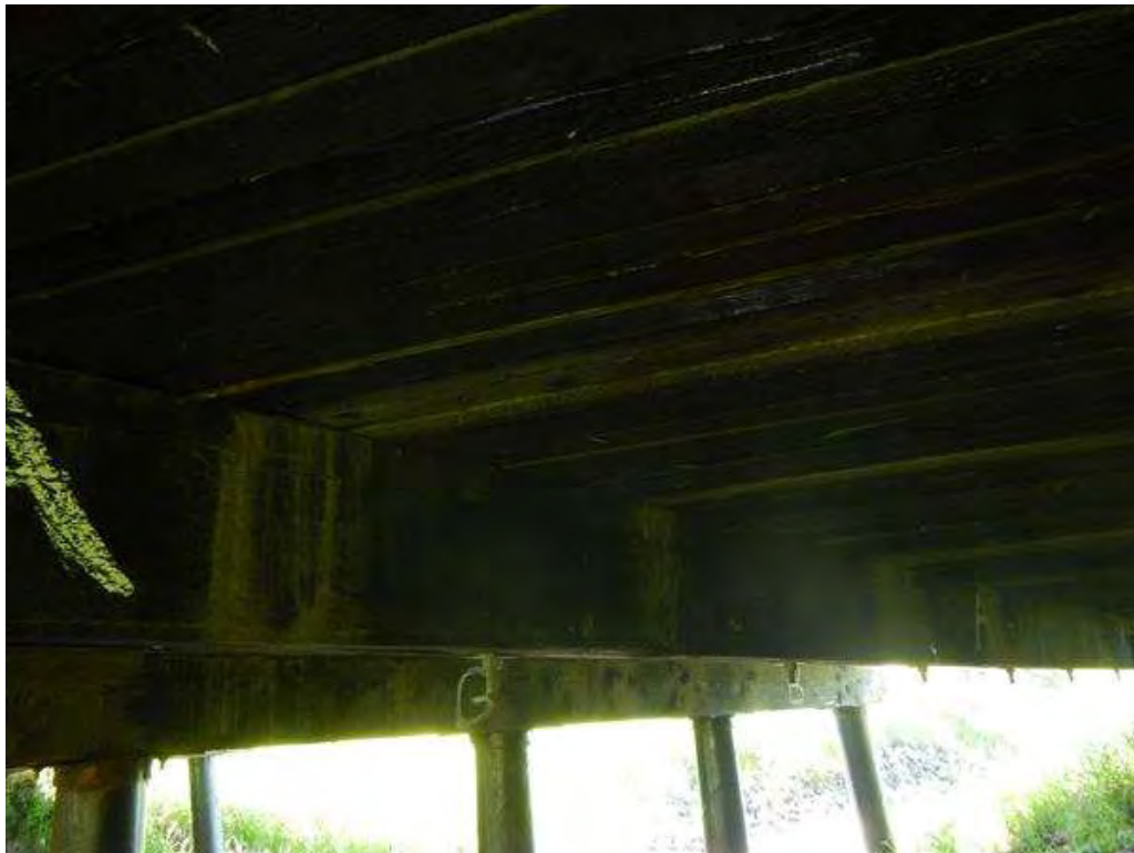
Photo 8 - Span 1 - Moisture pen. through deck.
