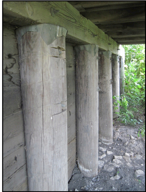
Figure 1.6. Timber piling and backwall forming a timber abutment.
