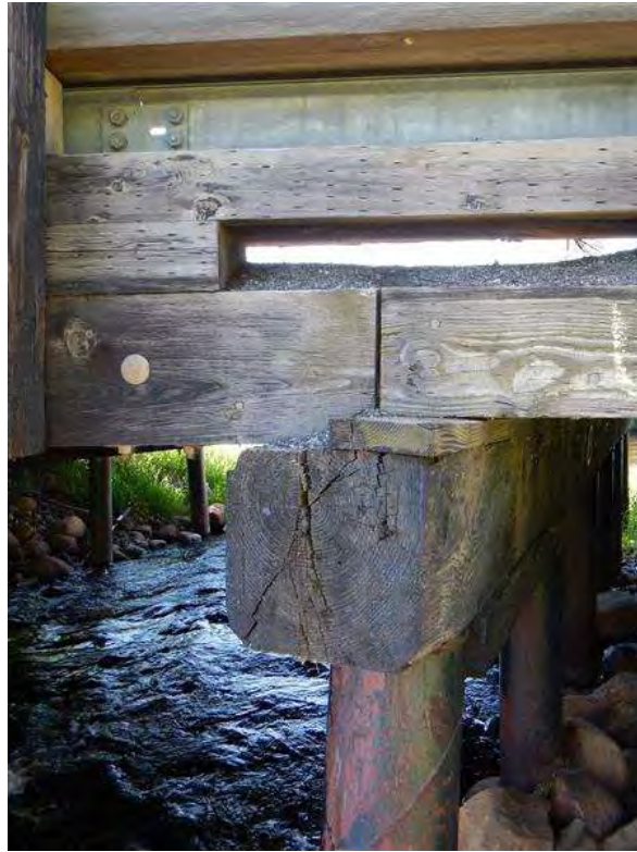
Photo 9 - Pier 2 - South end - Through split continuing 24 inches into cap.
