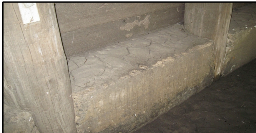
Figure 3.23. Timber piling in direct contact with concrete footing, creating high moisture content conditions.
