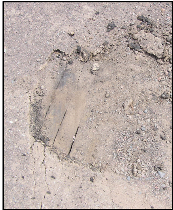
Figure 3.17. The bituminous wear layer has deteriorated exposing structural timber decking to moisture and potential deterioration.
