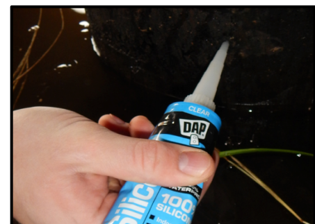
Figure 6.7. Silicone is used to fill the small drilling hole.
