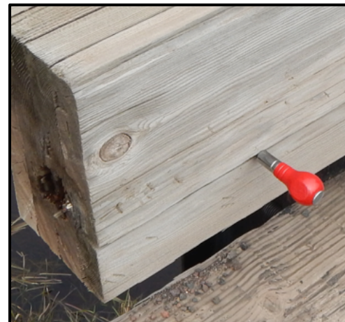
Figure 4.2. An awl is used to assess the depth and presence of decay in a horizontal split.
