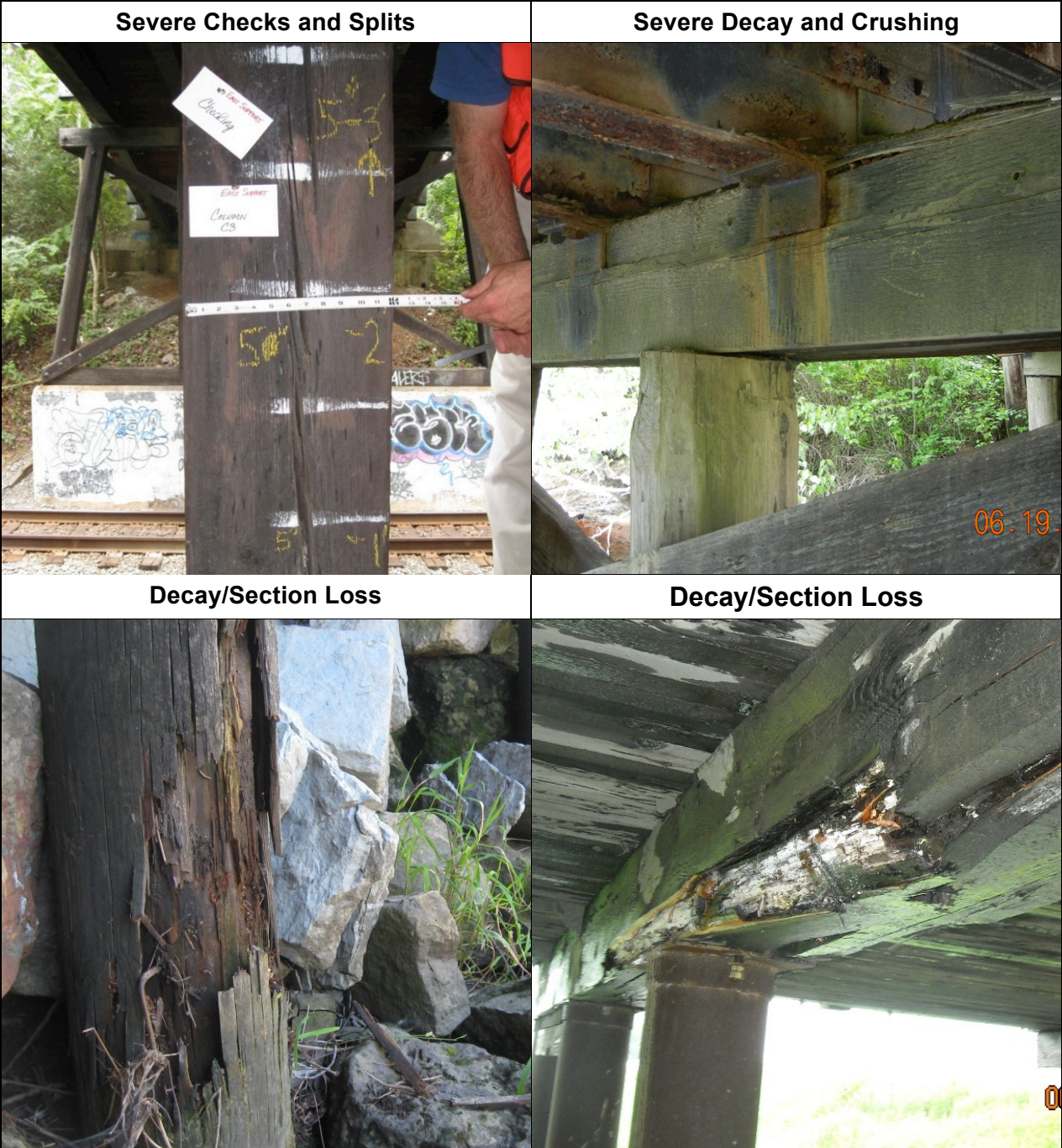
Figure 7.7. Examples of deterioration of timber substructure elements.
