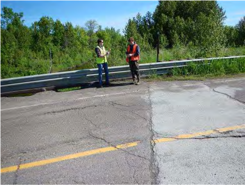
Photo 3 - Bituminous east end before abutment
