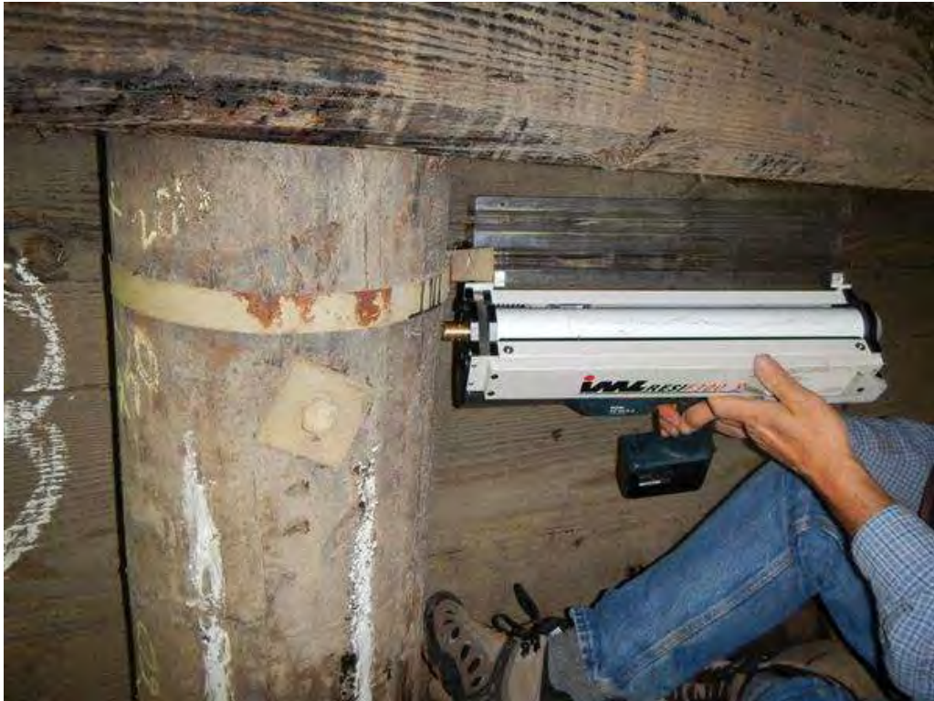
Photo 14 - E abut - Pile 11 - Sound condition
