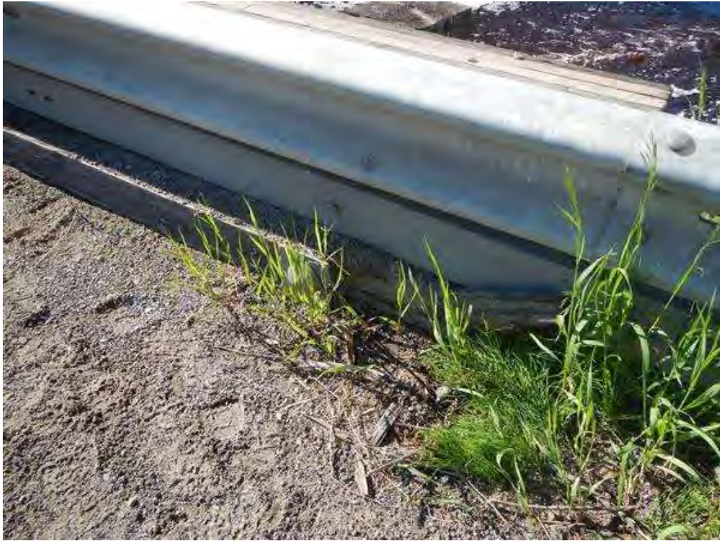
Photo 5 - SW corner of bridge showing vegetation and gravel/sand near curb. Deterioration noted.
