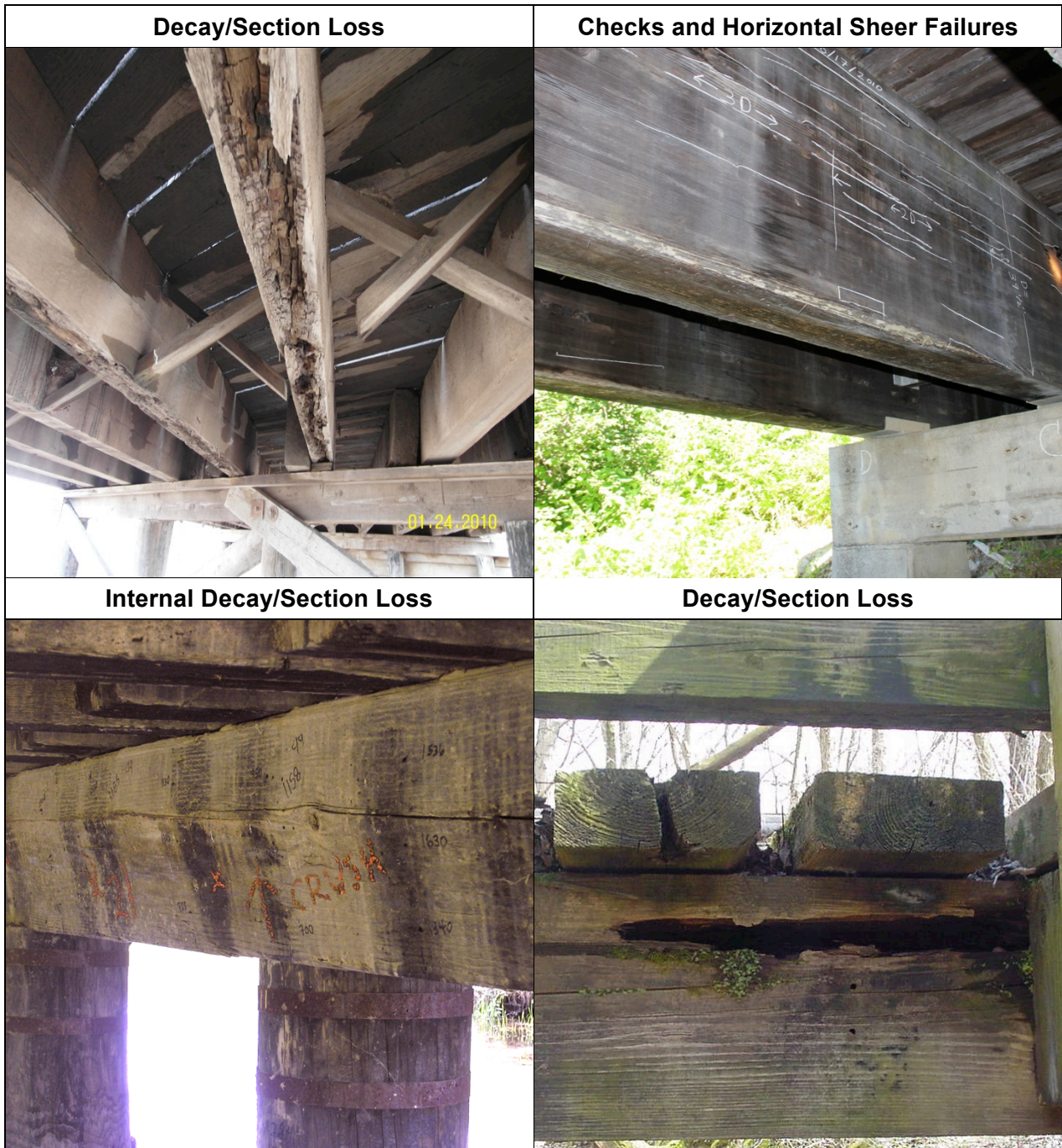
Figure 7.5. Examples of deterioration of timber superstructure elements.
