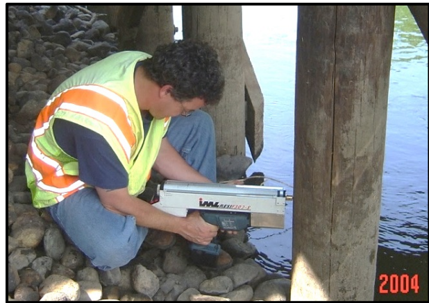
Figure 6.2. A resistance microdrill is the preferred drilling inspection technique for timber bridge elements.
