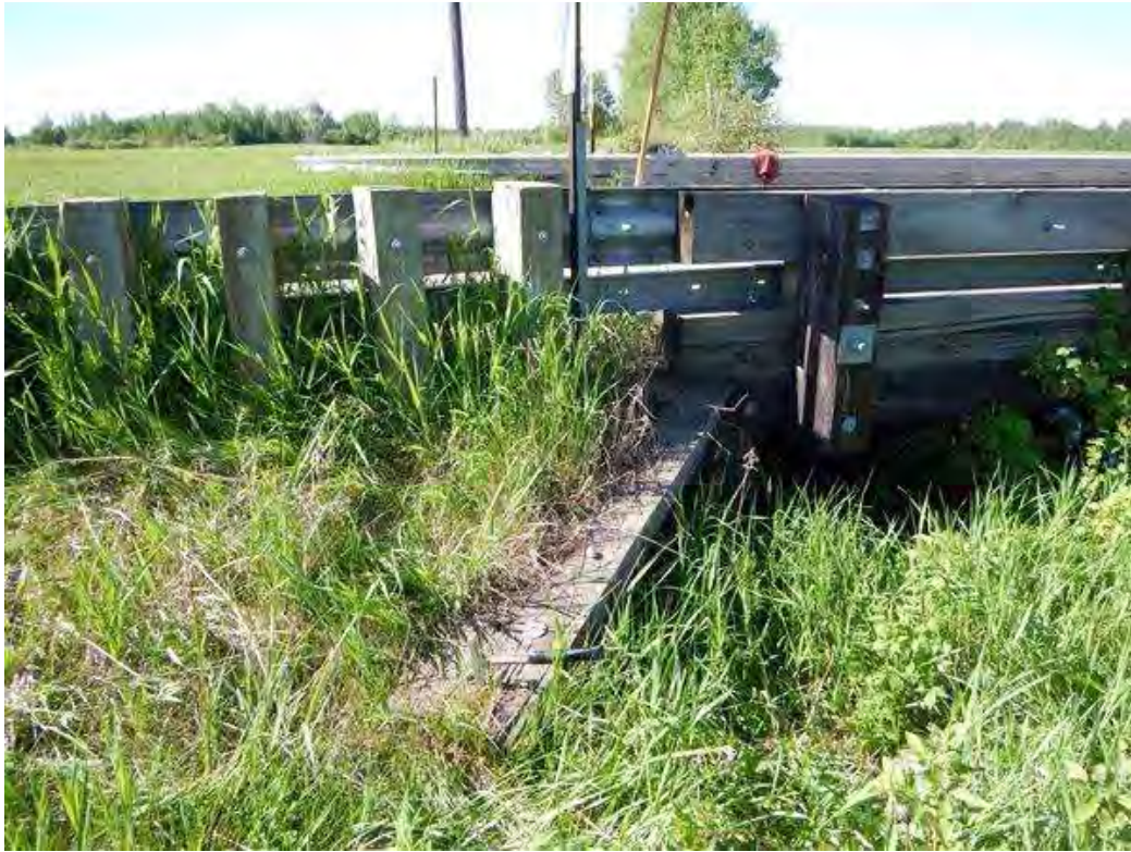
Photo 17 - Wing wall with significant vegetation
