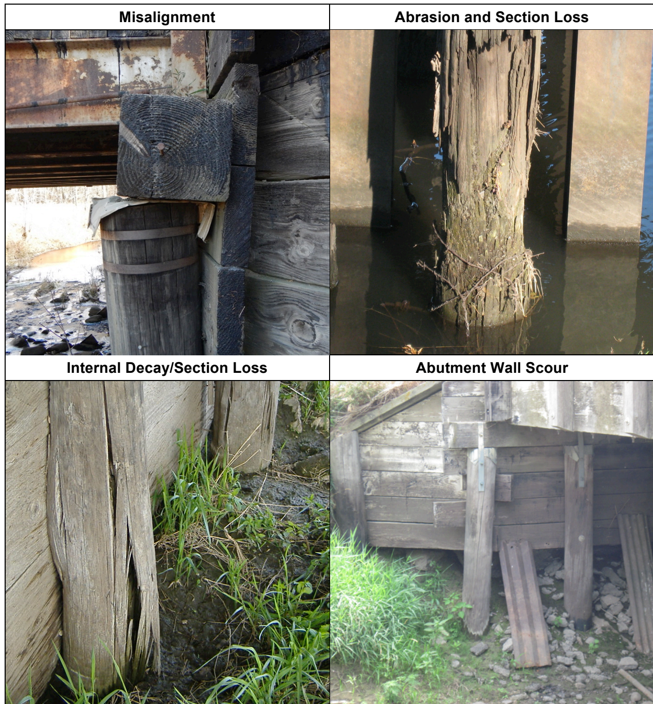
Figure 7.6. Examples of deterioration of timber substructure elements.
