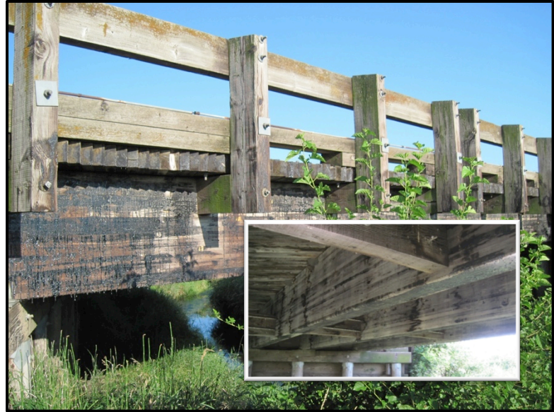
Figure 1.2 Glulam beam timber bridge construction.
