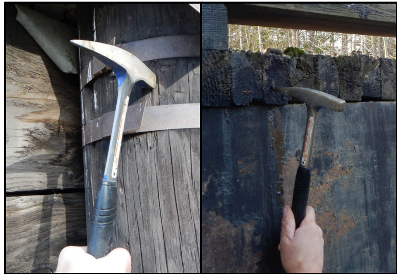
Figure 4.1. A hammer pick is an effective tool for initial assessments of timber bridge elements.
