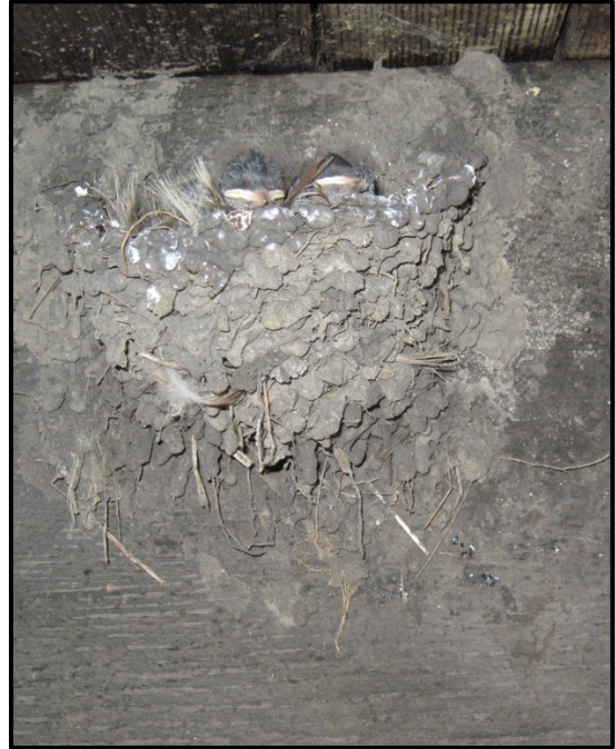
Figure 3.9. Nesting birds are often found under timber bridges and their nests can trap and hold moisture against timber beams and bracing.
