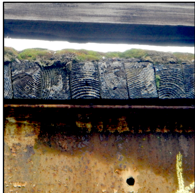
Figure 3.10. Moss growing on the surface of a nail laminated timber deck supported by steel beams along the curb/scupper zone.
