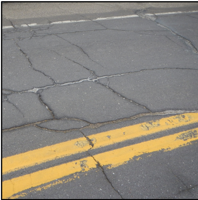
Figure 3.16. Cracking and deterioration of bituminous wear layers create opportunities for water to pond on the deck and seep into the superstructure elements creating decay potential.
