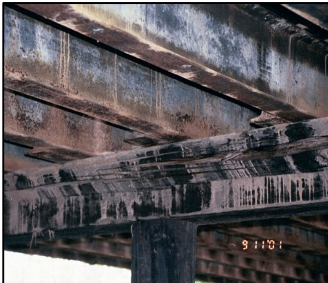
Figure 3.4. Timber abutment cap showing visual evidence of localized failure demonstrated by longitudinal cracking. Photo courtesy of MnDOT.
