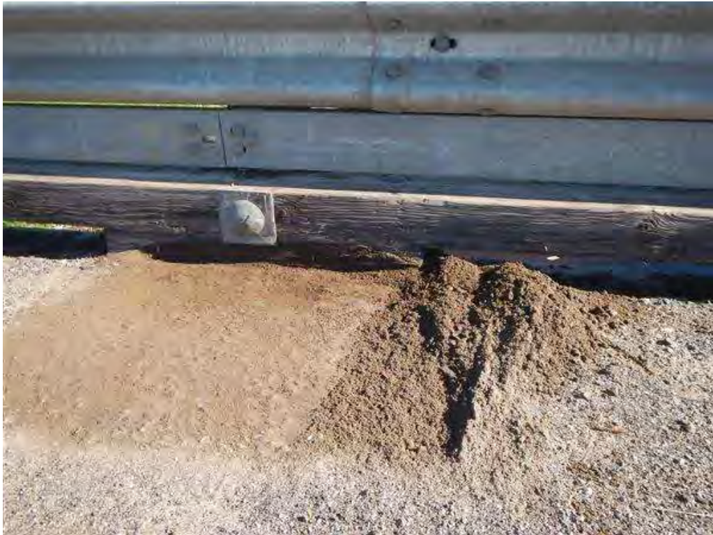
Photo 4 - N. deck-scupper 3" sand on deck
