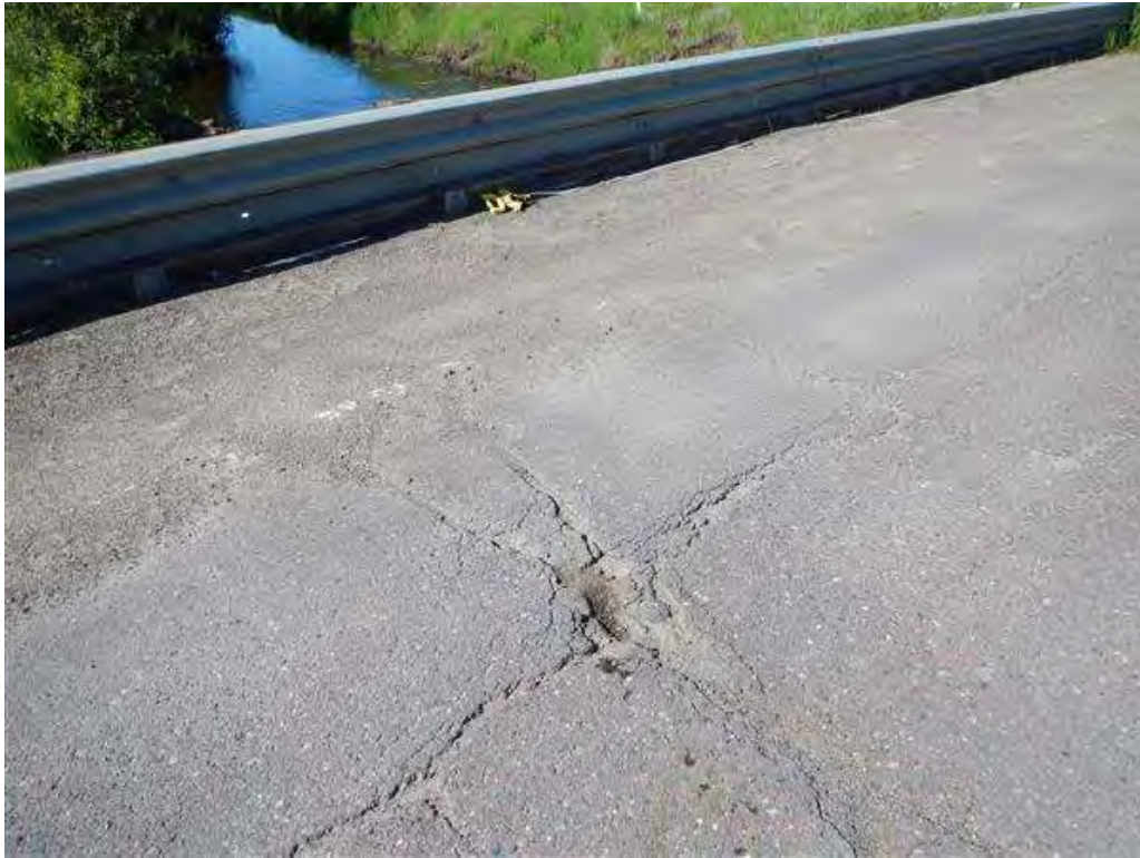
Photo 2 - Deck - Pot hole above Pier 2 with longitudinal cracking
