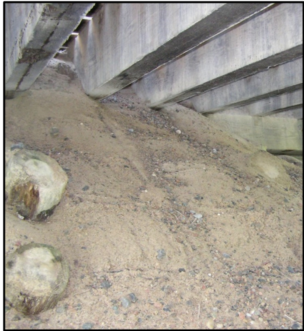
Figure 3.22. Sand and gravel are covering the timber abutment cap and the longitudinal timber beams, holding moisture against these elements.
