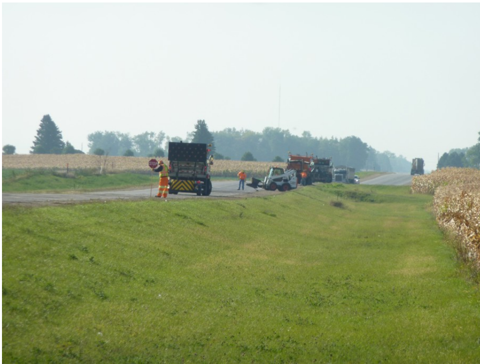
Figure 5.5 View of Work Zone
