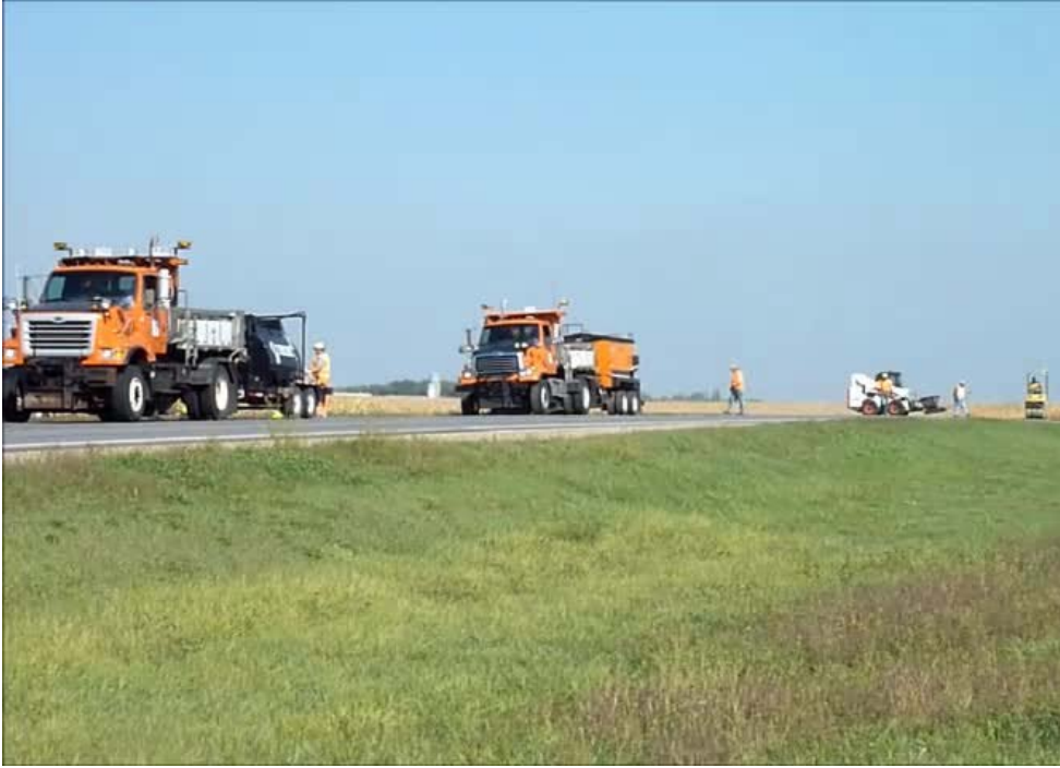
Figure 5.8 View of Work Zone
