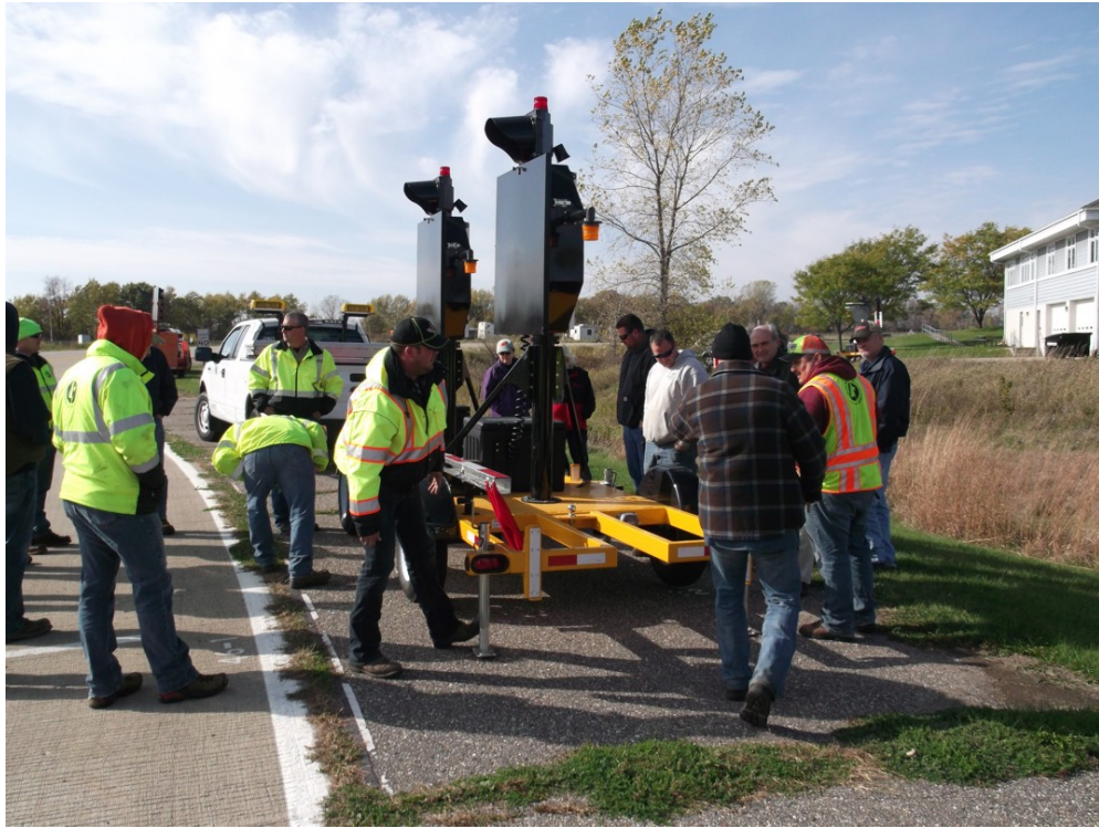
Figure 4.6 AF-76 Being Setup at Test Site
