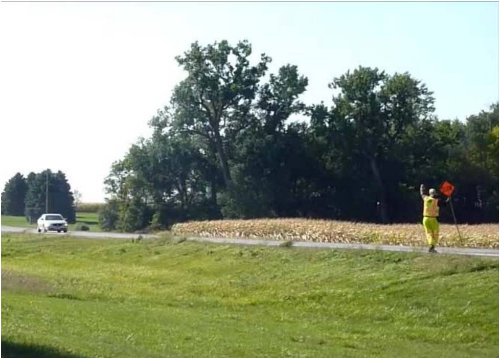
Figure 5.7 Vehicle Approaching Flagger
