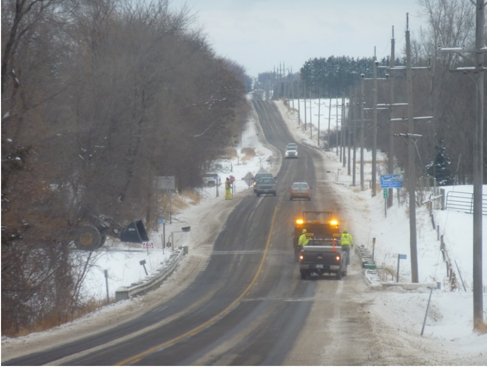
Figure 5.4 View of Work Zone
