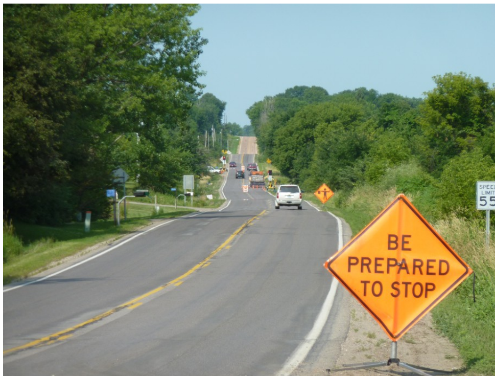
Figure 5.15 View of Work Zone
