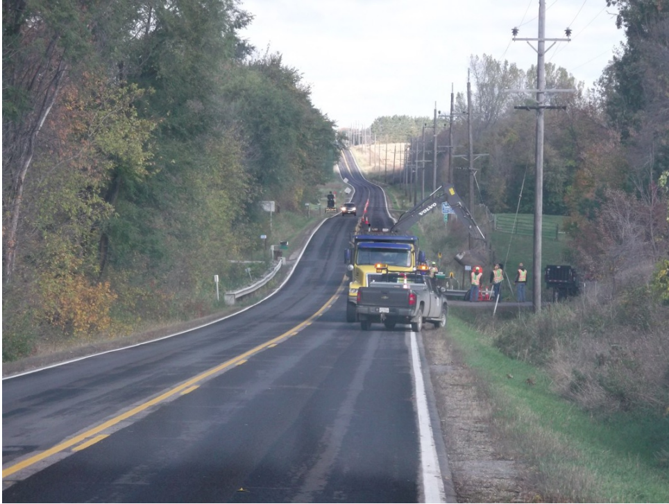
Figure 5.13 View From Operator Location Inside Truck
