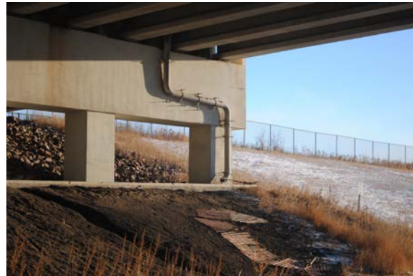
b) Down chute piping, outside lane.
