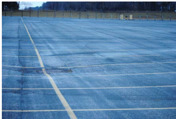
a) Drainage structure at Canterbury Park
