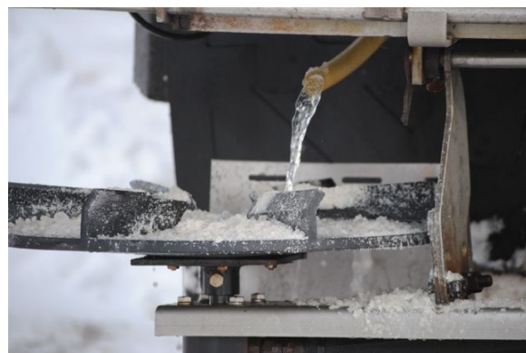
d) Prewet flow onto salt distributor (not in motion/not being fed deicer at time of photo).
