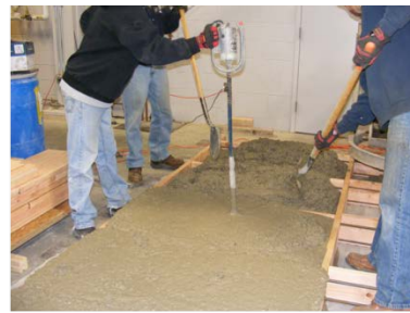
(b) Concrete vibration
