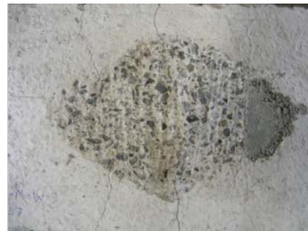
(b) Slab after testing
