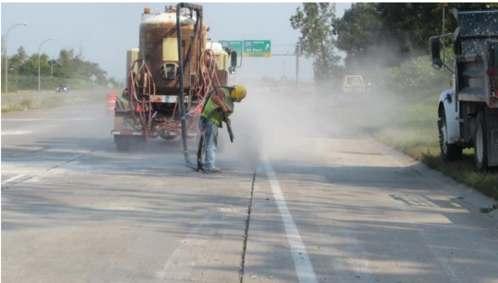
Figure 82: Sandblasting the patch area prior to being filled
