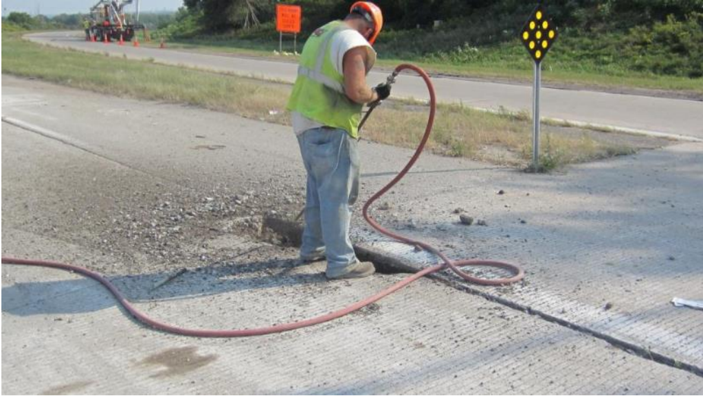
Figure 81: Air blasting the hole to remove excess loose material
