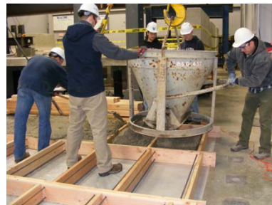
(a) Concrete placement
