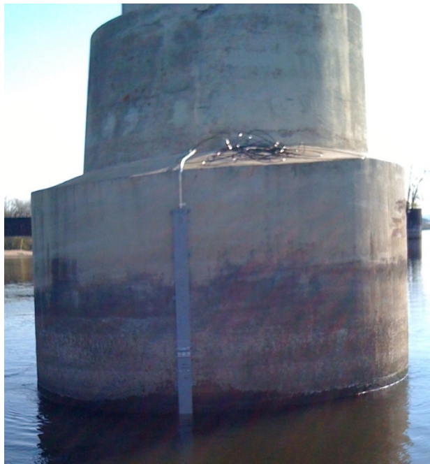
Figure 10: Bridge 5900 - Installed Sonar Mount
