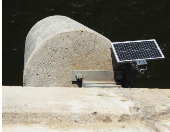
Figure 14: Bridge 07011 - Pier 4 Solar Panel from Deck
