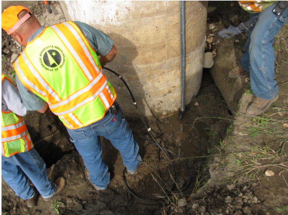
Figure 13: Bridge 07011 - Installation of Tethered Buried Switches
