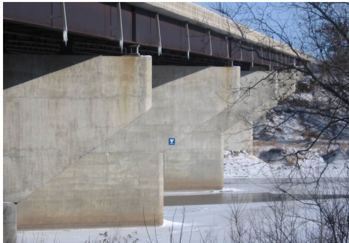
Figure 1: Bridge 07011 - Upstream profiles of piers 3 through 6
