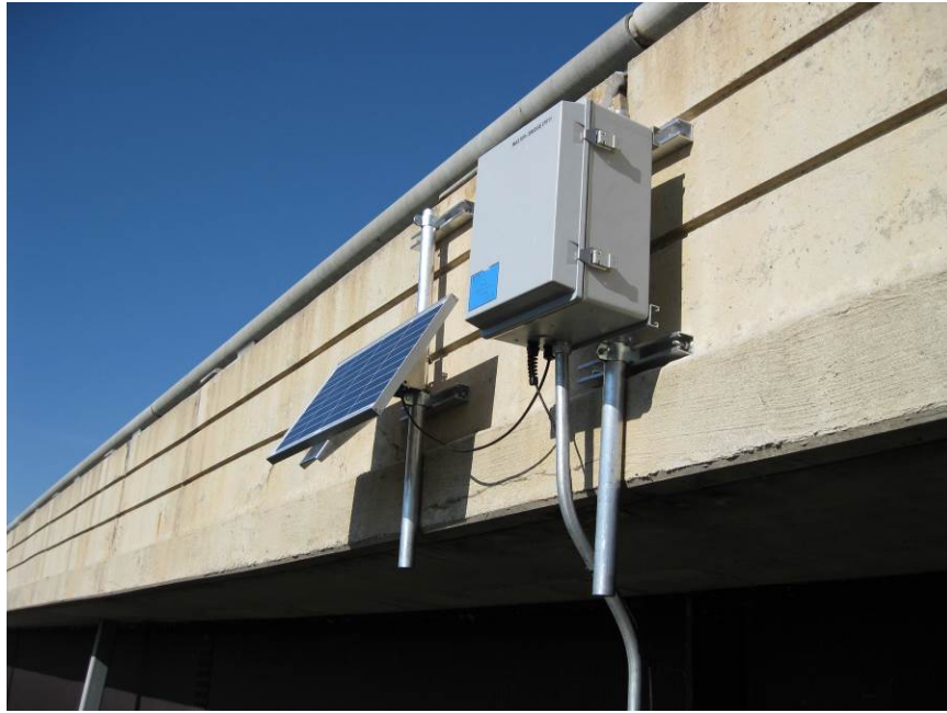
Figure 21: Bridge 07011 – Pier 5 Datalogger and Solar Panel
