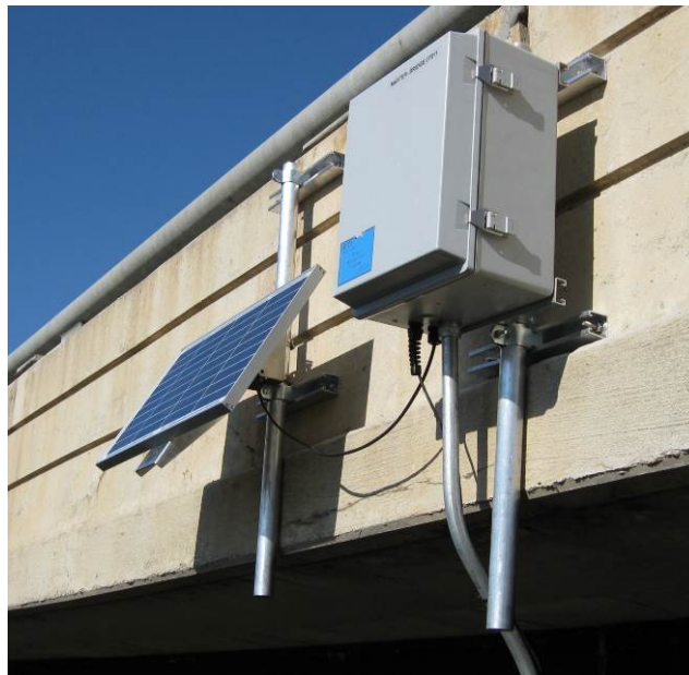
Figure 15: Bridge 07011 - Pier 5 Solar Panel
