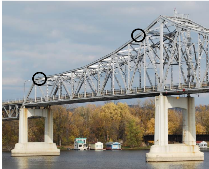
Figure 16: Bridge 5900 - Solar Panel Locations
