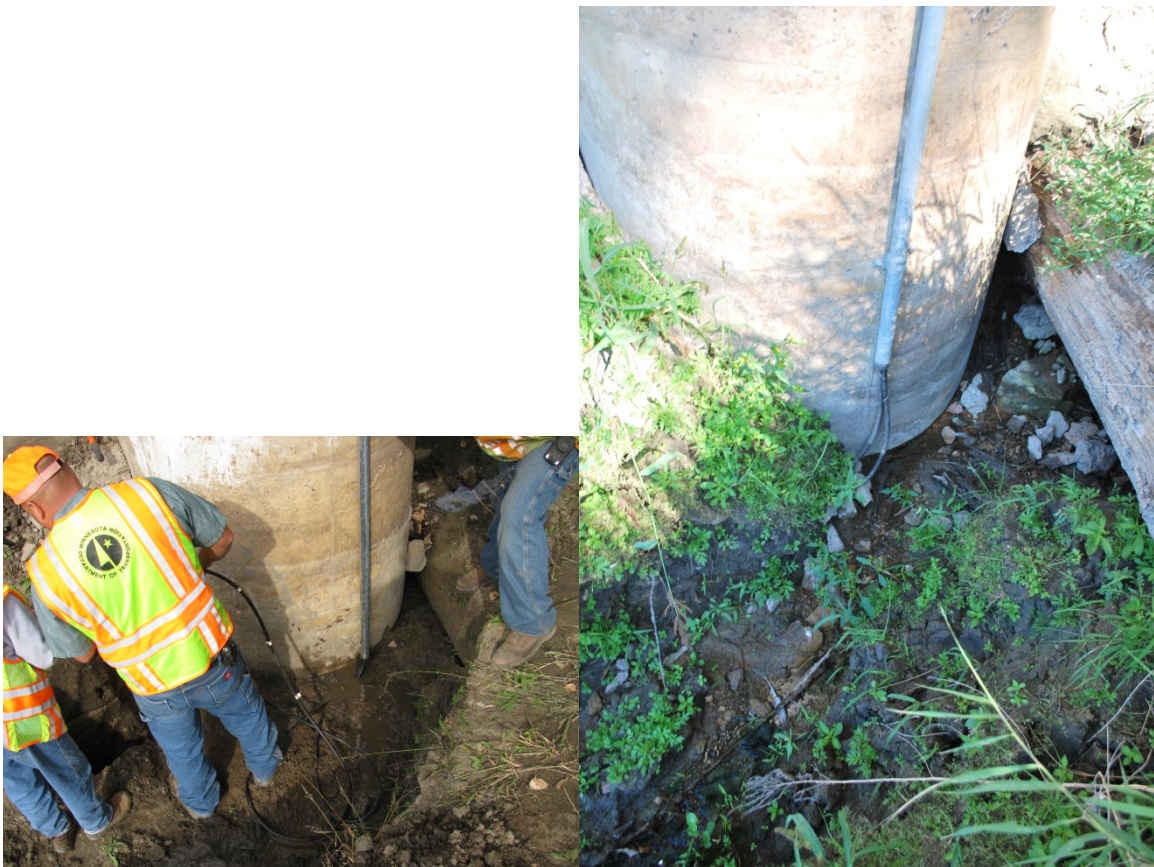
Figure 24: Pier 5 at Installation (10/25/2011) and Testing Event (9/12/2013)
