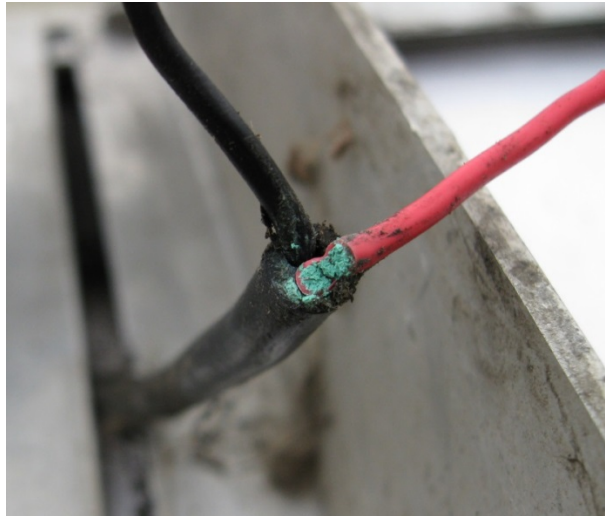
Figure 55: Wire Corrosion on Solar Panel Wire
