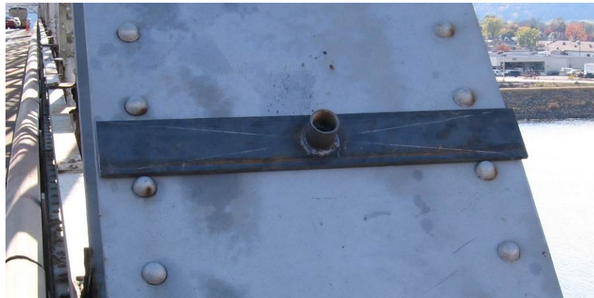
Figure 17: Bridge 5900 - Solar Panel Bracket
