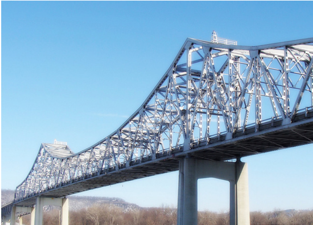
Figure 2: Bridge 5900 - Piers 18, 19, and 20 from Right to Left
