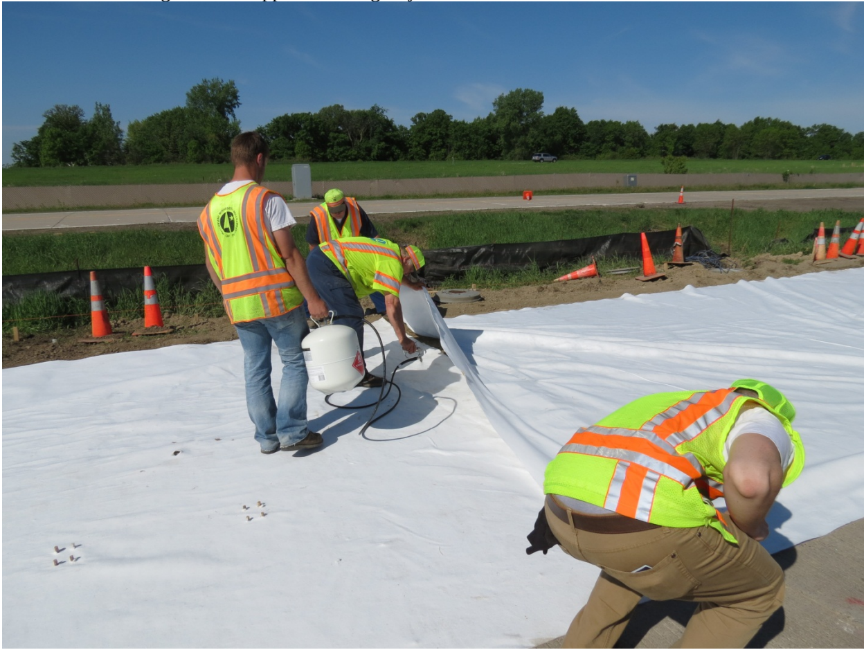
Figure 3.1 – Application of geosynthetic adhesive in cells 140 and 240.
