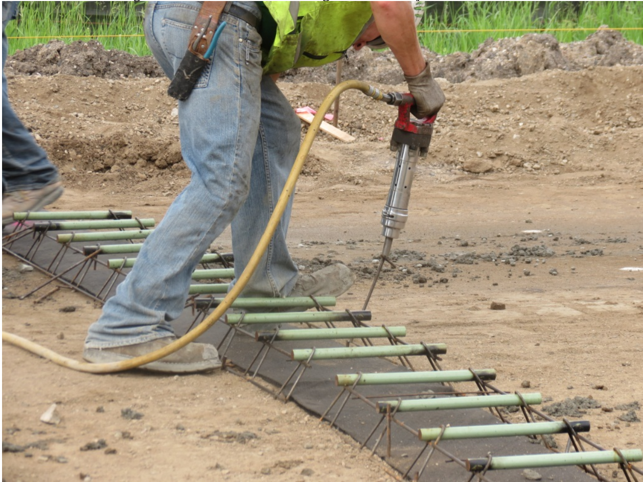
Figure 4.1 – Installation of drainage fabric under joints in cell 613.
