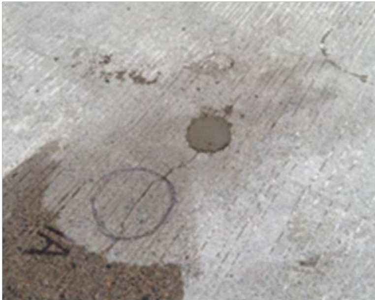
Figure 10. Final Patched Bridge Deck and Original Test Location.
