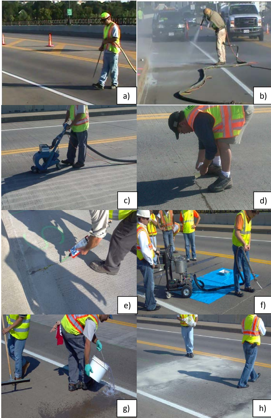
Figure 5. Typical Operations During Application. a) blowing surface with air b) sand blasting c) shot blasting d) bottle application e) caulk gun application f) pump application g) flood application h) sand casting on surface.
