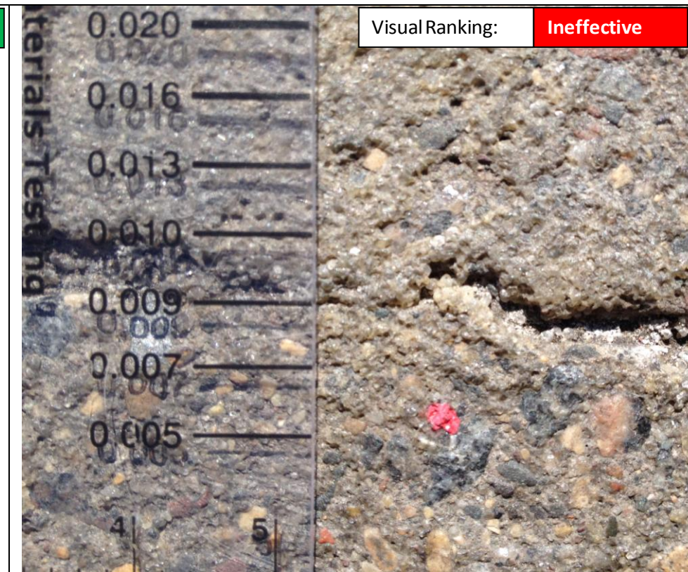
Photograph #: 57 Test Information: Test Section 10, Test 22A - Sika Corp Sikadur 55 SLV (Epoxy) Surface Prep & Application: Air, Route, Pump (squeegee), Sand: Yes Date: April 8, 2014 Project BL-09-03973 BRAUN INTERTEC
