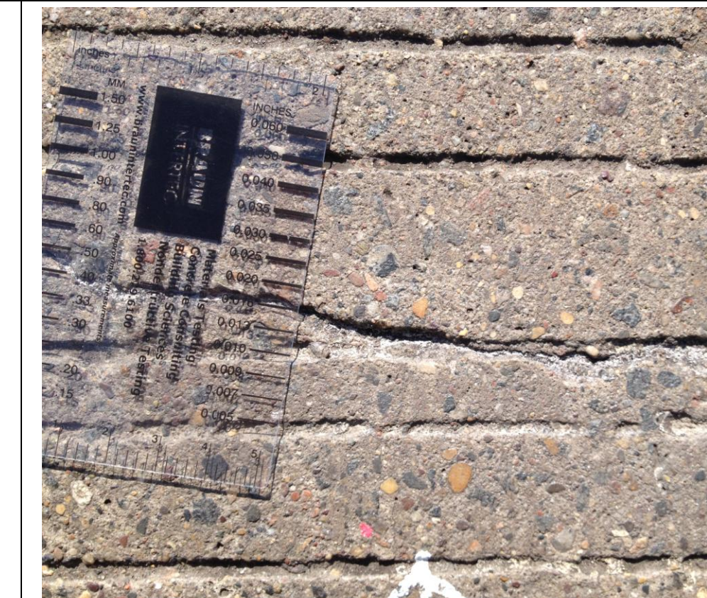
Photograph #: 9 Test Information: Test Section 2, Test 3A - CONTROL Surface Prep & Application: CONTROL Date: April 8, 2014 Project BL-09-03973 BRAUN INTERTEC
