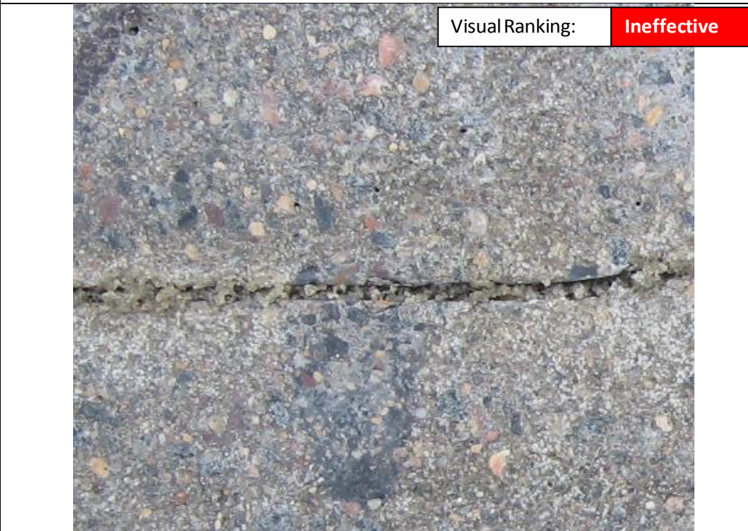
Photograph #: 59 Test Information: Test Section 10, Test 23A - Sika Corp Sikadur 55 SLV (Epoxy) Surface Prep & Application: Air Hose, Route, Pump (squeegee), Sand Coat: Yes Date: April 30, 2013 Project BL-09-03973 BRAUN INTERTEC
