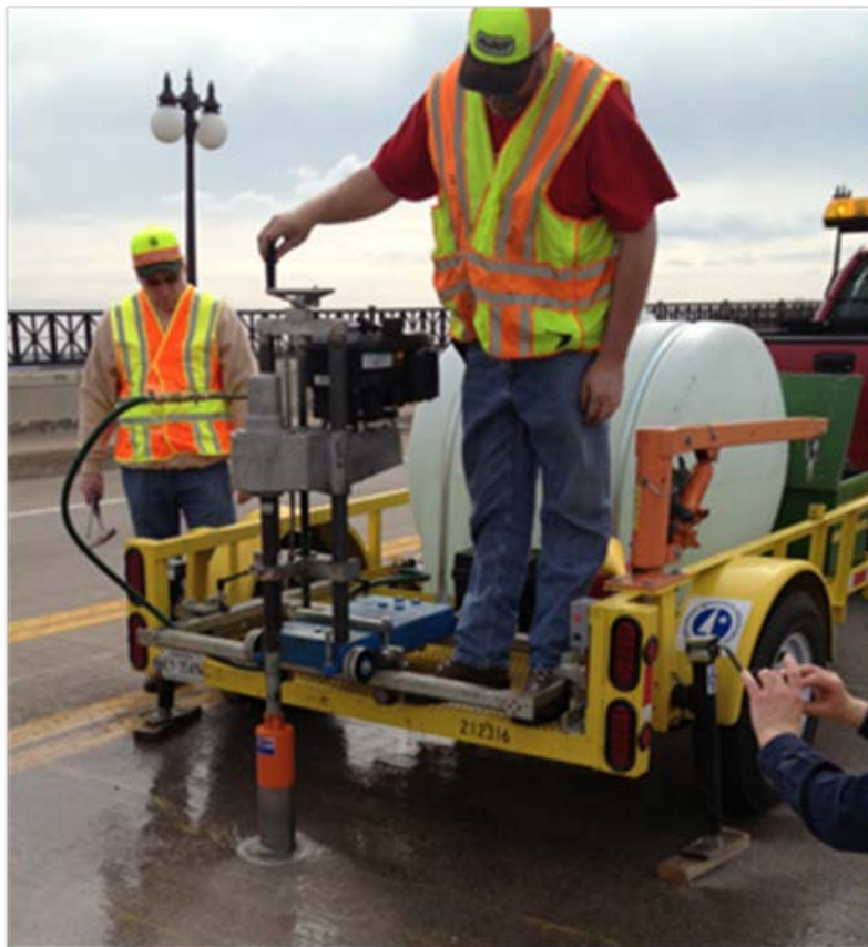
Figure 8. Coring on the Smith Avenue High Bridge.
