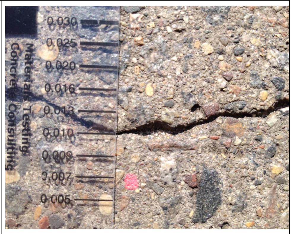
Photograph #: 36 Test Information: Test Section 6, Test 15A - CONTROL Surface Prep & Application: CONTROL Date: April 8, 2014 Project BL-09-03973 BRAUN INTERTEC
