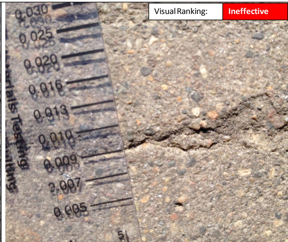
Photograph #: 39 Test Information: Test Section 7, Test 17A - BASF Epoxeal GS Structural (Epoxy) Surface Prep & Application: Air Hose, Flood (cracks), Sand Coat: Yes Date: April 8, 2014 Project BL-09-03973 BRAUN INTERTEC
