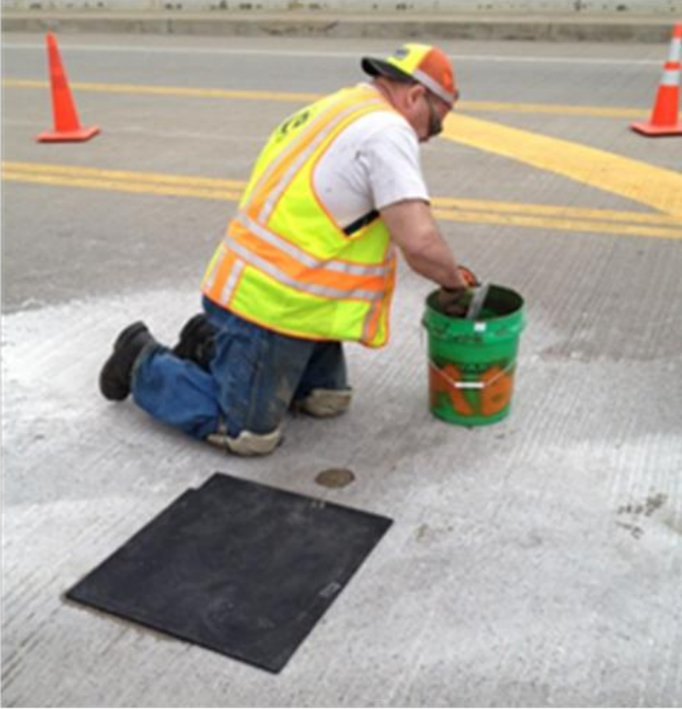
Figure 9. Patching Core Holes on the Smith Avenue High Bridge.
