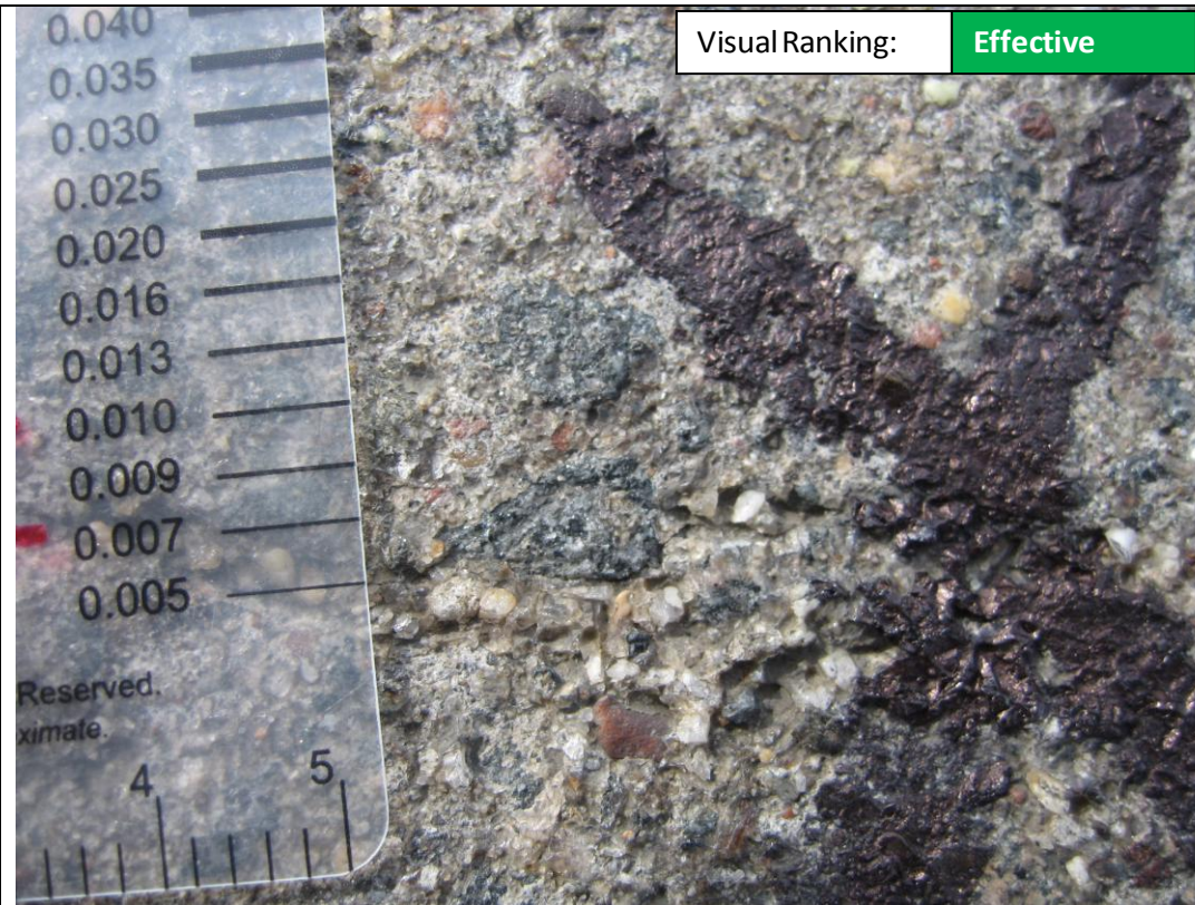
Photograph #: 43 Test Information: Test Section 8, Test 18A - Kwik Bond KBP 204 P (HMWM) Surface Prep & Application: Shot Blast, Flood, Sand Coat: Yes Date: May 11, 2012 Project BL-09-03973 BRAUN INTERTEC
