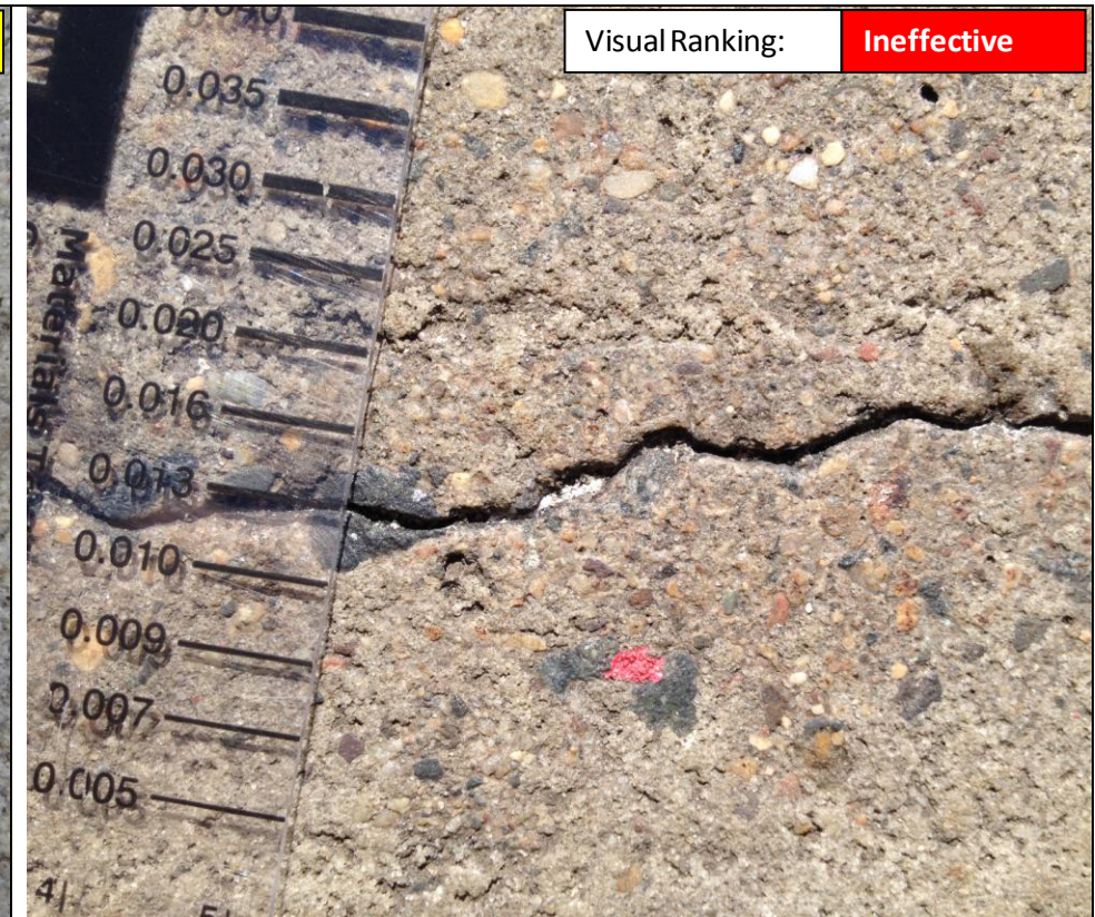
Photograph #: 75 Test Information: Test Section 13, Test 25A - Euclid Chemical Dural LM 50 (Epoxy) Surface Prep & Application: Air, Pretreat, Bottle (squeegee), Sand: Yes Date: April 8, 2014 Project BL-09-03973 BRAUN INTERTEC
