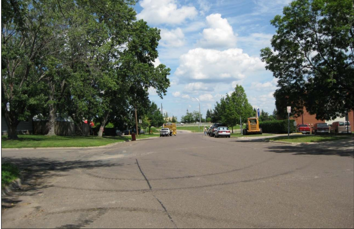
Figure 4.20: Example of 76 th Street Cross-Section Before Reconstruction Source: City of Richfield, Minnesota
