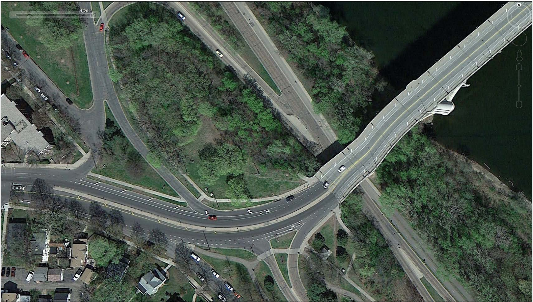
Figure 4.54: East Franklin Avenue Near Mississippi River Bridge After Reconstruction Showing Two Travel Lanes
