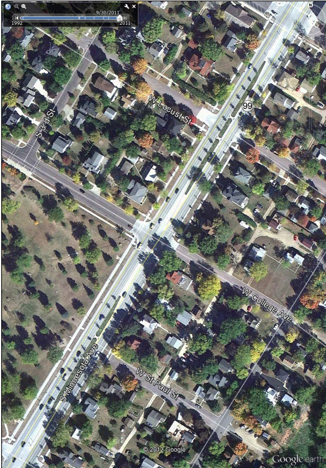
Figure 4.33: TH 169 Between West Elm Street and West Walnut Street After Reconstruction Showing Raised Median and Exclusive Left-Turn Lane Improvements
