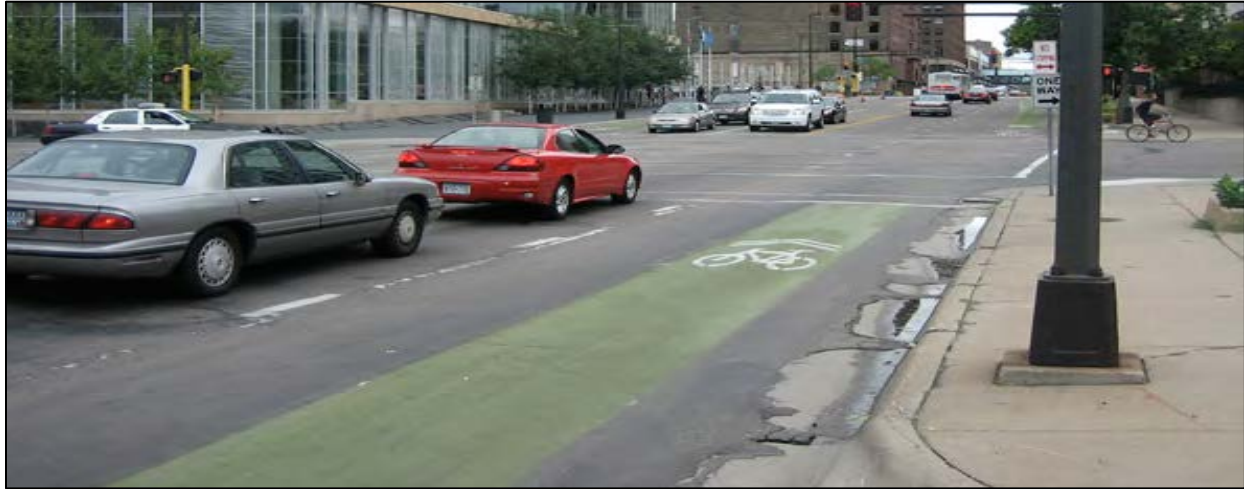
Figure 4.39: Example of Hennepin Avenue Bicycle Lane After Reconstruction
