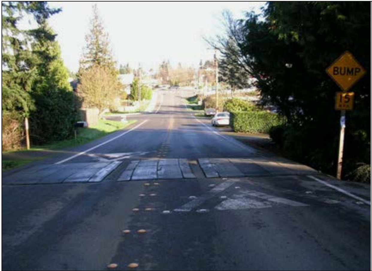
Figure 2.8: Speed Cushion in Seatac, Washington [20]
