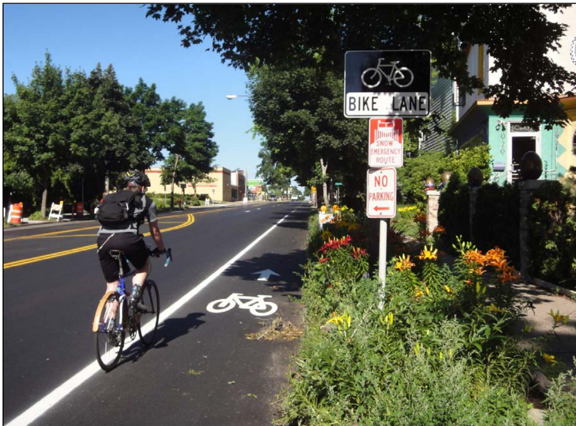
Figure 4.52: East End of Franklin Avenue After Reconstruction Showing Two Travel Lanes and Bicycle Lane
