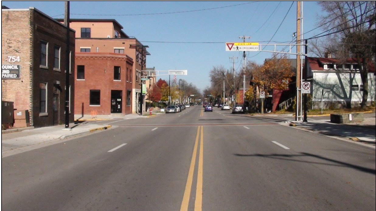
Figure 4.42: Williamson Street Cross-Section Following Reconstruct with Widened Terraces
