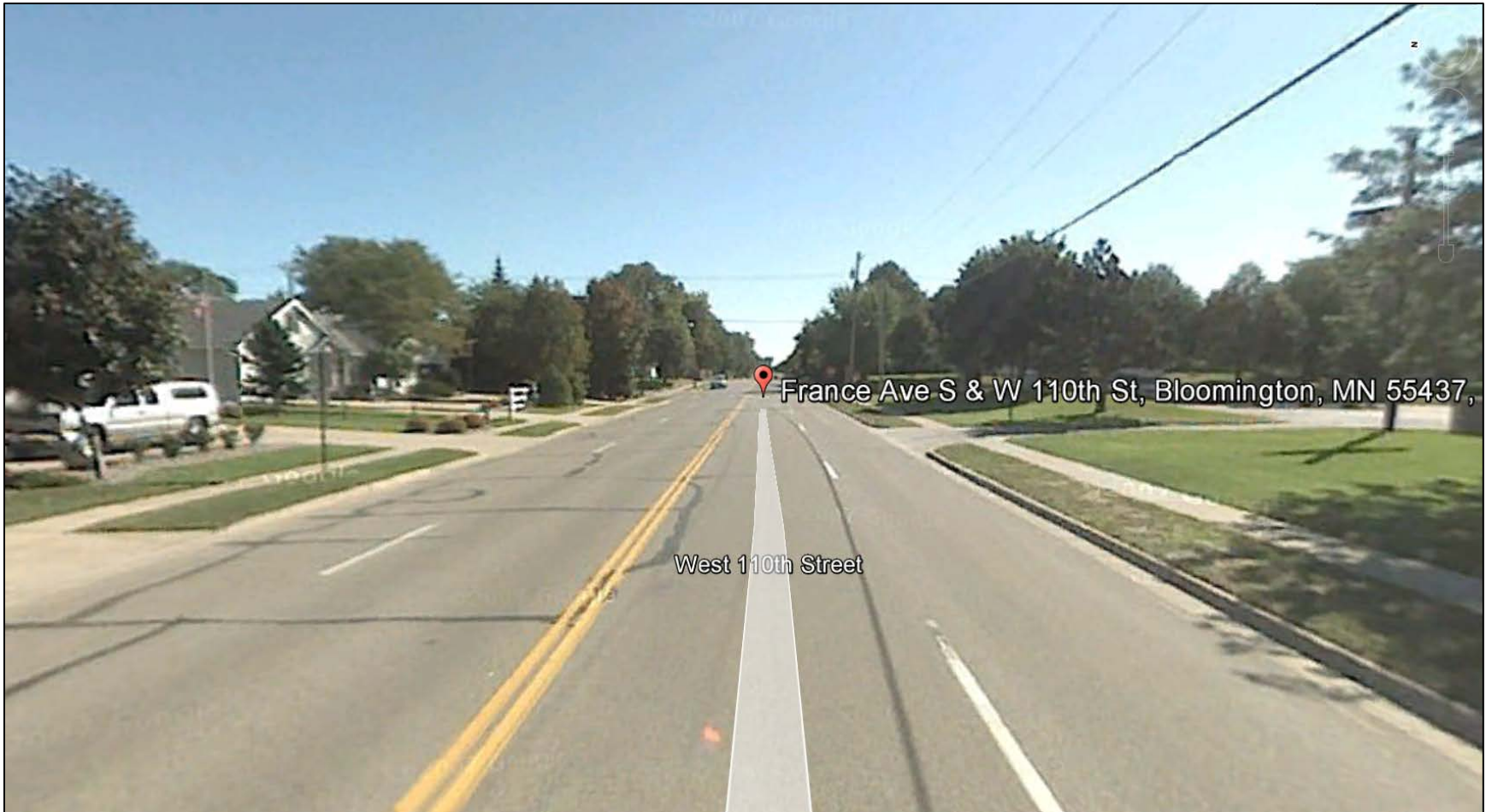
Figure 4.10: Example of West 110 th Street Section (Near France Avenue) Before Reconstruction Showing Four-Lane Roadway and Off-Peak Parking in Outside Lanes
