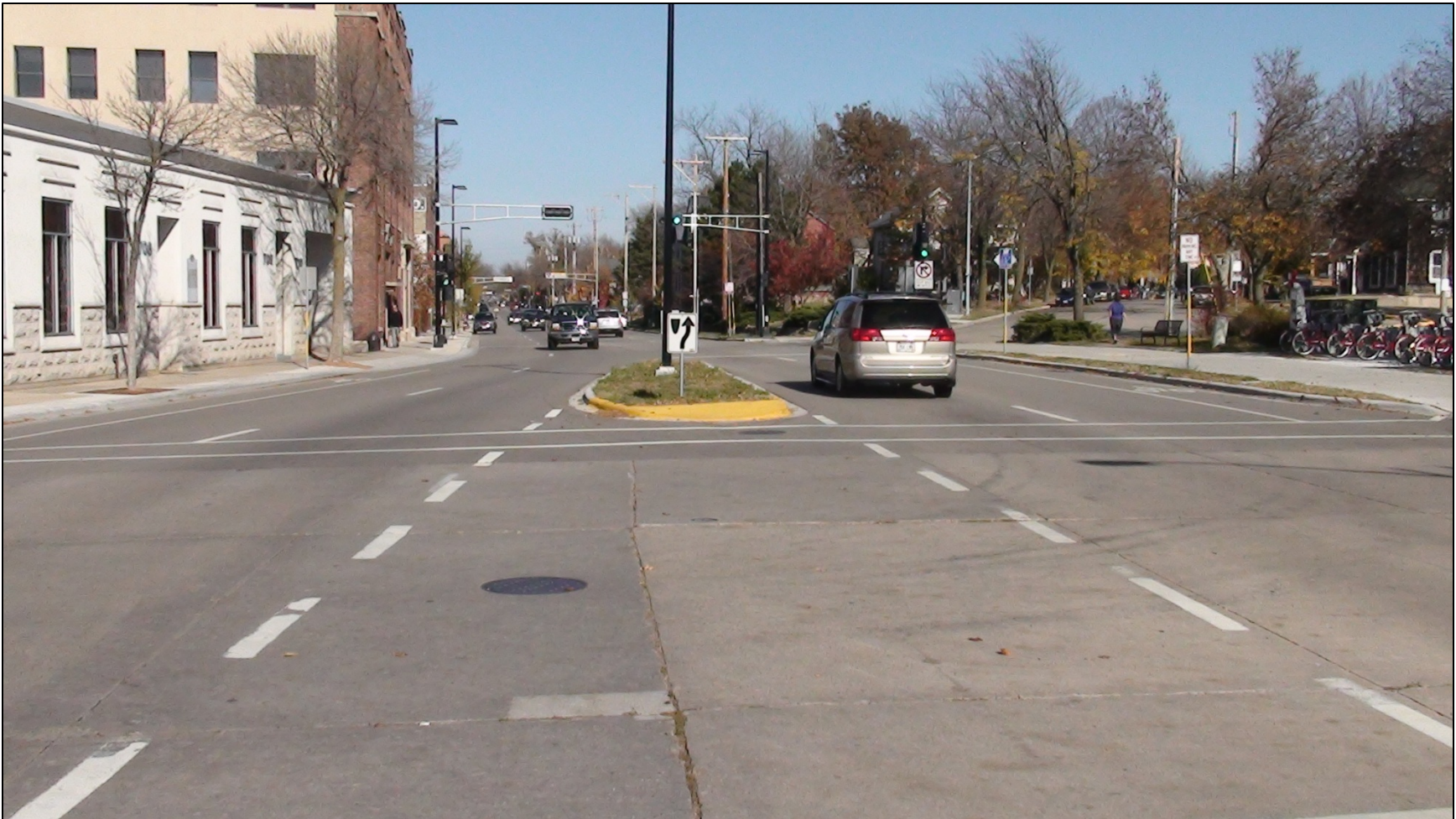
Figure 4.44: Intersection of Williamson Street and Blount Street After Reconstruction Showing Reduction in Lane Width and Addition of Bicycle Lanes
