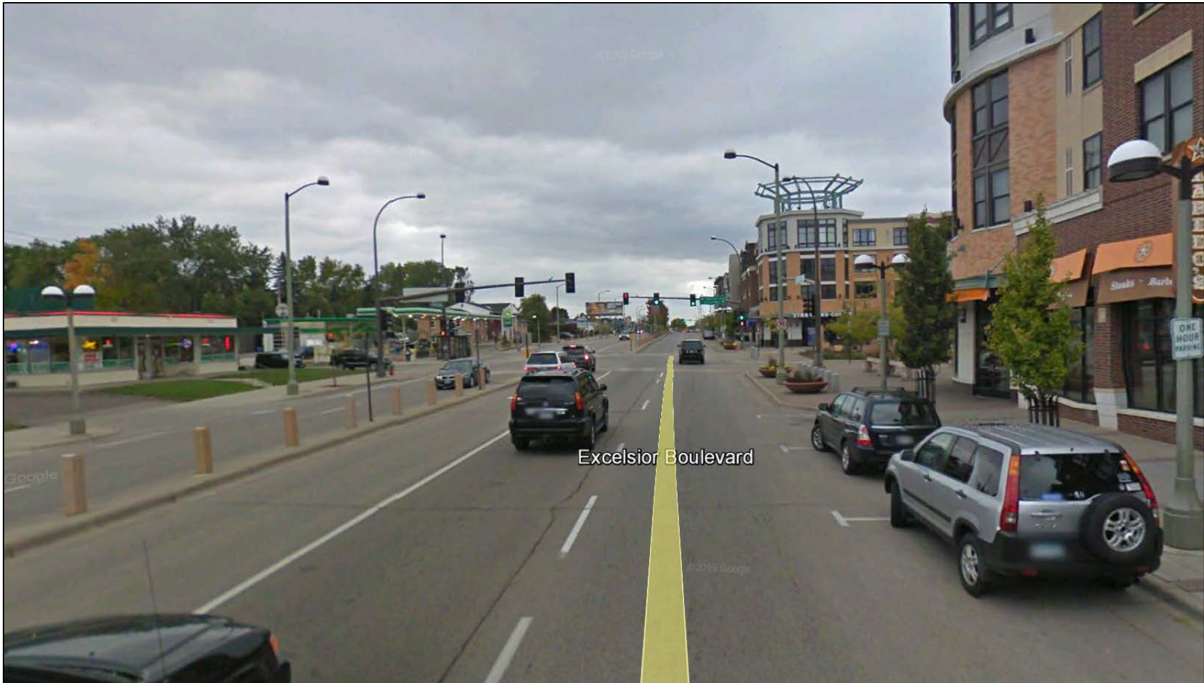
Figure 4.3: Excelsior Boulevard and Grand Way Intersection After Reconstruction
