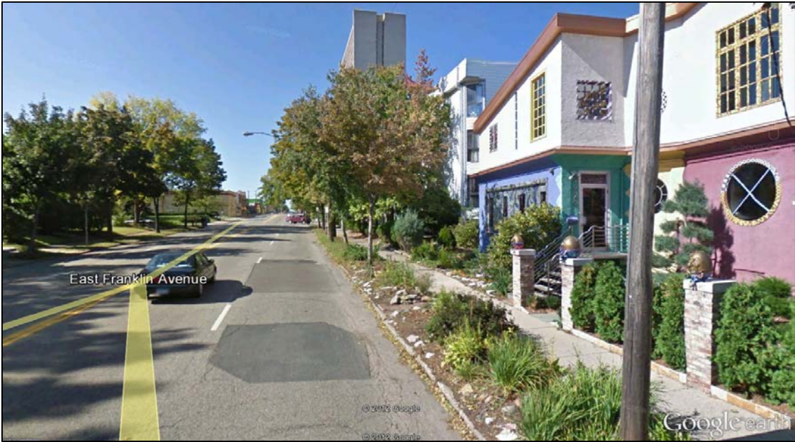
Figure 4.51: East End of Franklin Avenue Before Reconstruction Showing Four Travel Lanes
