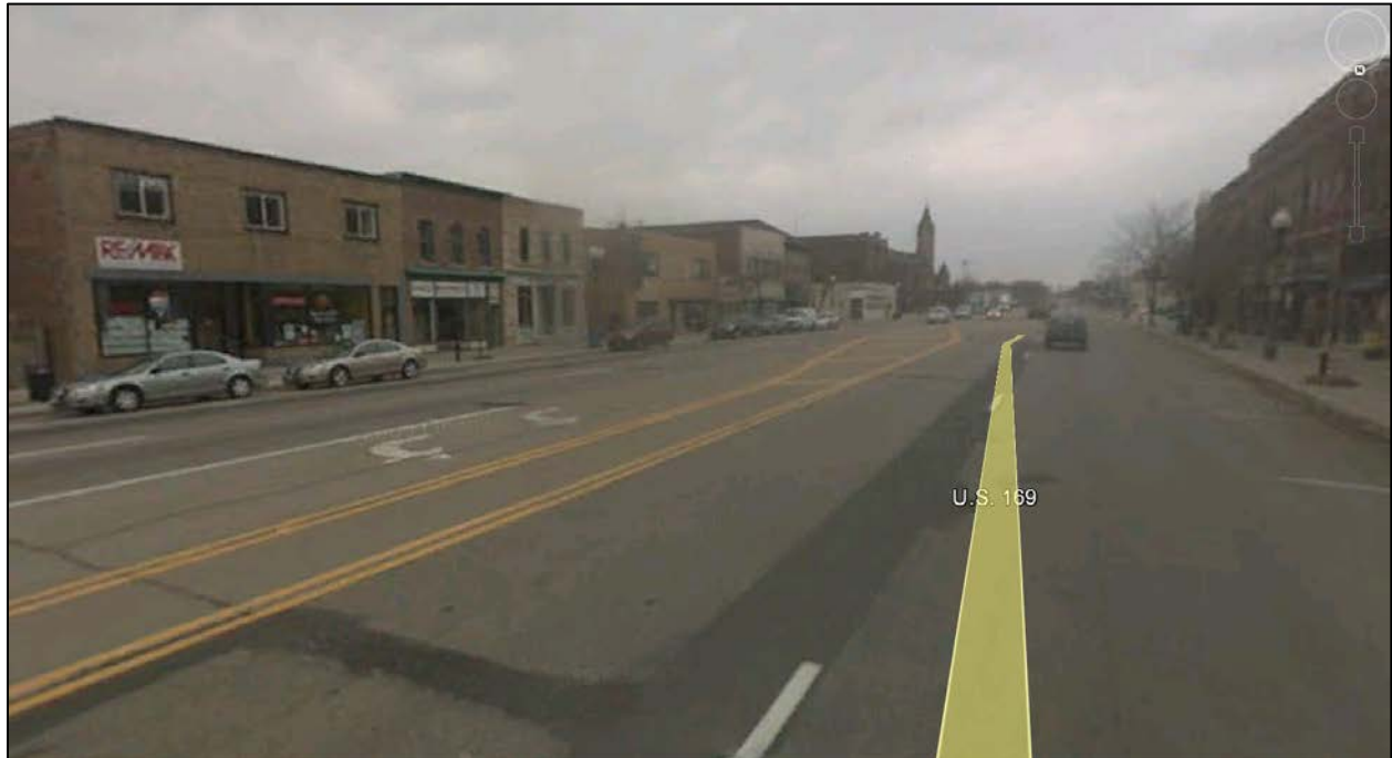
Figure 4.30: Example of Median Before Reconstruction on TH 169 (Near West Nassau Street Intersection)
