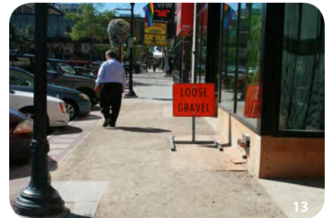
13. During maintenance along Broadway, efforts are made to keep the ground level so the sidewalk is still accessible.
