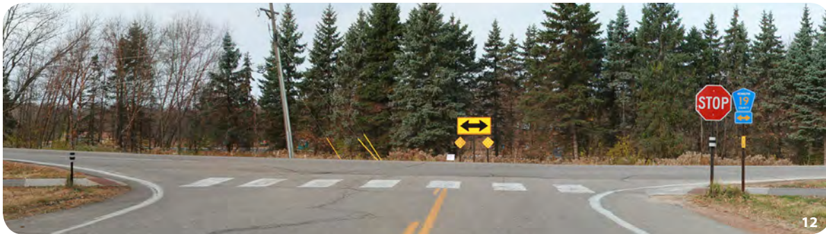
10-12. CSAH 19 near Loretto includes a multiuse trail along the east side of the highway. This trail features visible crossings at key intersections and separates bikes and pedestrians from the vehicle travel lanes where the speed limit is 55 miles per hour.
