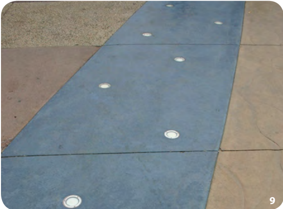
9. Integrated lighting provides additional pedestrian scale lighting and becomes a design element that runs throughout the plaza across 1st Avenue where the plaza continues.
