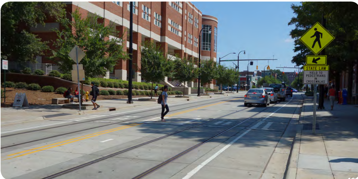
18. Elizabeth Avenue, which runs through Central Piedmont Community College, was recently rebuilt with track laid for a planned streetcar line. The streetcar project will be completed in 2014, but the installation of track was coordinated with recent road construction. The roadway accommodates a large amount of vehicle, bicycle, and pedestrian traffic. Mid-block crossings and signage and bike lanes facilitate non-motorized travel.
