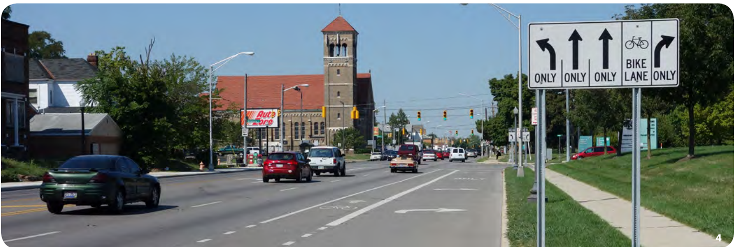
3. Bike lanes and signage on West Broad Street near the Ohio Department of Transportation illustrate complete streets on a wide arterial street.
