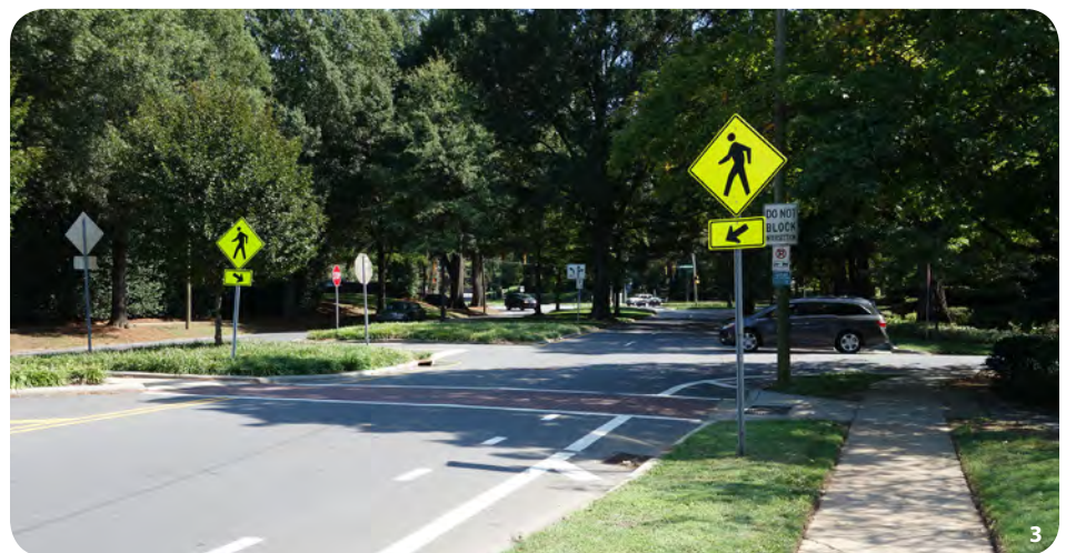
3. East Boulevard mid-block crossing near Freedom Park and intersection with Queens Drive and Kings Drive. Roadway features medians, landscaping, and a bike lane.
