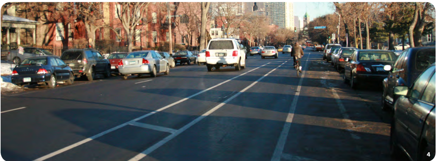
4. Park and Portland Avenues in Minneapolis feature new buffered bike lanes. Buffers are incorporated on both sides of the bike lane putting cyclists in a safer zone from moving cars, or opening car doors. The buffers are indicated by pavement striping and signage at intersections.
