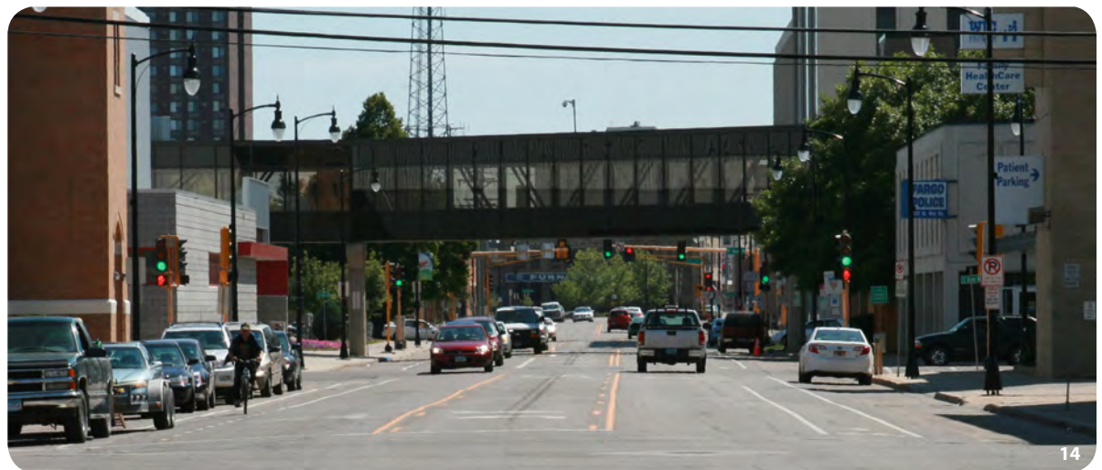
14. In a more urban section of 4th Street North, travel lanes are clearly marked and bicycles are separated from the vehicle travel lanes.
