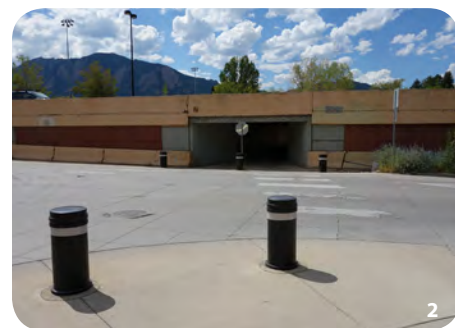
1-2. 28th Street Frontage Road includes sharrows, wide sidewalks with landscape buffers, crosswalks, and a tunnel under the Denver-Boulder Turnpike connecting hotels and apartments to the University of Colorado Boulder.
