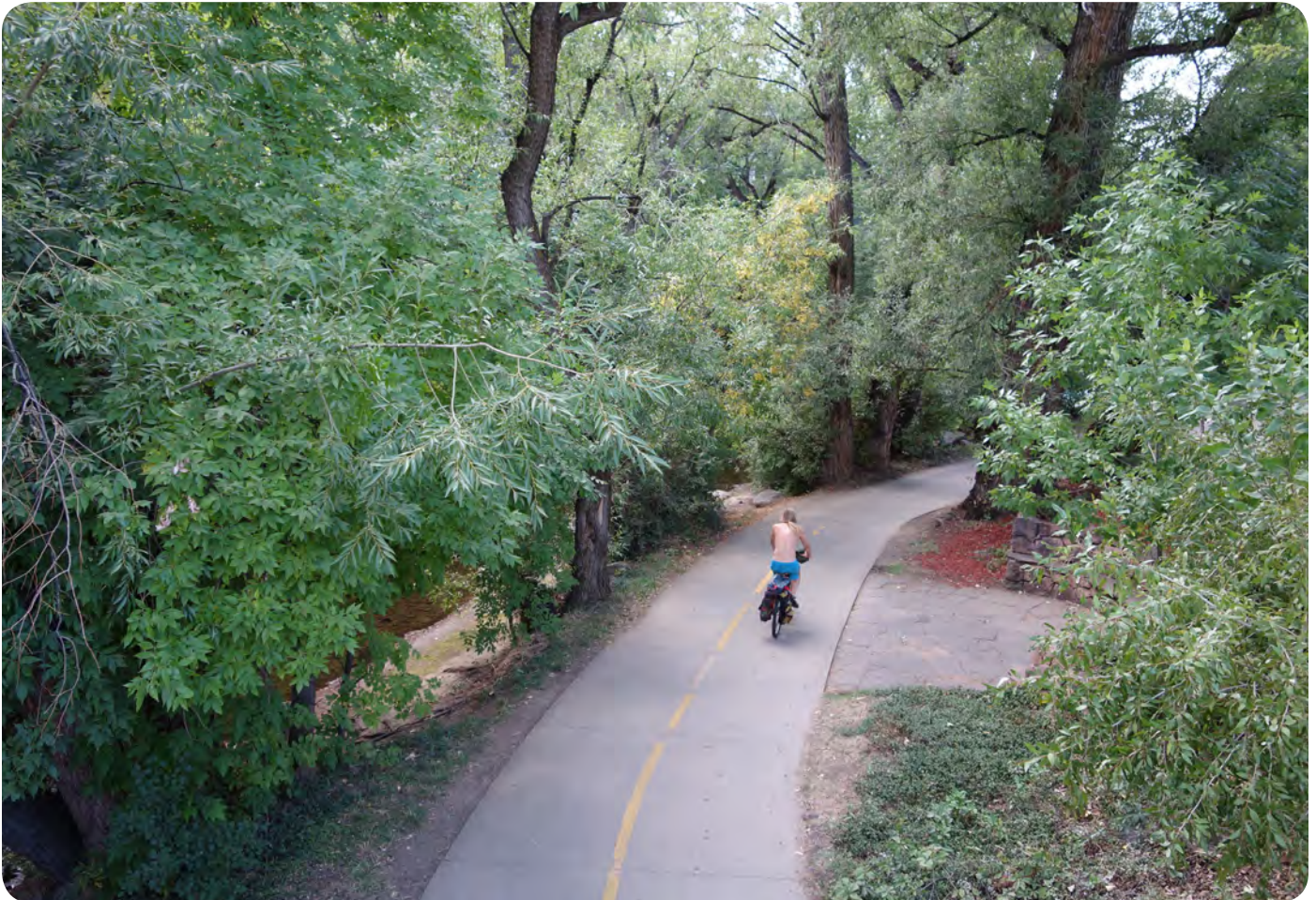
The Boulder Creek Multi-Use Path was constructed as part of a larger flood control project, in coordination with Boulder’s Flood Control Utility. It provides a critical east-west connection through the city.
