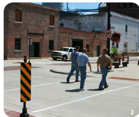
2. Bump outs and caution signage make it safer for pedestrians to cross 10th Street.
