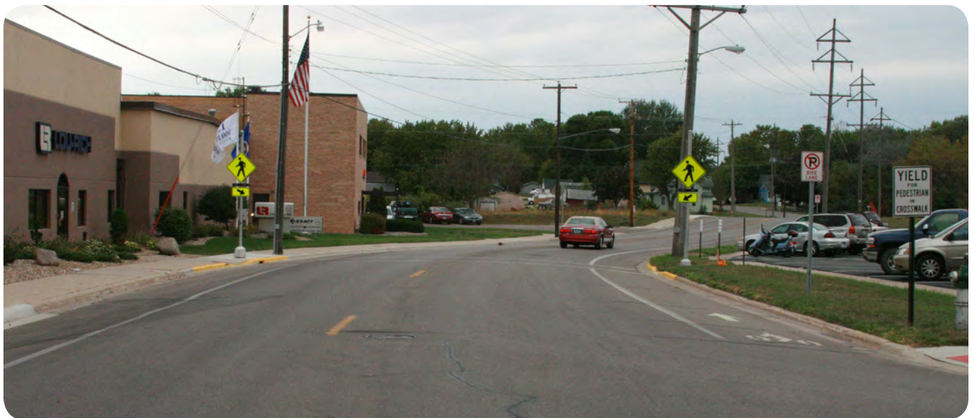
A highly visible pedestrian crossing connects employment centers to a surface parking lot along Albert Lea's Front Street. The crossing sign lights when activated by a pedestrian.
