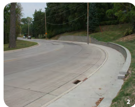
2. Widened sidewalk and improved retaining wall along Lakeview Boulevard.
