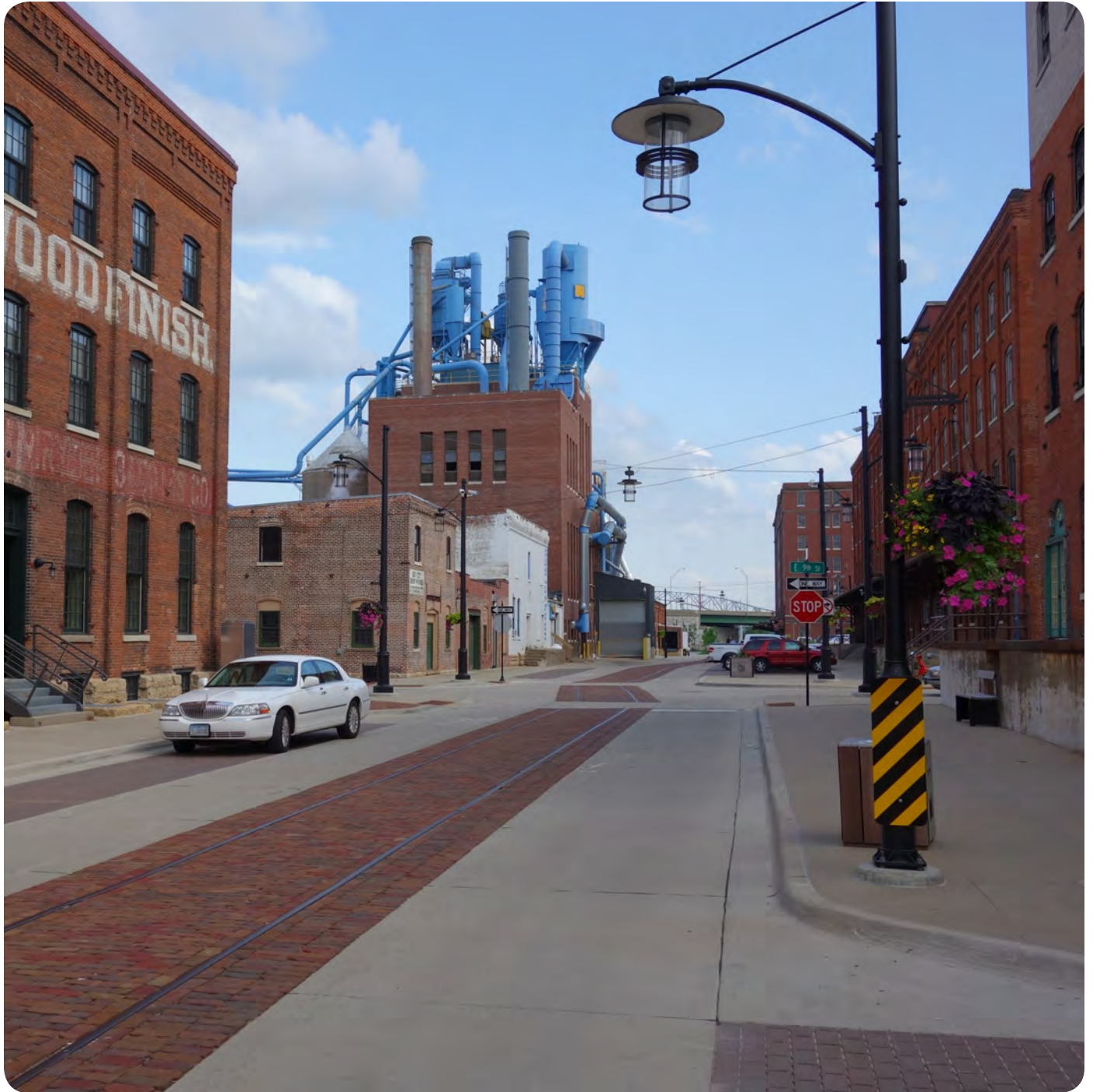
The 12-block Historic Millwork District in Dubuque incorporates complete streets features.
