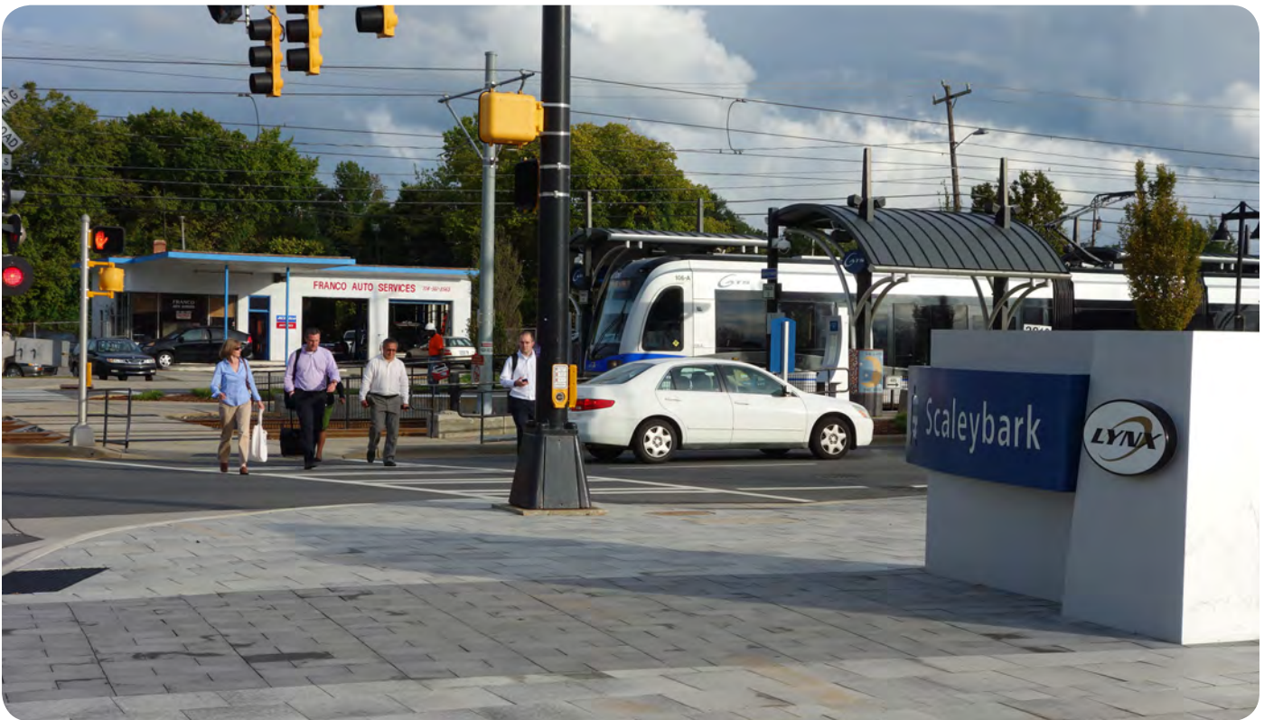
The Scaleybark station on the LYNX line in Charlotte includes design features that facilitate safe access from the train platform to the adjacent park and ride facility.
