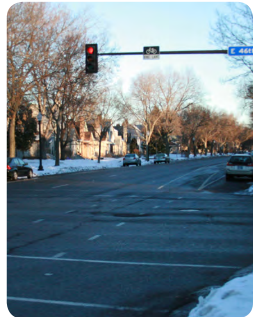
An example of how the bike lane is striped through a busy intersection.
