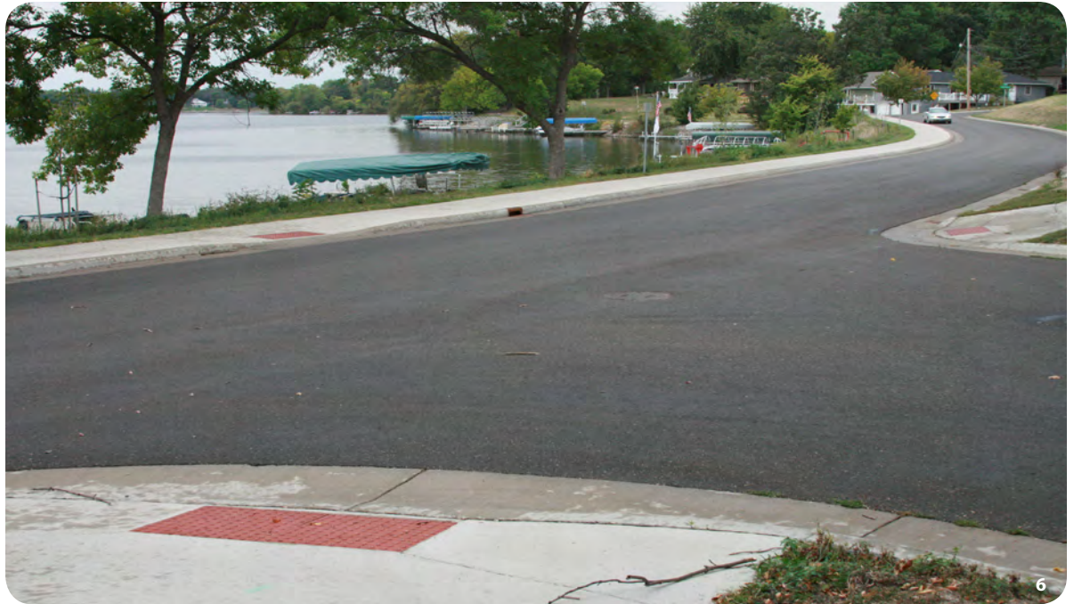
6. An improved intersection along West Lakeshore Avenue with wider curb cuts, ADA compliant ramps, and a sidewalk that allows residents to walk along the lake shore. The sidewalk connects to the Fountain Lake Trail an important multi-use trail that allows pedestrians and cyclist to remain along the lake shore instead of navigating city streets and provides access to Brookside Park.
