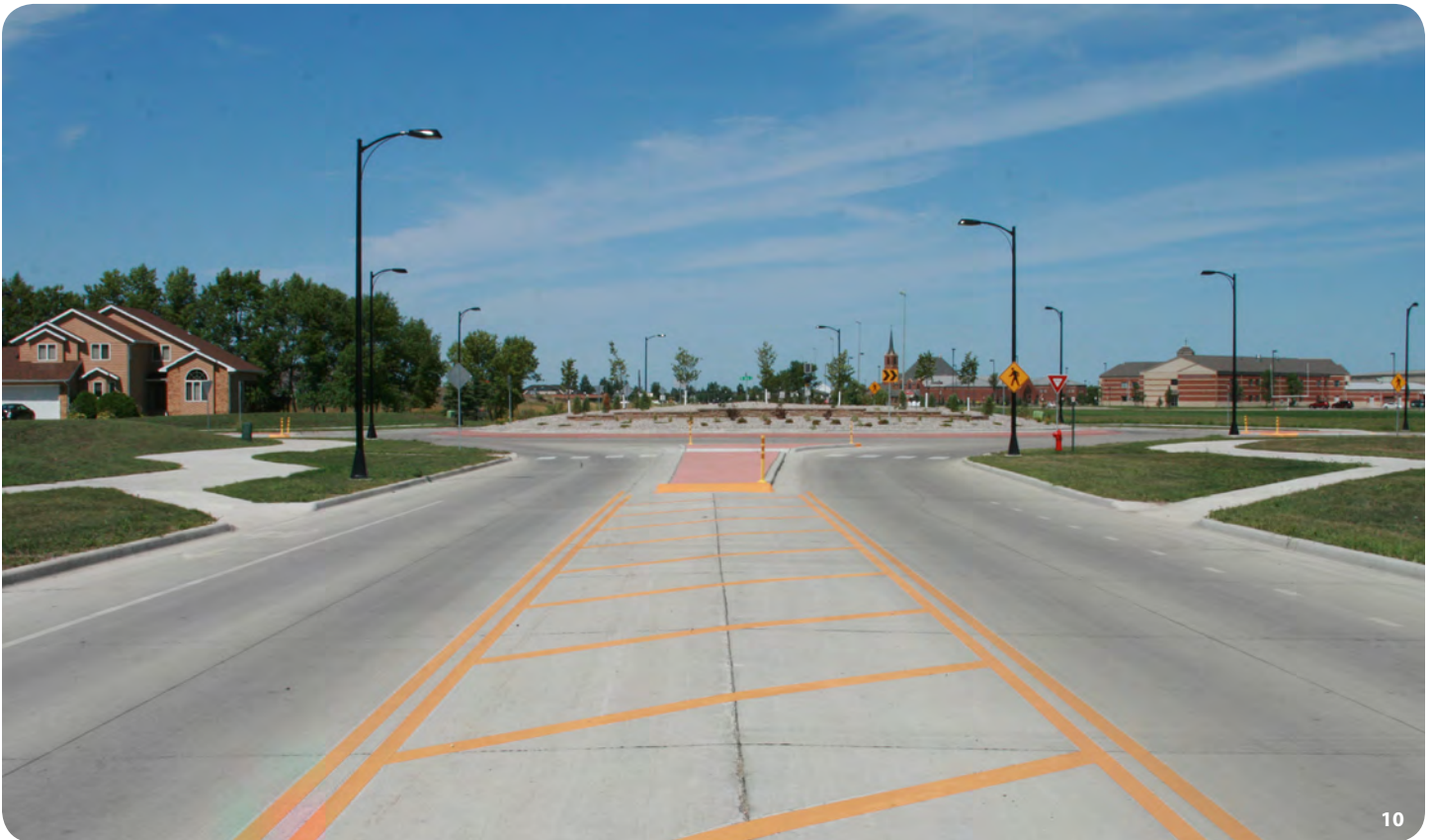
10. The City of Fargo Engineering Department has experimented with various roundabout configurations and developed a design standard that works well for safety and winter maintenance. This roundabout features a large center island with a flat surface, or apron. This configuration is easier to plow in the winter months and allows large emergency vehicles to surmount the center island curb if necessary.
