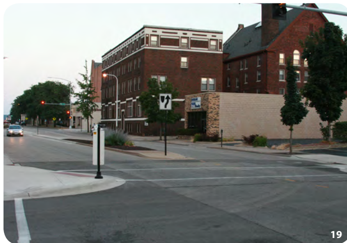
19. New bump outs, ADA compliant ramps, and median along Iowa Street.
