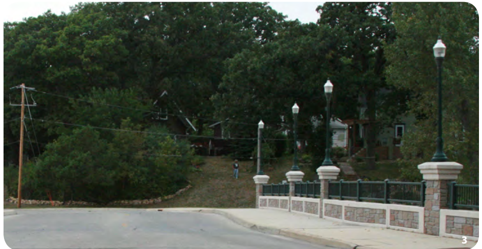
3. New wide sidewalks, period lighting, ADA compliant ramps, and unique concrete detailing on the Lakeview Boulevard bridge make it more pedestrian friendly.
