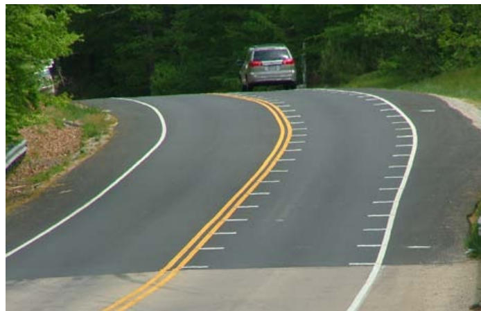
Figure 9. Optical speed bars (VDOT 2006)
