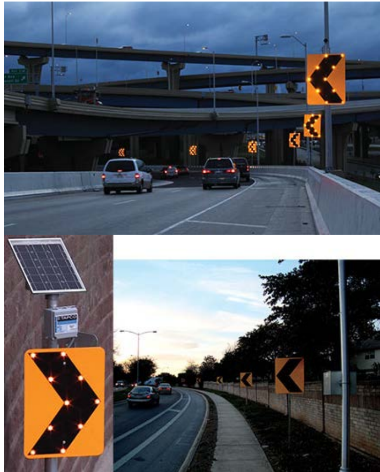
Figure 36. Sequential dynamic curve warning system (FHWA 2012)
