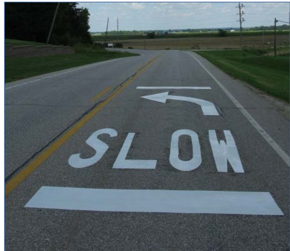
Figure 30. On-pavement curve sign
