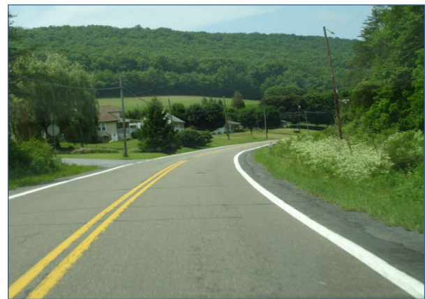
Figure 7. Before and after application of wider edge lines (Donnell et al. 2006)
