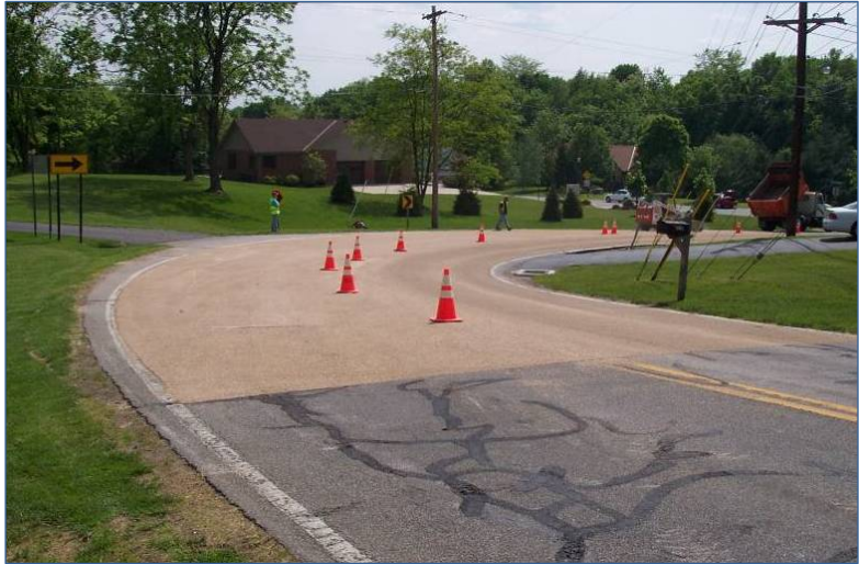
Figure 5. High-friction treatment (The Transtec Group, Inc., highfrictionroads.com )
