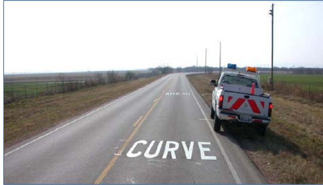
Figure 31. On-pavement curve markings (Chrysler and Schrock 2005)
