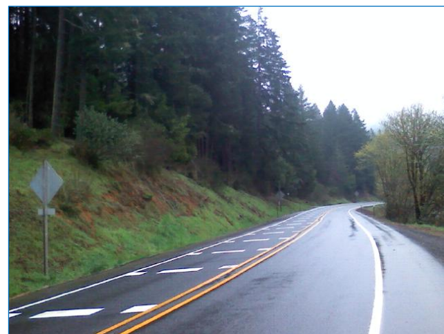
Figure 8. Various on-pavement curve markings
