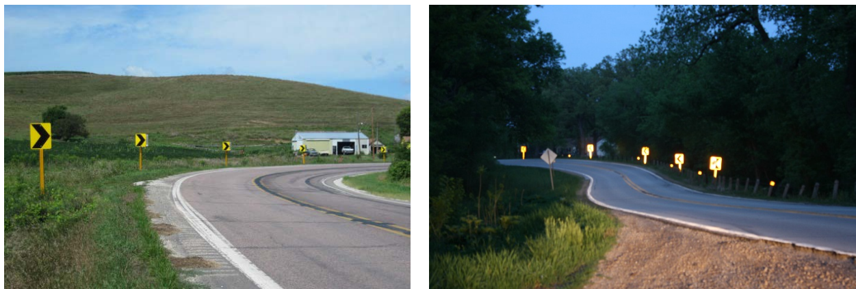
Figure 23. Reflective treatment added to existing chevron posts
