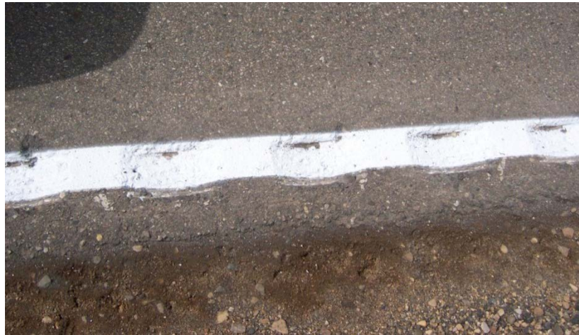
Figure 27. Edge-line rumble stripe on a rural Iowa highway (Hallmark et al. 2010)
