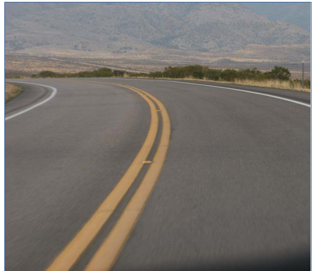
Figure 6. RPMs used in the center of a curve
