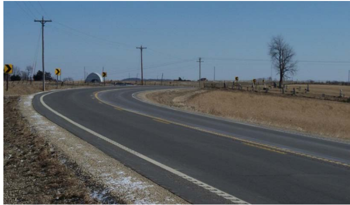
Figure 24. Edge-line and centerline rumble strips
