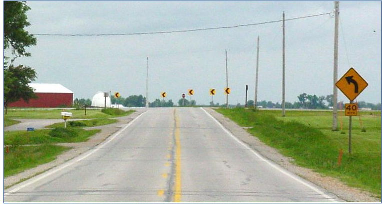
Figure 2. Oversized chevrons on US 6 in Johnson County, Iowa (Tom Welch, Iowa DOT)
