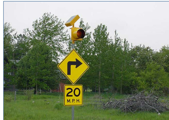
Figure 33. Flashing beacons (Bowman 2012)
