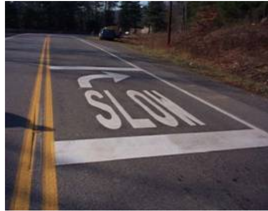
Figure 32. On-pavement treatment applied in Iowa
