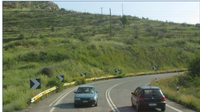
Figure 3. Panels of retroreflective sheeting to delineate curves
