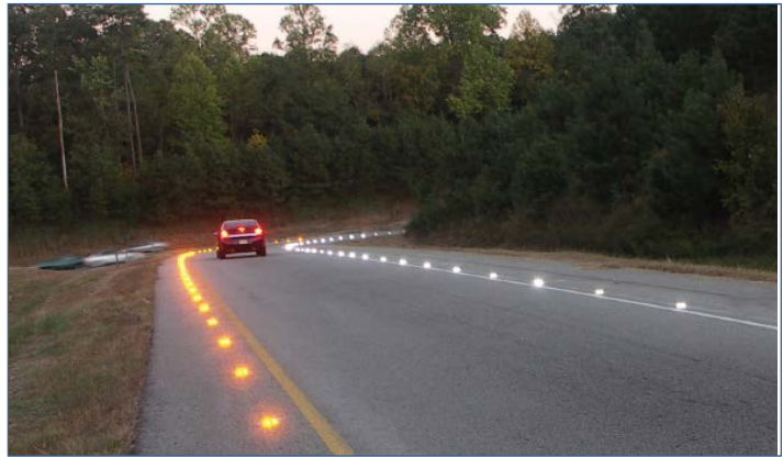
Figure 42. In-pavement lighting (FHWA 2011)
