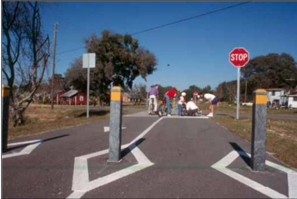
Figure 3.17: Bollards on Bike Trail [6]
