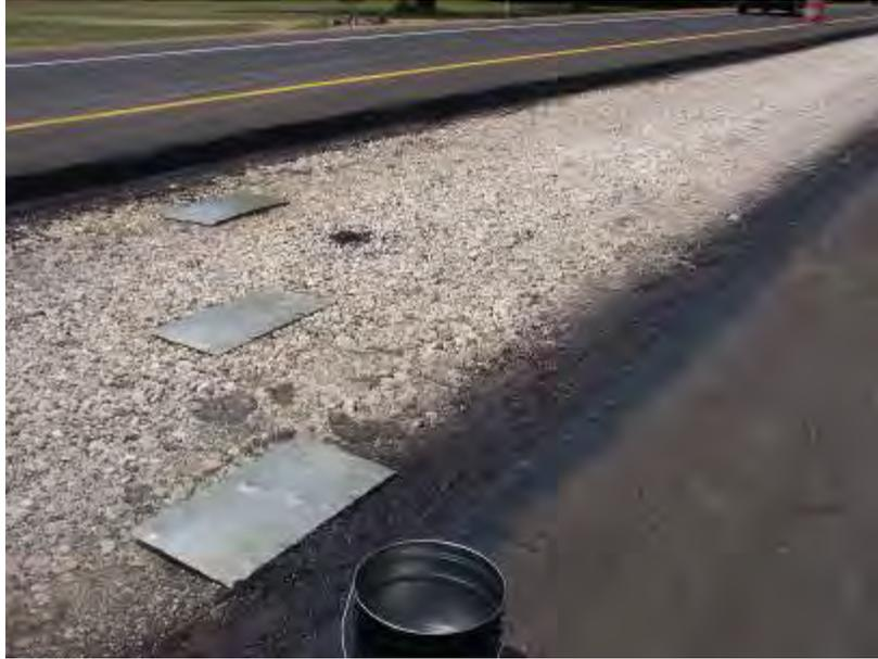
**Figure 5-19: Plates randomly placed under HMA mat.**
