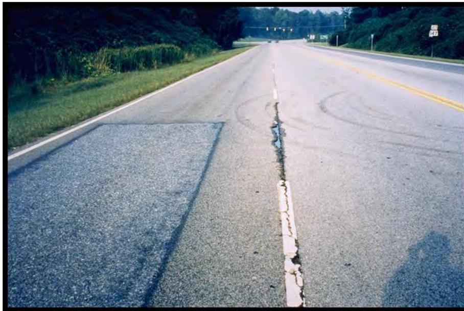
**Figure 5-11: Raveled longitudinal joint (Brown, 2006).**
