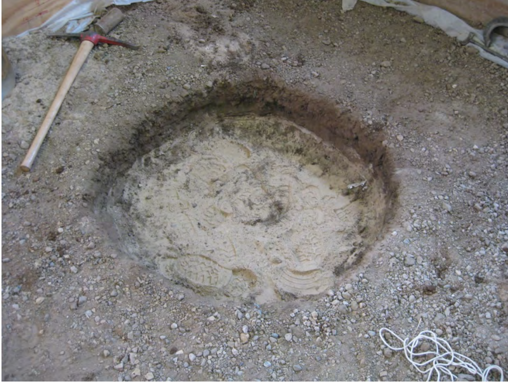
Figure A.1. Overview of Abbreviated Test Pit Area prior to Material Placement.
