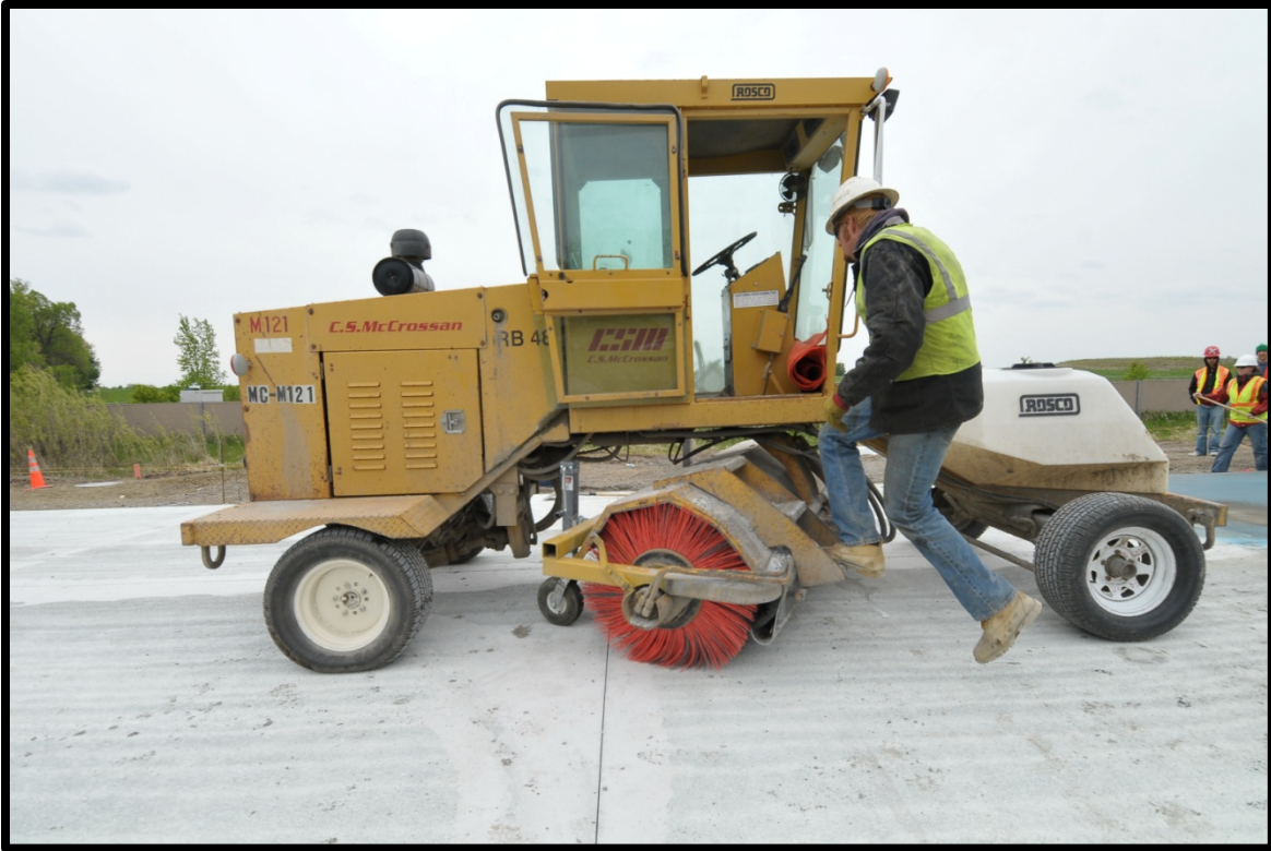
Figure 15: MnROAD Mainline Cell 72 Brushing (1)
