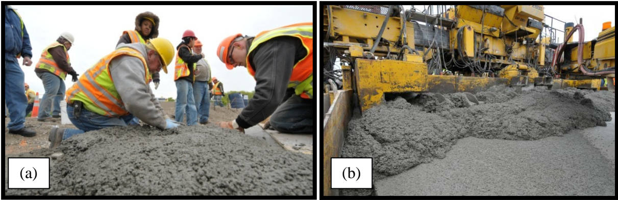
Figure 13: (a) Fresh Concrete Testing and (b) MnROAD Mainline Cell 72 Construction
