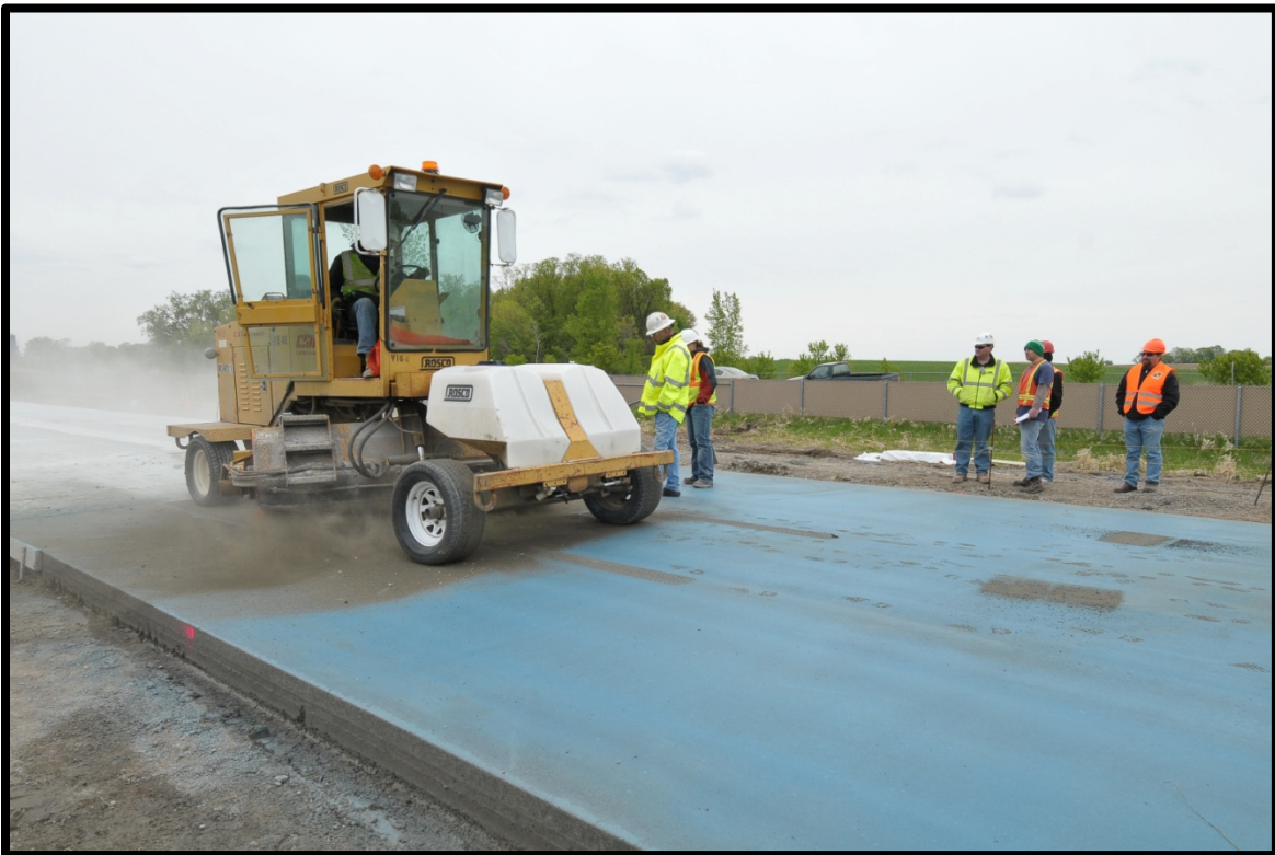
Figure 16: MnROAD Cell 72 Brushing (2)
