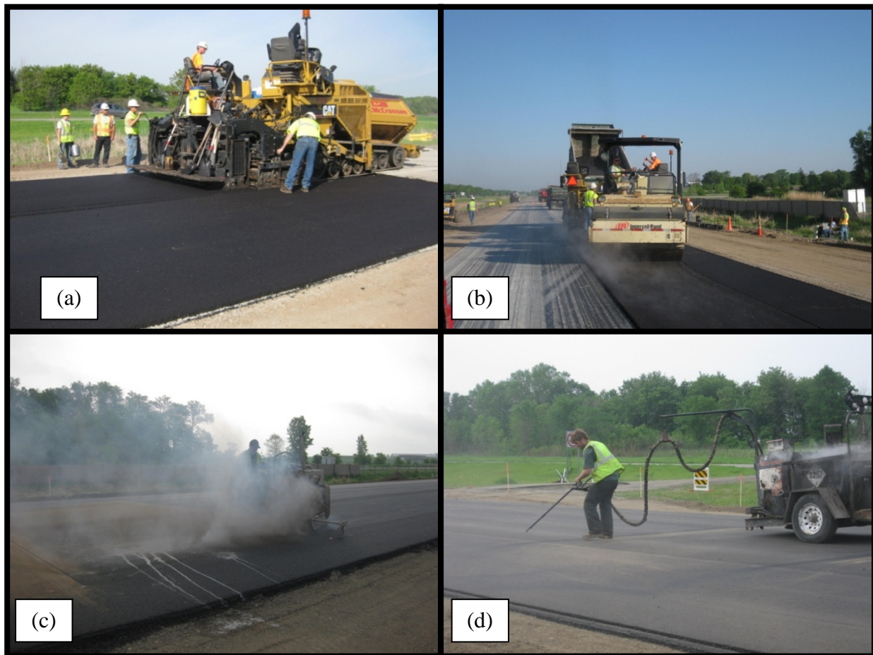
Figure 17: (a) through (d) MnROAD Mainline Cell 70 - Top Lift Construction
