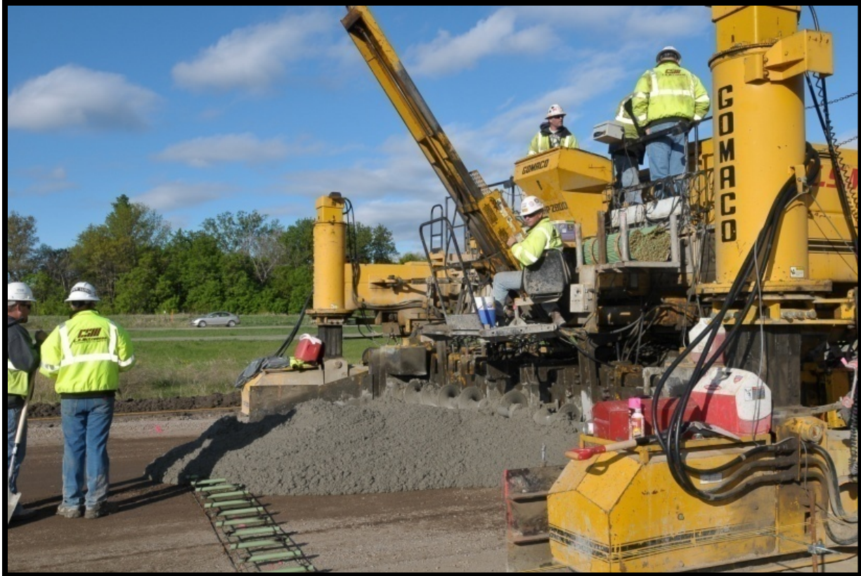
Figure 11: MnROAD Mainline Cell 70 – Lower Lift Construction
