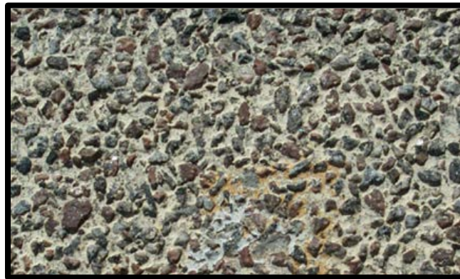
Figure 10: Demo Slab Finished Surface
