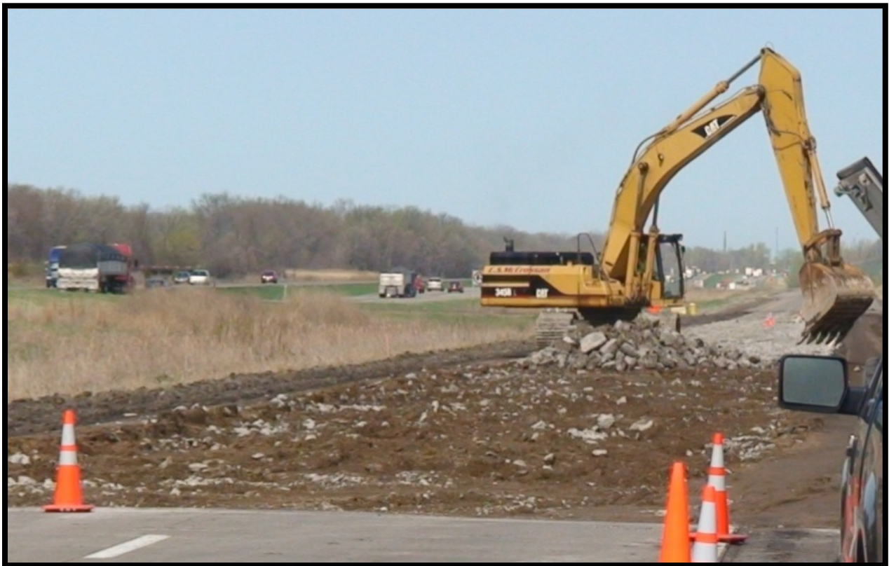
Figure 6: PCC Removal
