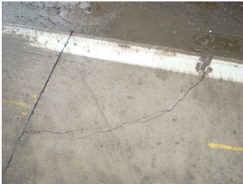
Figure 6.25. New corner break on cell 32 during spring 2010 testing
