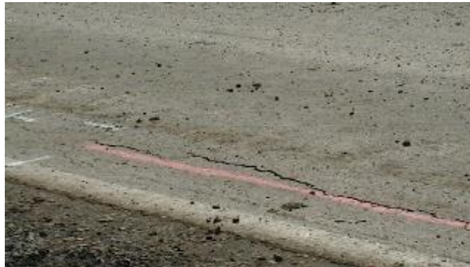
Figure 3.21. Failure at cell 83 westbound lane on 18 th March 2009
