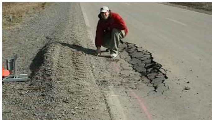
Figure 3.22. Failure at cell 83 westbound lane on 19 th March 2009
