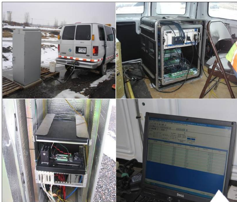
Figure 3.14. MnROAD pavement response data collection system
