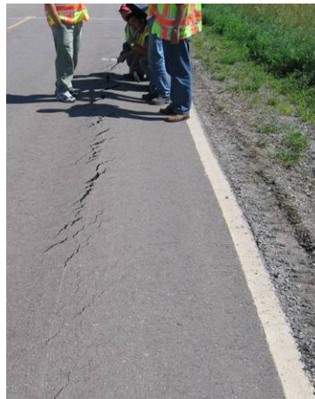
Figure F.1. Pavement failure in cell 83 eastbound lane
