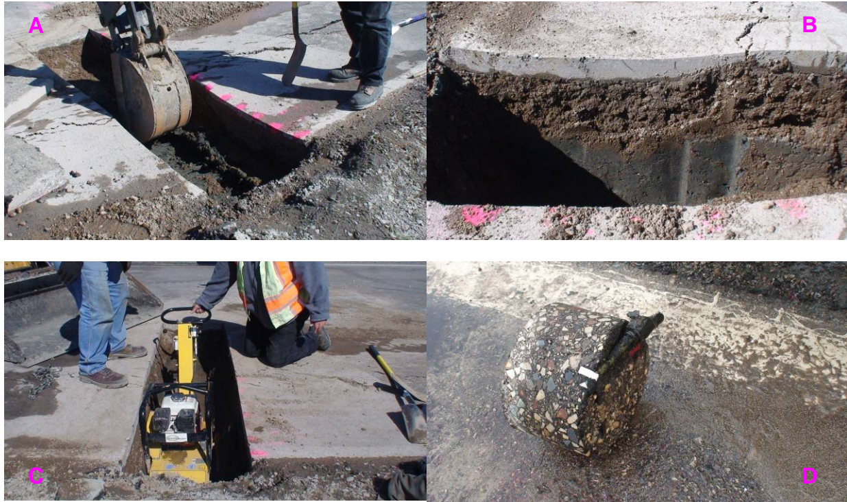
Figure F.2. Forensic activities: (a) removing material with backhoe, (b) forensic trench, (c) compacting backfill, (d) asphalt core with strain gauge
