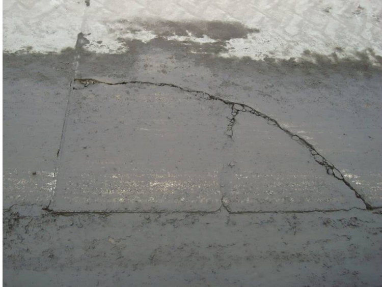
Figure 6.24. Aggravated corner break from fall 2009 testing cycle
