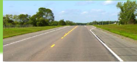
Hwy 71 @ Reference Point 173.998
