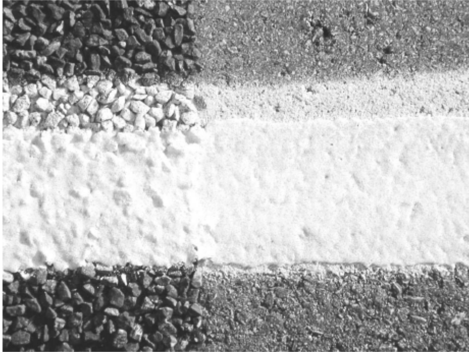
Figure 4. Thermoplastic Marking on Seal Coat (left) vs. HMAC (right) (4)
