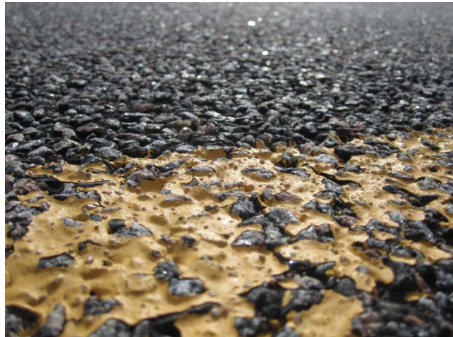
Figure 22. Aggregate Size and Marking Damage
