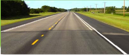
Hwy 25 @ Reference Point 81.993
