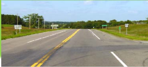
Hwy 71 @ Reference Point 169.958
