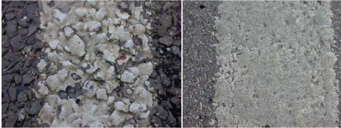
Figure 5. Thermoplastic after Two Years (Seal Coat on Left vs. HMAC on Right) (4)
