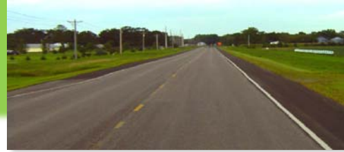
Hwy 47 @ Reference Point 67
