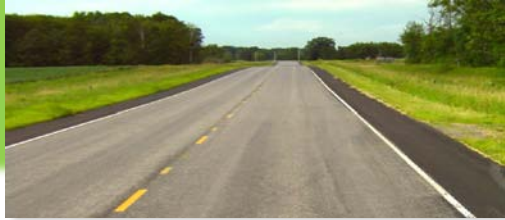
Hwy 47 @ Reference Point 60
