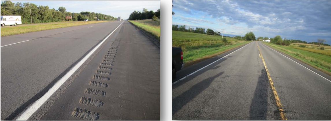
Figure 23. Example Roadway Characteristics
