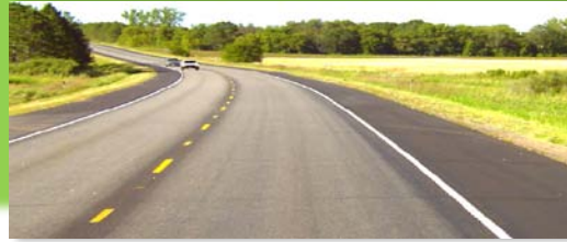
Hwy 25 @ Reference Point 93.020
