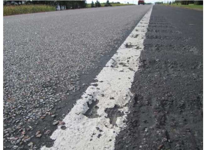
Figure 18. Rumble Stripe Damage
