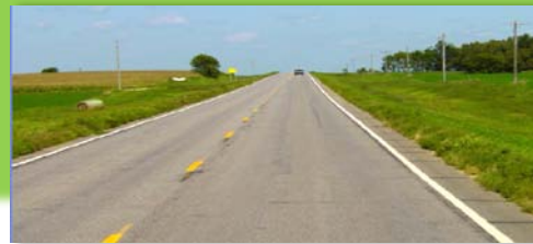
Hwy 4 @ Reference Point 162.998
