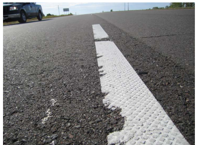
Figure 20. Damage to Tape after 1 Year on Micro Surface
