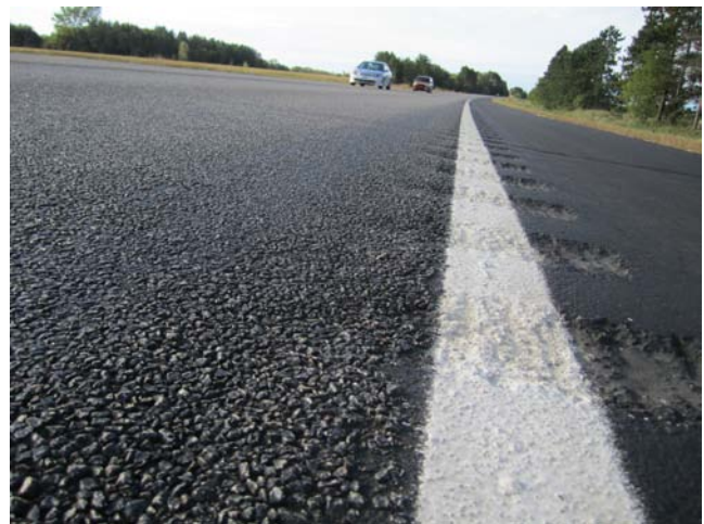
Figure 17. Rumble Stripe Placement Outside of Seal Coat
