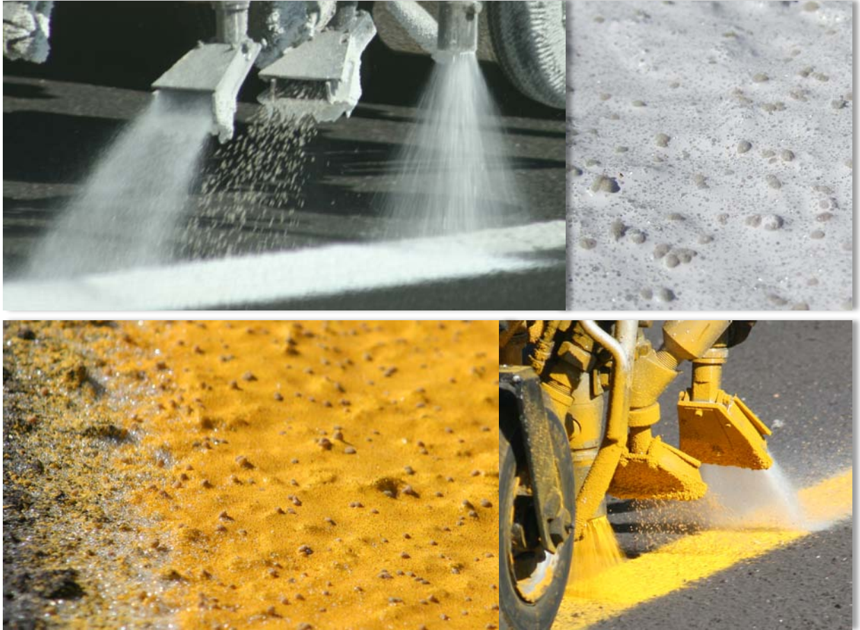
Figure 11. I-94 Micro Surface Project Permanent Marking Placement
