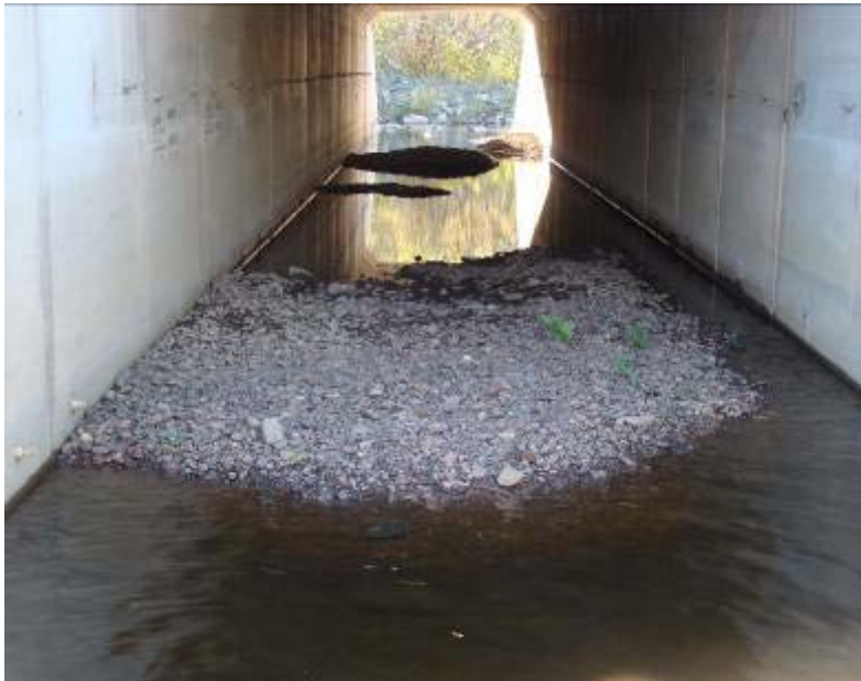
Figure 5.4. Photograph showing gravel and small cobble accumulating in the side barrel at Beaver River site (St. Louis County).
