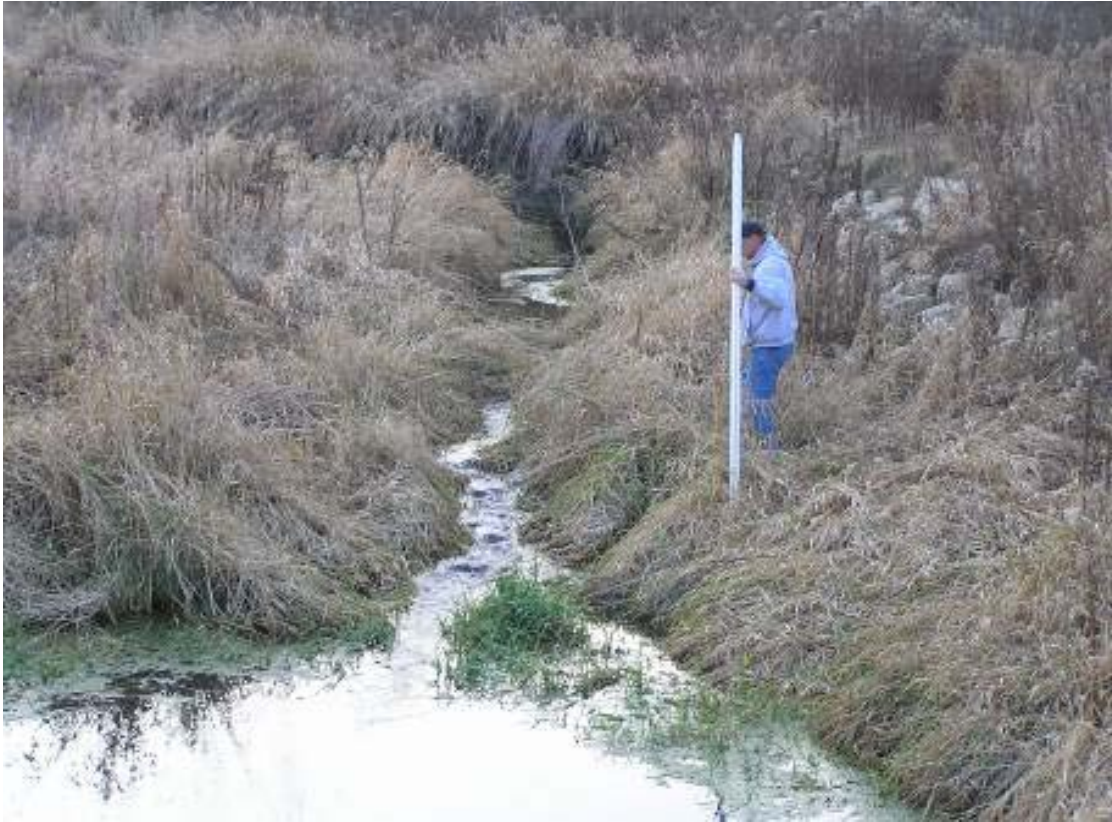
Figure 5.1. Photograph of rip-rap placed at upstream end of the pool to prevent the formation of a head cut developing from the recessed culvert installation.
