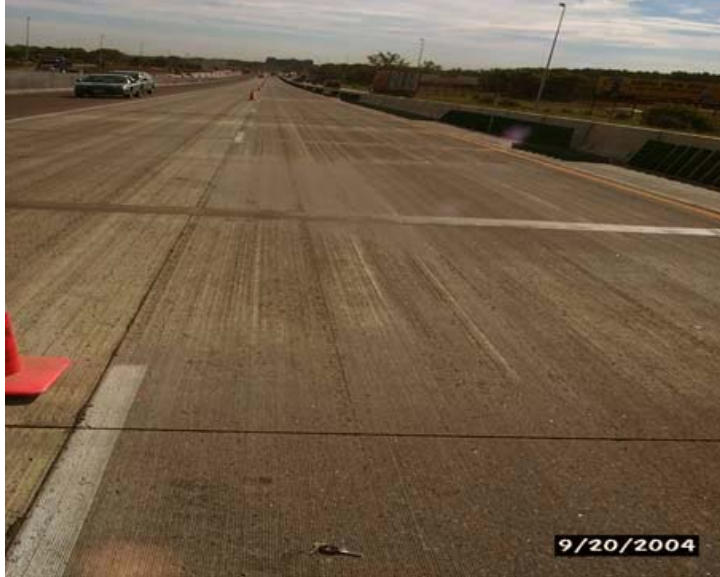
Figure 2.8: Concrete Pavement with Longitudinal Broom Drag
