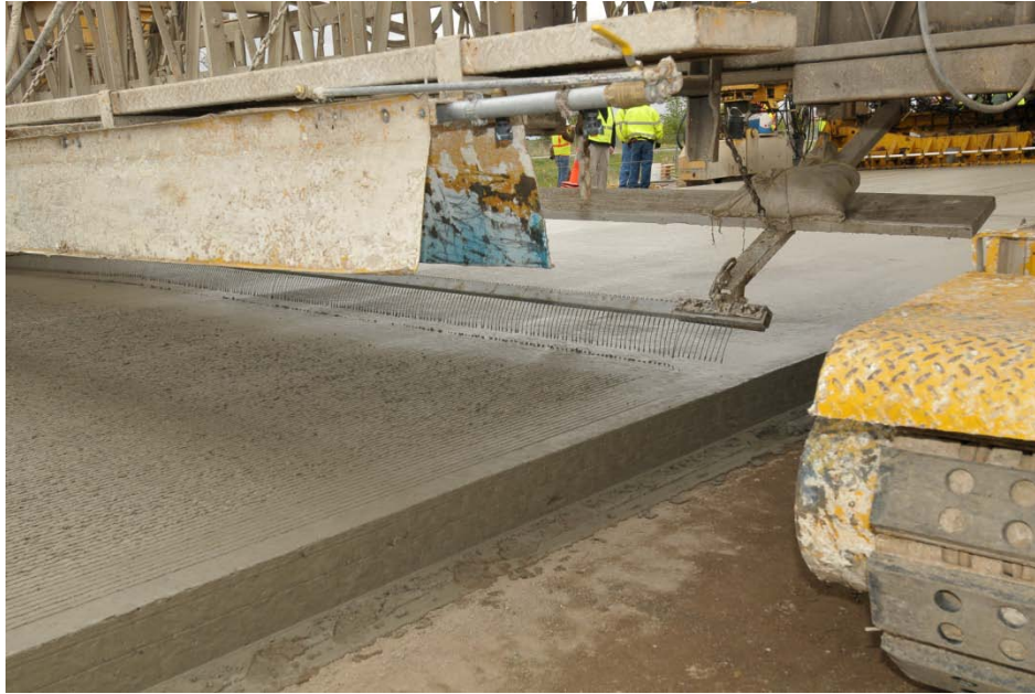
Figure 2.5: Longitudinal Tining on Concrete Pavement
