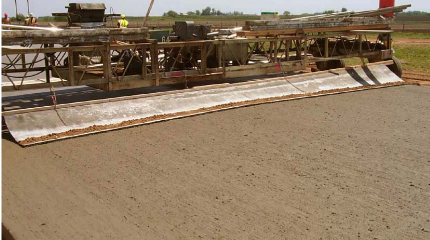
Figure 2.6: Concrete Pavement Finishing with Inverted Piece of AstroTurf
