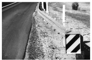
guardrail exits the head safely and the vehicle is brought to a controlled stop. When impacted along the side within the length-of-need, the FLEAT-350<sup>TM</sup> functions like guardrail. The errant vehicle is safely redirected back toward its original travel path.
