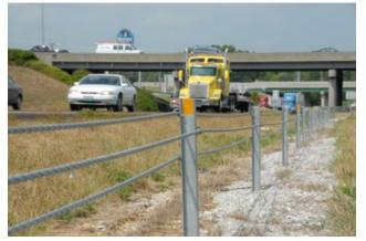
resists impact using cables tied to PCC anchors. Post spacing is typically 12 feet-6 inch but can be reduced to limit deflections. High deflections of 10 feet can be expected with a 4500 pound vehicle at 60 mph and at a 25 degree hit, with a 12 feet-6 inch post spacing. The posts are designed to break off instead of leaning on impact, reducing roll-overs. Three-Cable guardrail systems have passed NCHRP-350 standard for a weak post design.
