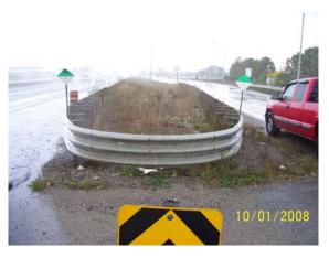
**Design:** Surrounds the hazard from every direction. Designed to act as a strong post thrie-beam guardrail without any hard ends that need to be treated.
