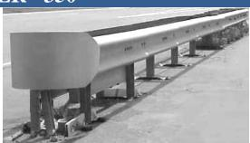
breakaway assembly, the W-beam telescopes, the posts break and the cable acts to help absorb the energy and bring the vehicle to a safer stop. Redirects when hit from the side.
