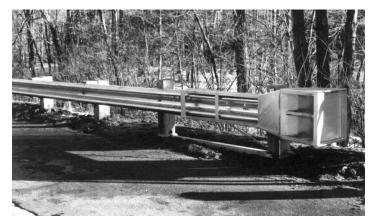
length-of-need, the SKT-350<sup>TM</sup> functions like guardrail. The errant vehicle is safely redirected back toward its original travel path.
