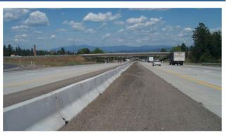
**Design:** Rigid barriers are constructed 32 inches high and will not deflect when hit. Construction consists of slip-formed, pre-cast, or cast-in-place. Concrete barriers can be placed directly on the pavement or a footing. Additional height may be added if busses or trucks are expected to require this type of guardrail protection. Commonly referred to as Jersey barrier.
