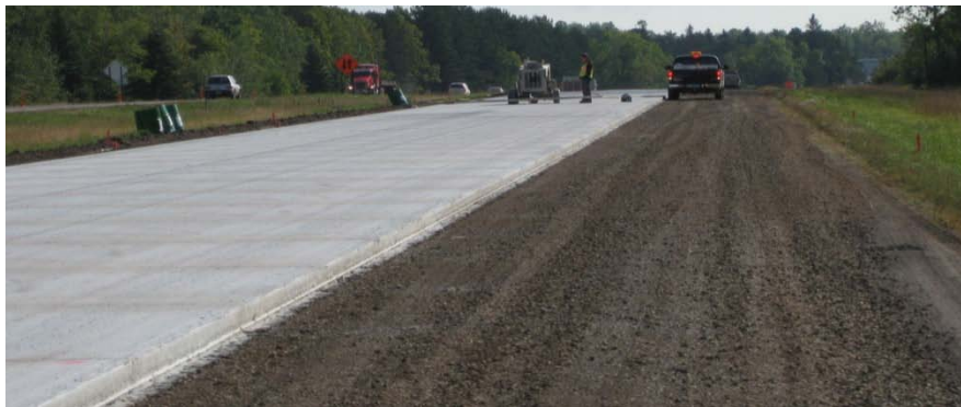
Figure 3.7. TH 53 Thin Unbonded Concrete Overlay, September 2008
