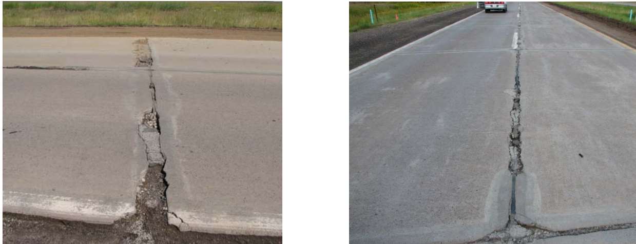
Figure 3.4. Typical Transverse and Longitudinal Joint Condition Prior to Overlay
