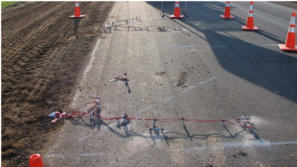
Figure 2.4. Installed Instrumentation Prior to Paving the Overlay [September 9, 2008]
