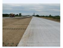
The new smoothness specification covers newly constructed concrete pavements like this one as well as asphalt pavements.
