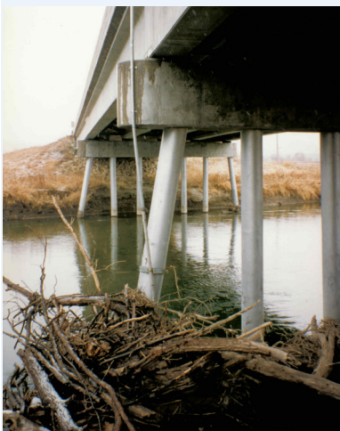
Debris can damage monitoring equipment, limiting or eliminating its effectiveness.
