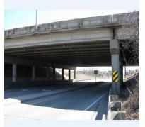
Mn/DOT cares for more than 1,200 prestressed concrete bridges built between 1929 and 2005.
