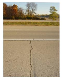
Low-temperatures cause asphalt pavements to contract, which may lead to cracking. Asphalt mixtures and binders that are not as rigid in cold temperatures are better able to relax stresses, making pavements less brittle and prone to fracture.
