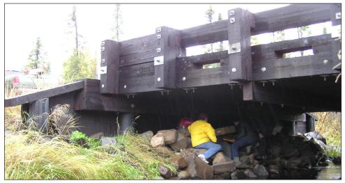
Researchers examined the potential for using vibration testing to assess the structural health of dowel-laminated bridge systems—wooden bridges constructed with laminated timbers held together transversely by metal dowels and supported by a spreader beam.
