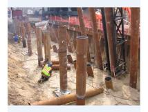
Pile capacity can increase significantly because pore water pressure created during pile driving dissipates and increases soil strength.
