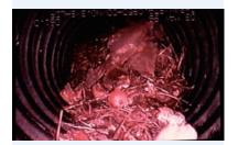
Rodent nests within the drainage pipe are one of the more common maintenance problems for subsurface drainage systems.
