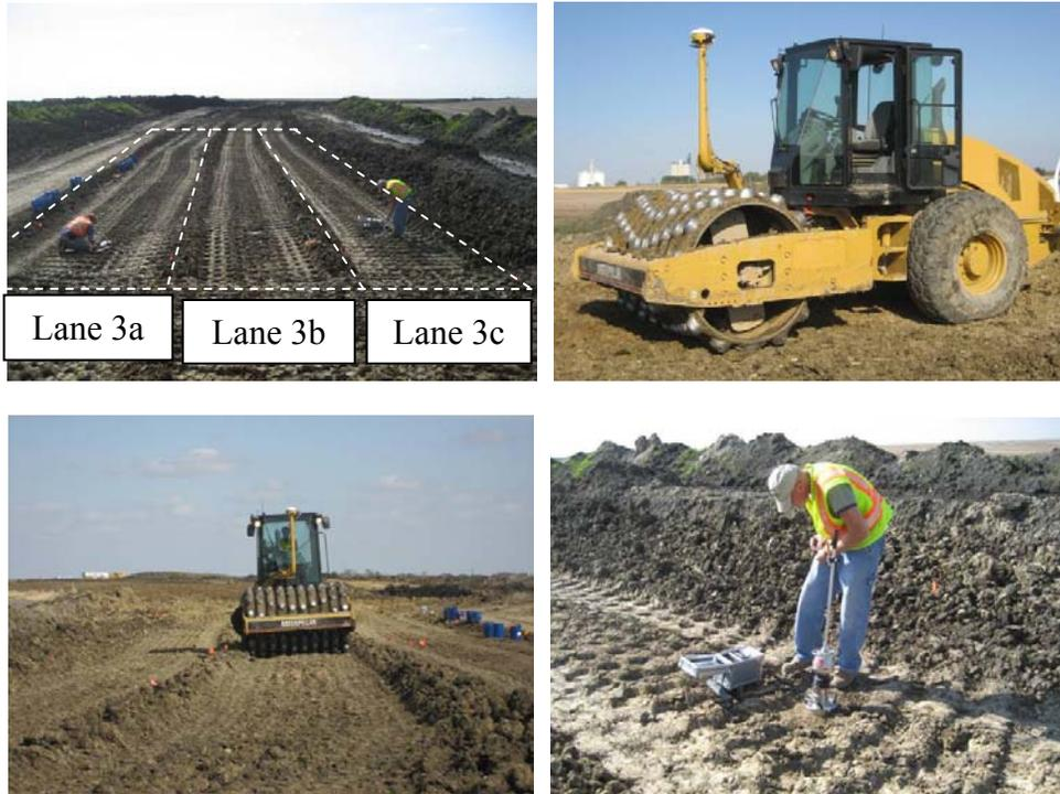
Figure 3.83. Test strip 3 prepared in three lanes (lanes 3a, 3b, and 3c) for rolling (top left), picture of roller used on-site (top right), rolling operations (bottom left), and LWD testing (bottom right) in at the bottom of the padfoot penetration
