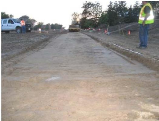
Figure 3.49. Compaction operations on test strip 5 with relatively uniform conditions across the test strip
