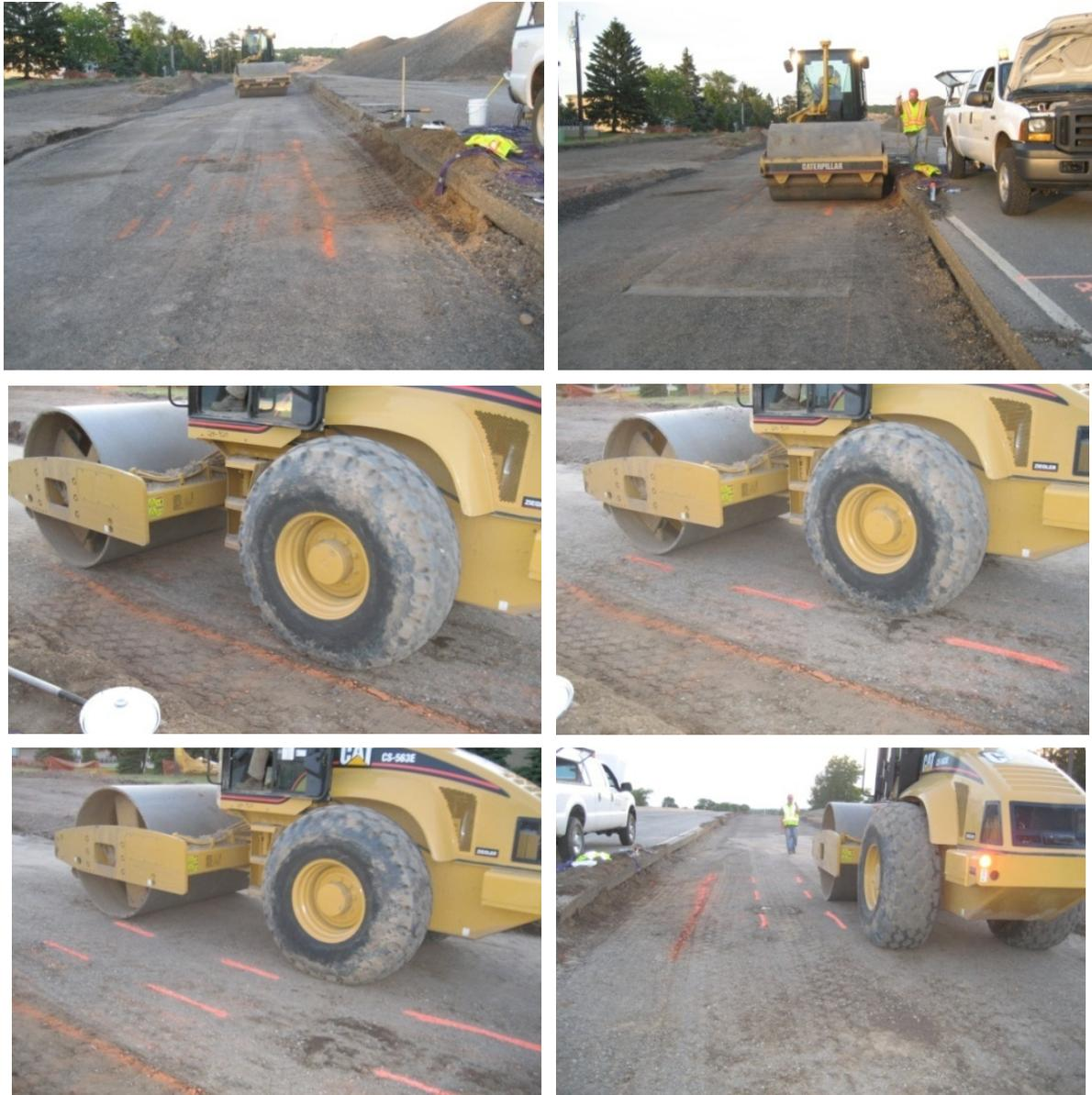
Figure 3.18. Pictures showing rolling pattern on test strip 3
