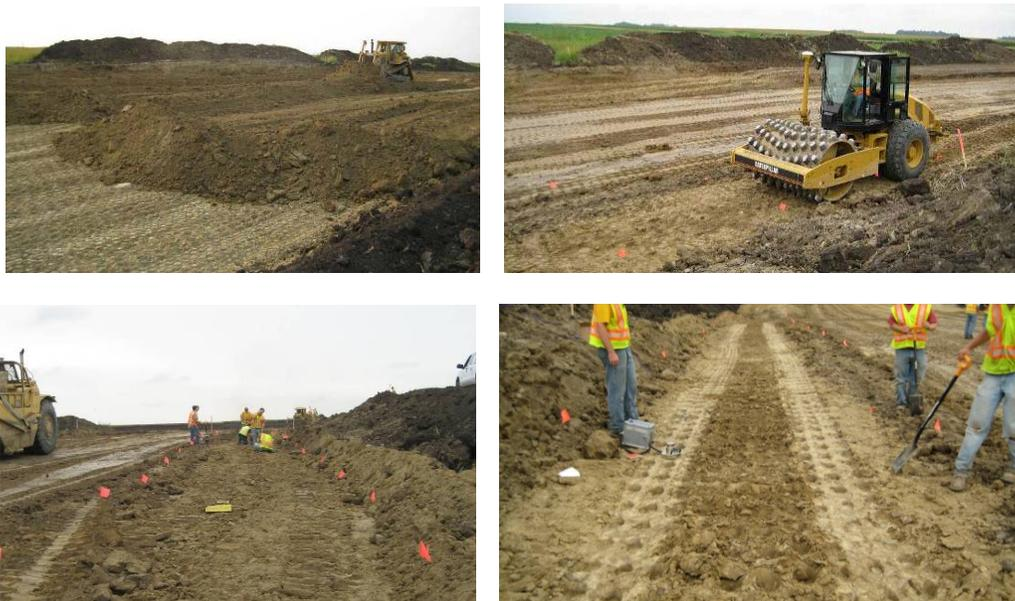
Figure 3.76. Pictures from test strip 2 construction: fill placement, compaction, in-situ spot testing, and final compacted surface (top left to bottom right)
