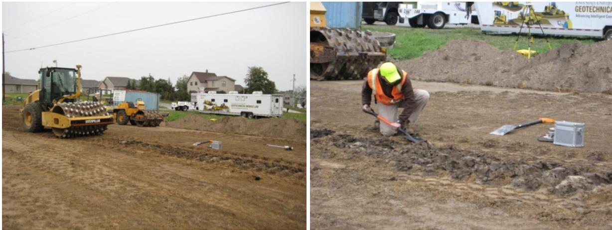
Figure 3.104. IC padfoot roller (left) and LWD test preparation (right) by excavating to bottom of padfoot penetrations
