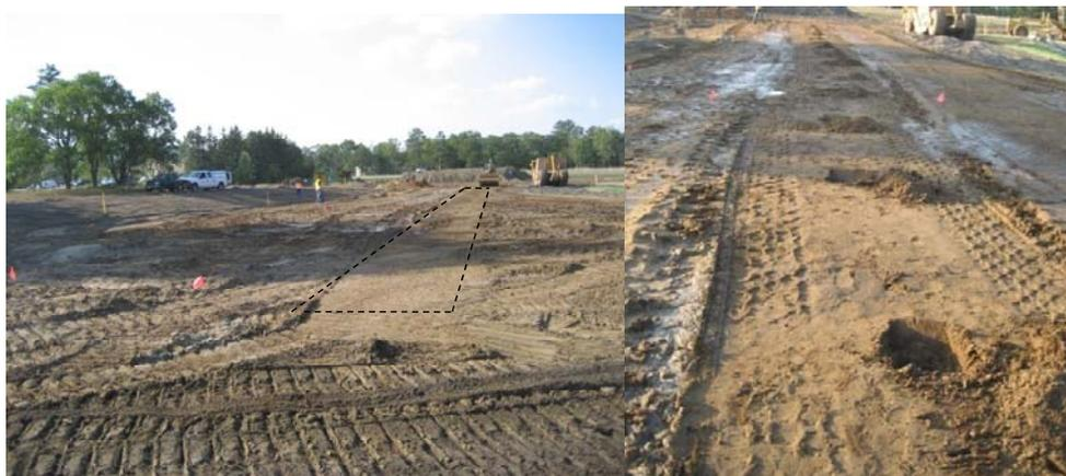
Figure 3.46. Compaction operations on test strip 3 (left) and excavations performed for LWD testing
