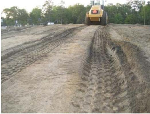
Figure 3.48. Compaction operations on test strip 4 with soft and uncompacted material
