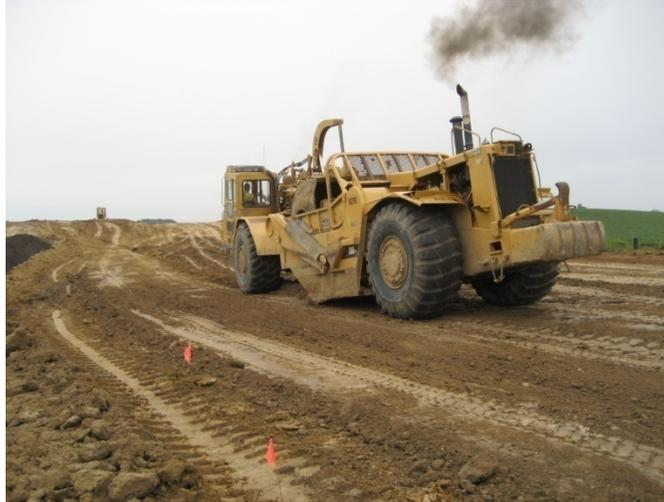
Figure 3.67. Scraper traffic contributing to compaction of fill materials
