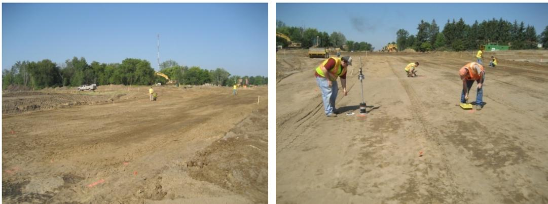
Figure 3.38. Photographs of test strip 2 after final pass (left) and in-situ testing (right)
