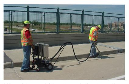
Sealing cracks in concrete decks is a routine part of bridge maintenance, but practices and products vary significantly. This study established best practices guidelines for concrete deck and crack sealing on Minnesota's bridges.
