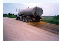
Dust control products could be sprayed by trucks used for applying asphalt products.
