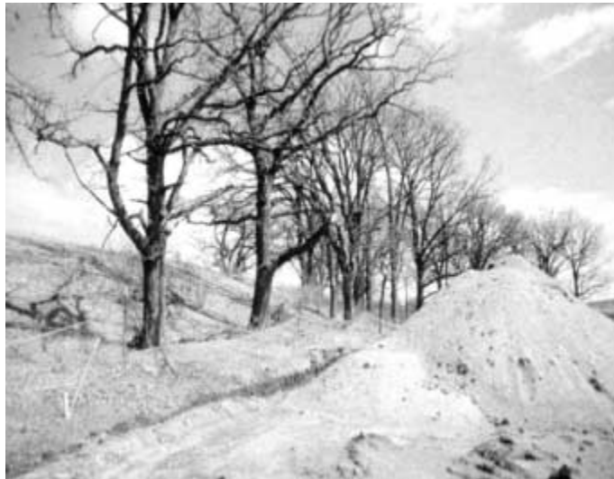
Figure 9-11. Using Temporary Tree Protection Fencing or Silt Fence - keeps equipment and construction activities off the tree root systems and trunks.
