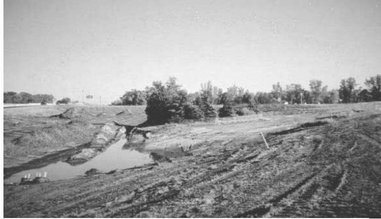
Figure 9-12. Protecting Trees during Construction
