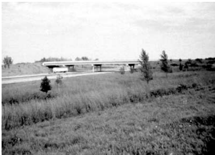
Prairie Restoration Project on Interstate 90
