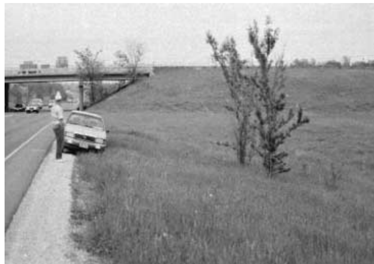
Remove trees that are hazardous roadside obstacles (in safety clear zone) when they are small.
