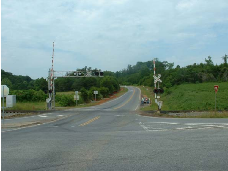
FIGURE 4-9 View of Railroad Crossing from the East Approach of GA 140
