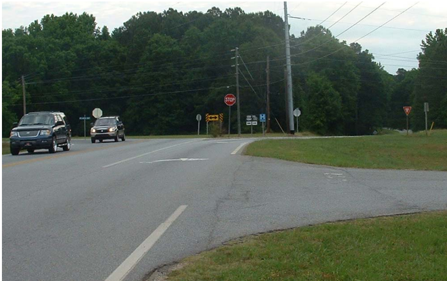
FIGURE 4-4 Northbound Approach of GA 83
