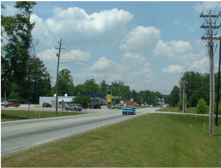
FIGURE 4-5 On GA 54 Looking North at Candidate Intersection
