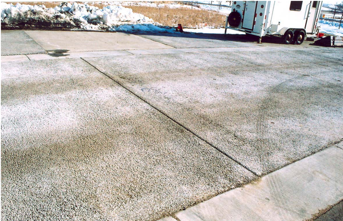
Figure C1. Tooled Joint, Cell 64 Facing Southeast, 9.21.06
