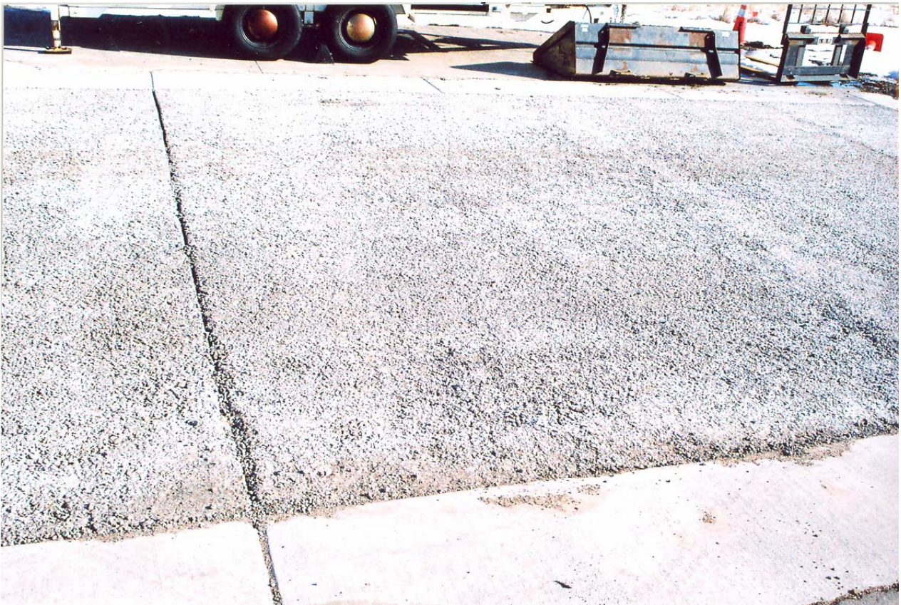
Figure C2. Header/Construction Joint, Cell 64 Facing Southeast, 9.21.06
