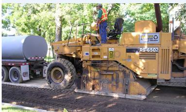
A water truck and road-reclaimer blended the ash, water and reclaimed pavement materials on 7th Avenue in Waseca.
