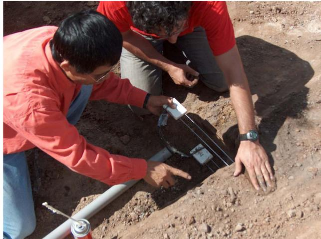
Researchers installed water content and temperature sensors to monitor the subgrade and road surface gravel on the newly paved County Road 53 in Chisago County for moisture and trace element levels.
