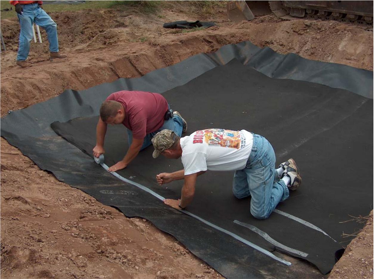
**Fig A16. Placement of geomembrane and geotextile.**
