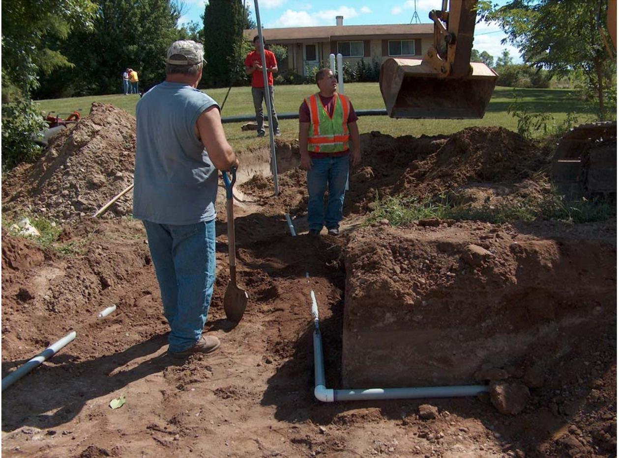
**Fig A19. Installation of temperature sensors into subgrade and RSG in lysimeter pit. Sensor 6 is in subgrade and Sensor 5 is in RSG.**
