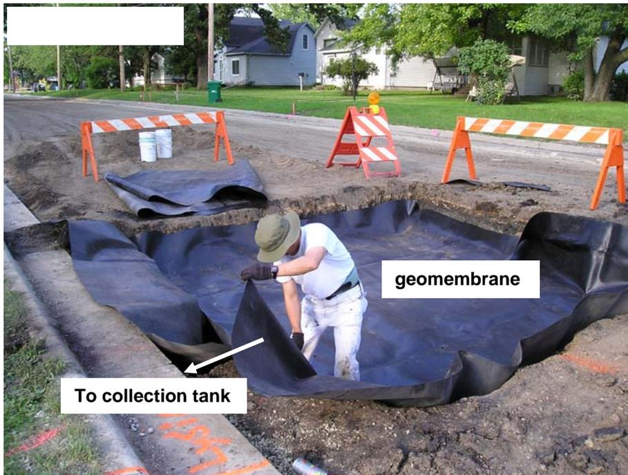
Fig. B1. Installing geomembrane for lysimeter.
