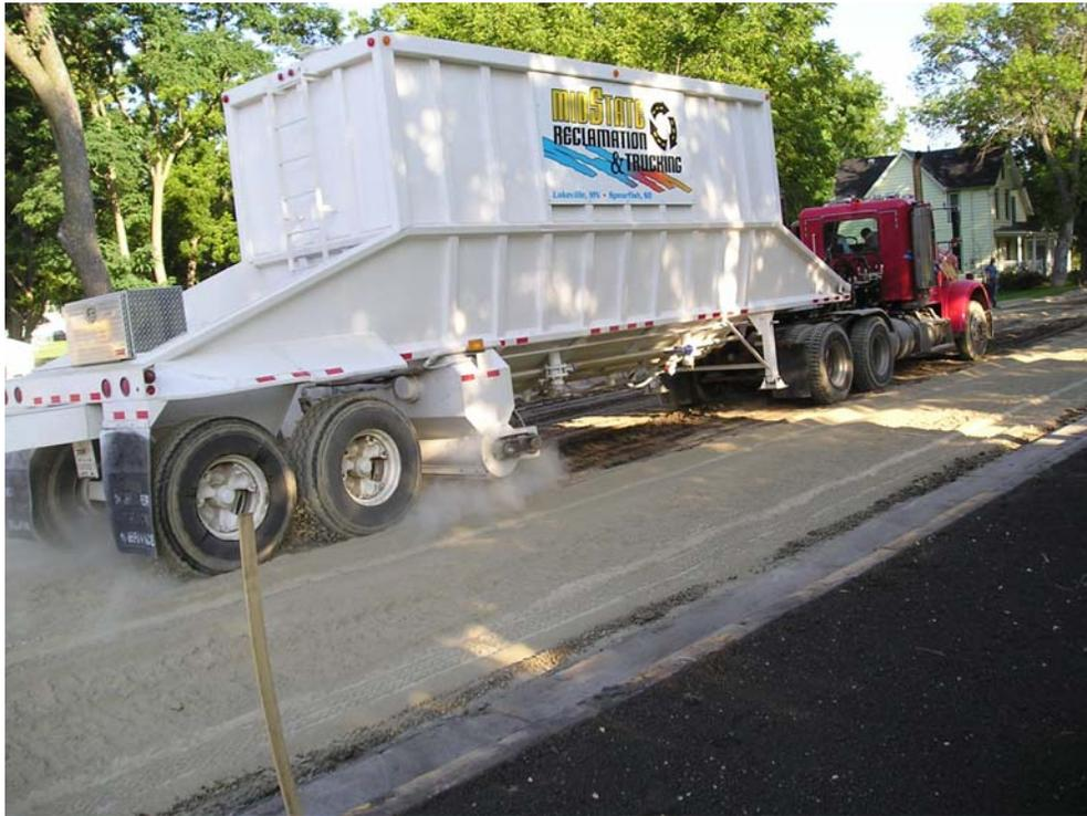
Fig. A2 Lay-down truck placing fly ash on SRPM.
