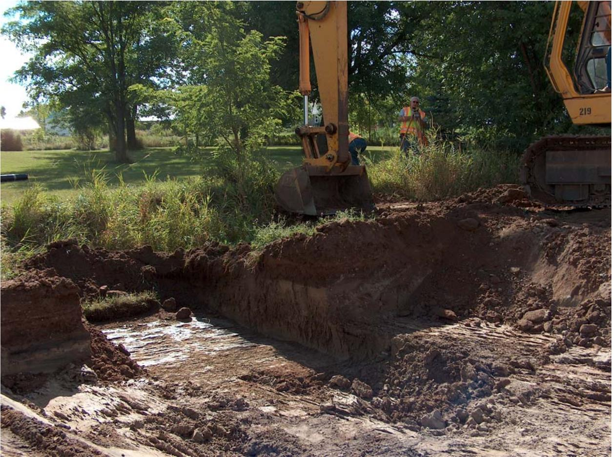
**Fig A14. Excavation of lysimeter pit.**
