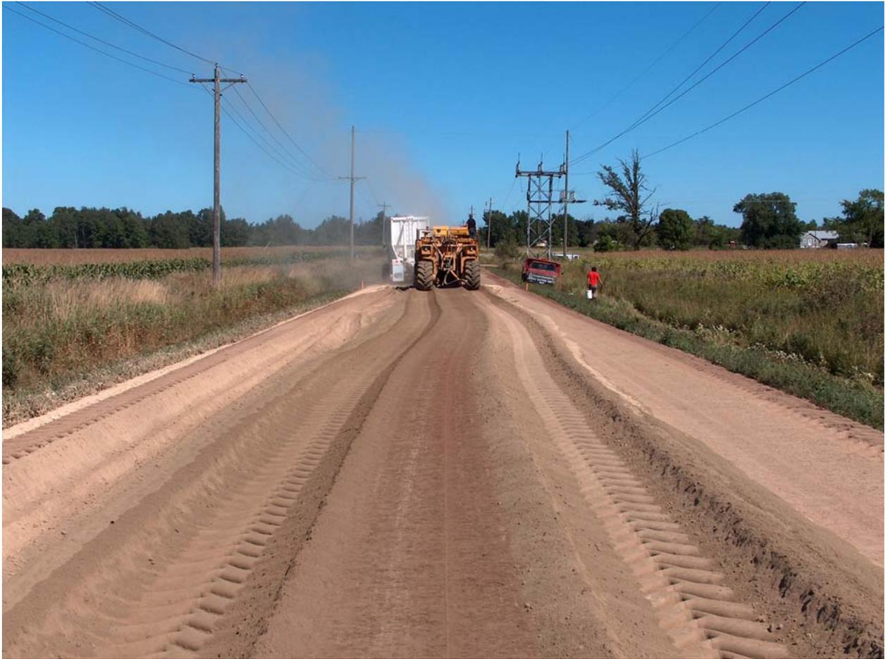
**Fig A8. Road surface after blending process.**
