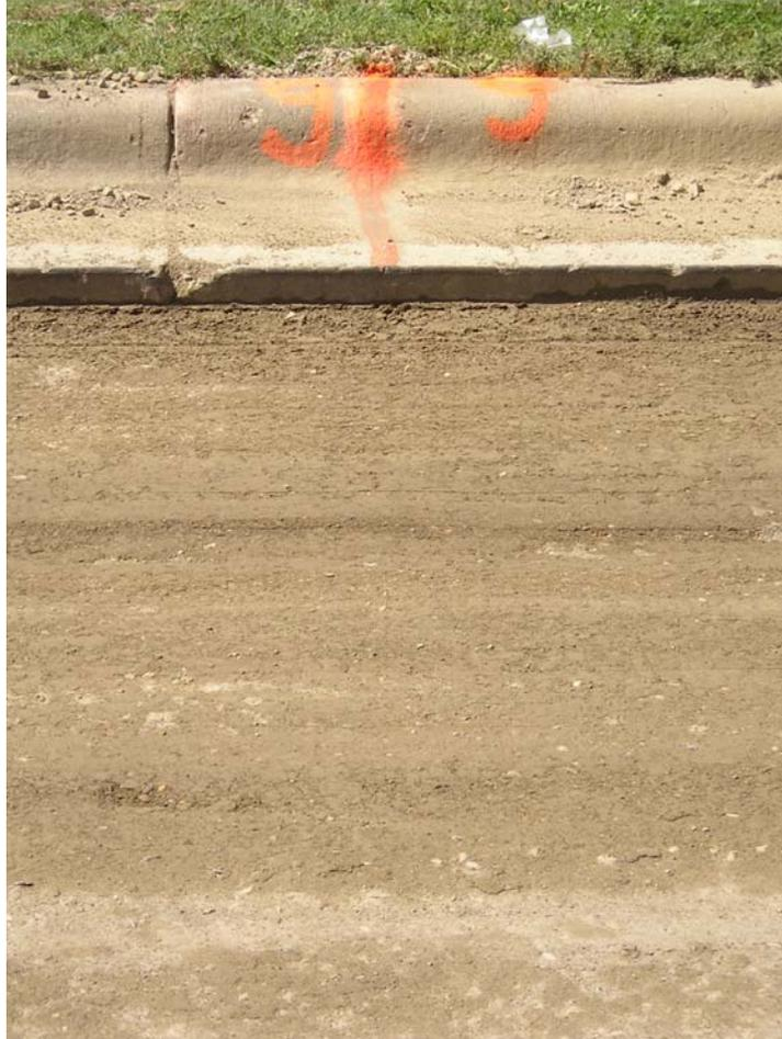
Fig. A4. Surface of SRPM after compaction.
