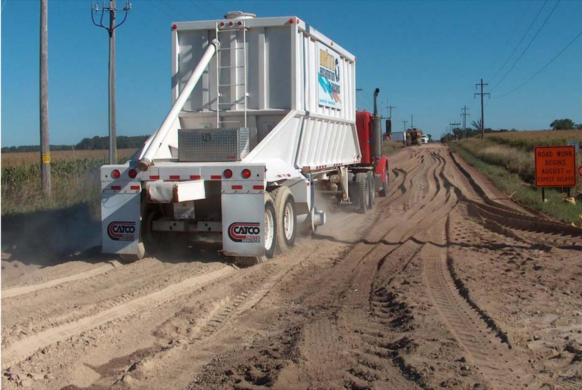
**Fig A6. Lay-down truck placing fly ash on RSG**
