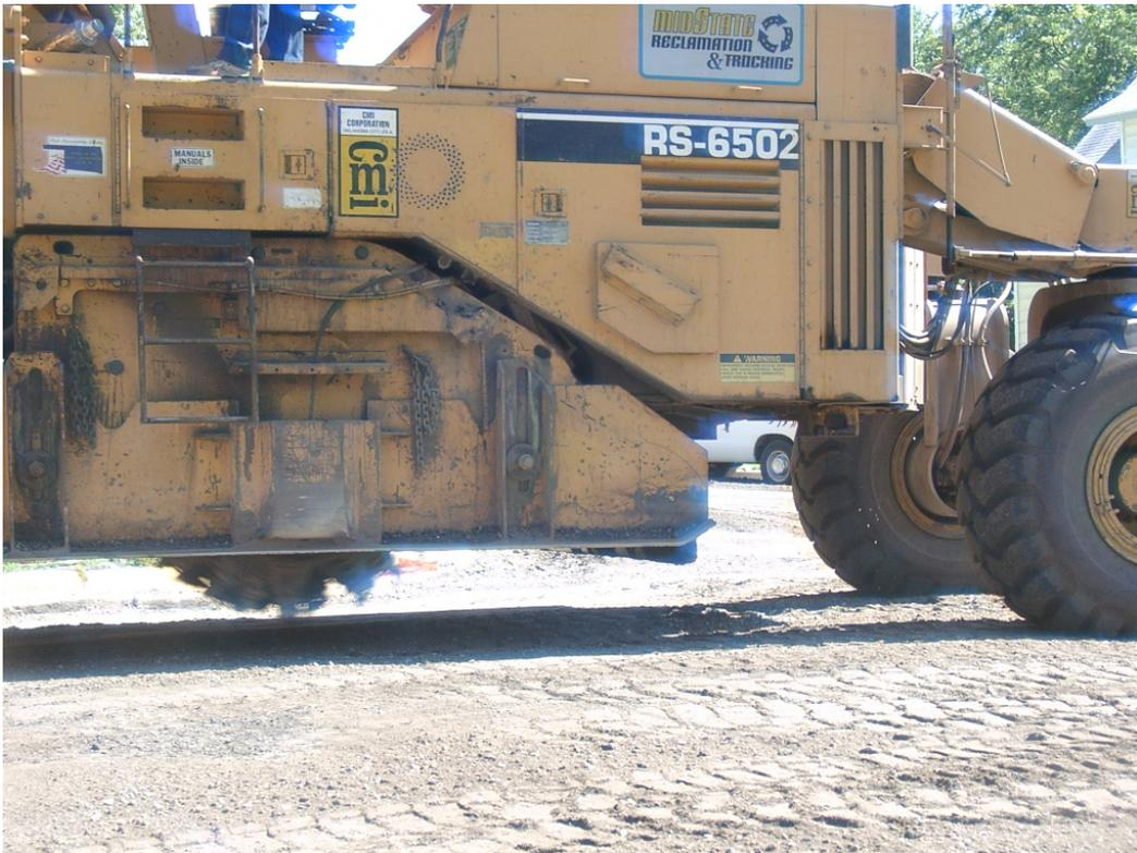
Fig. A5. Mid-section of road-reclaimer showing tines used to blend fly ash, water, and RPM.
