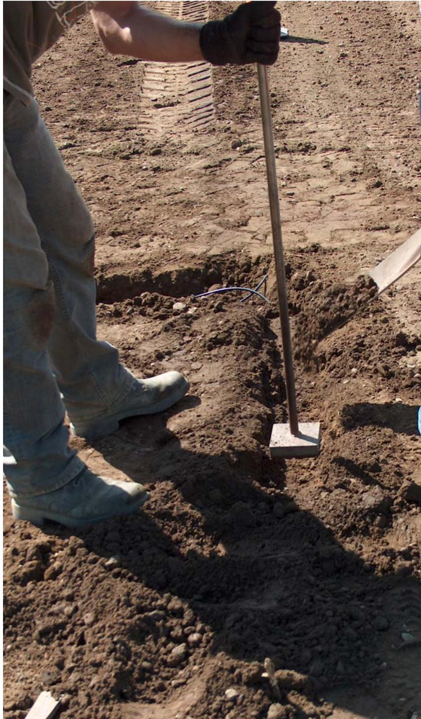
**Fig A21. Compaction of sensor trench with a hand compactor in S-RSG**
