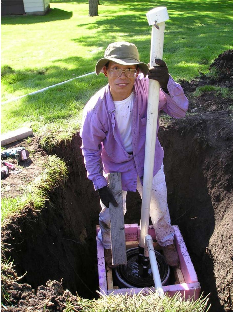
Fig. B2. Installing collection tank for lysimeter.
