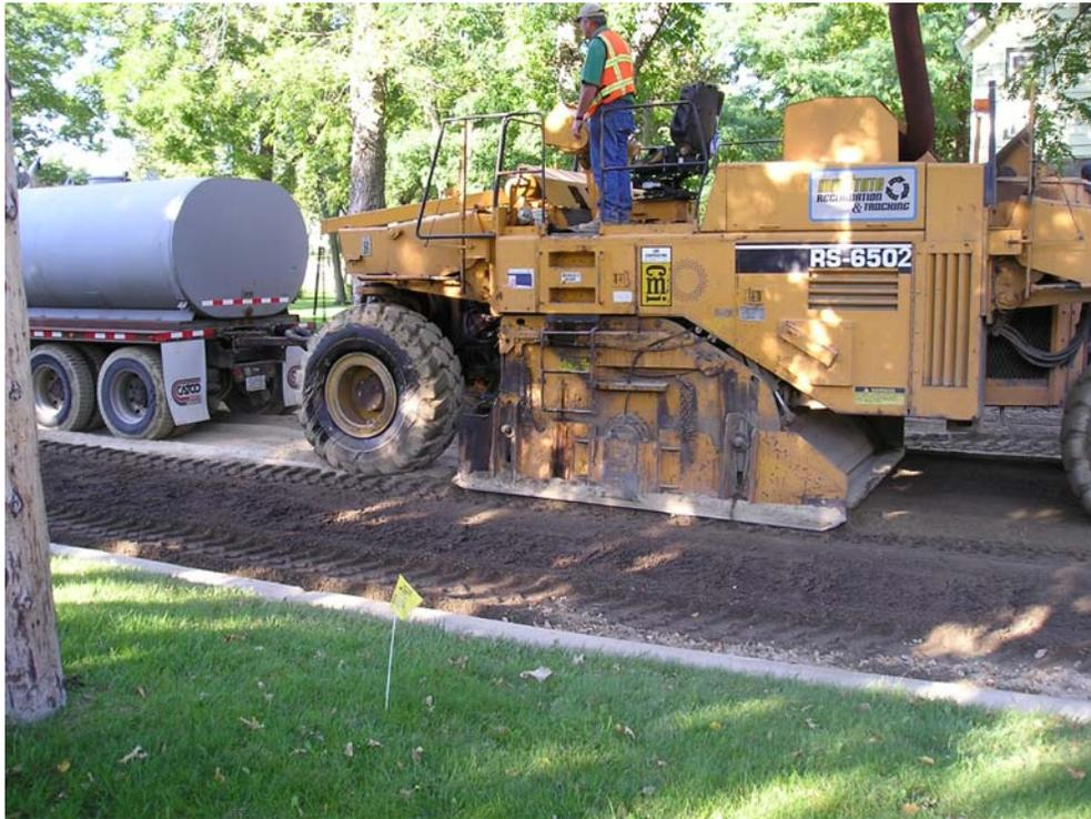
Fig. A3. Water truck and road-reclaimer blending fly ash, water, and RPM.
