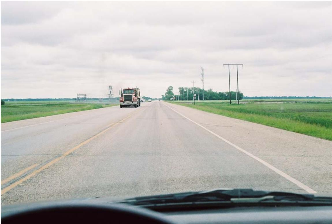
Photograph #361 (Reel #17, 7) (from West looking East): first rumble strips in view. [Note: a rail crossing warning and a warning sign (on the left-hand side of the road) both precede the first rumble strip. In addition, the distance between the “stop ahead” warning and the location of the rumble strips is unusually long.]
