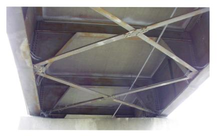
Lateral wind bracing, provided by the crossed steel ties shown above, was an important component to include in the model of the bridge in order to properly reproduce the measured stresses.
