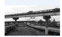
Researchers load-tested this bridge and found that the old methods for determining its carrying capacity underestimated the stresses actually measured.
