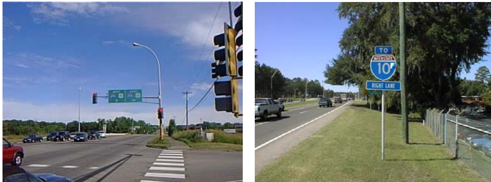
Figure E-3. Signs near I-694 and Lexington in St. Paul, MN (left) and I-10 (right)
