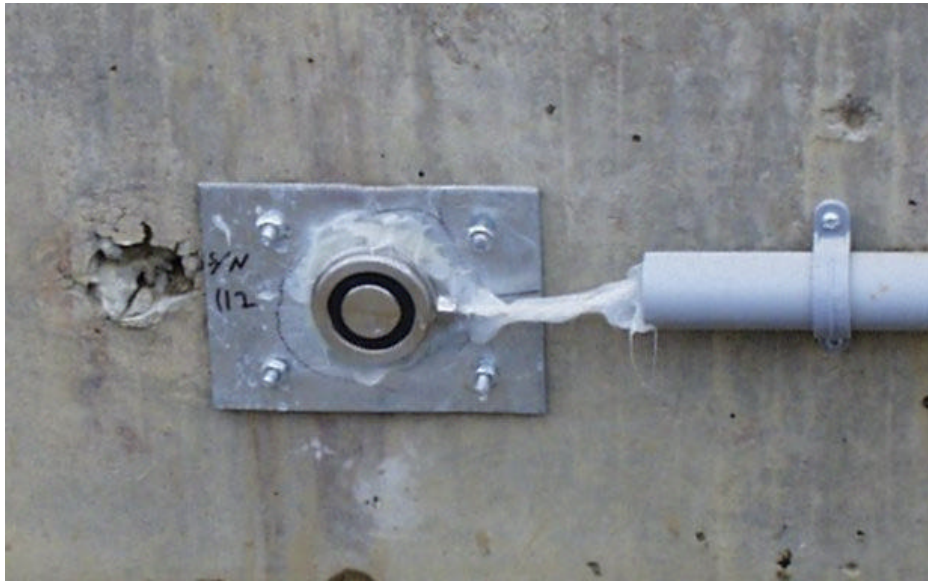
Figure 3.4. Kulite EPC attached to retaining wall.
