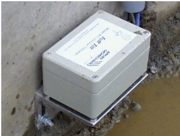
Figure 3.8. Tiltmeter attached to base of retaining wall stem.
