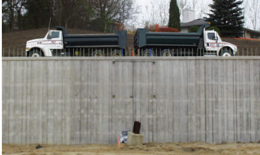
Figure 4.25. View towards front face of retaining wall during load test.
