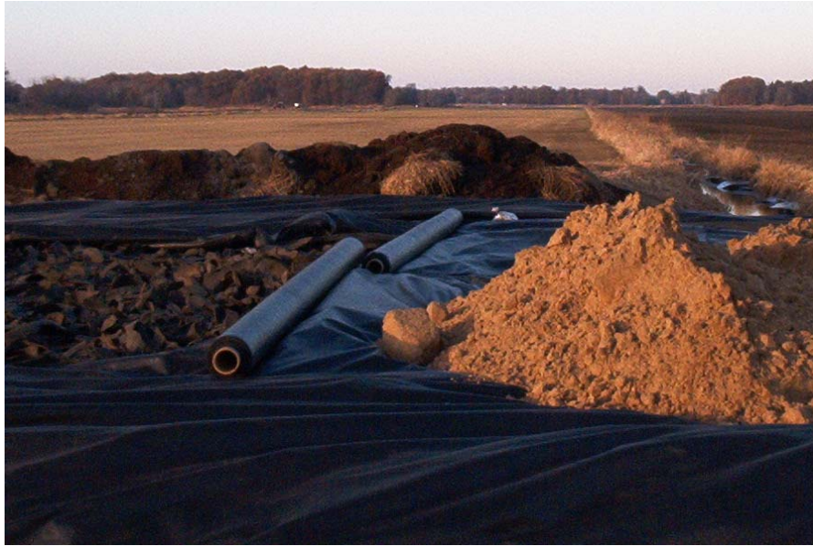
Figure 4.21 Geofabric and Fill being Placed over Tire Shreds
