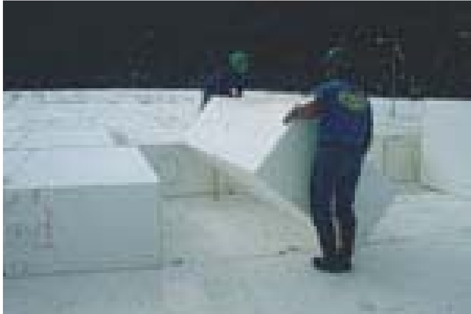
Figure 4.22 Placing Geofoam (EPS) Blocks (52).
