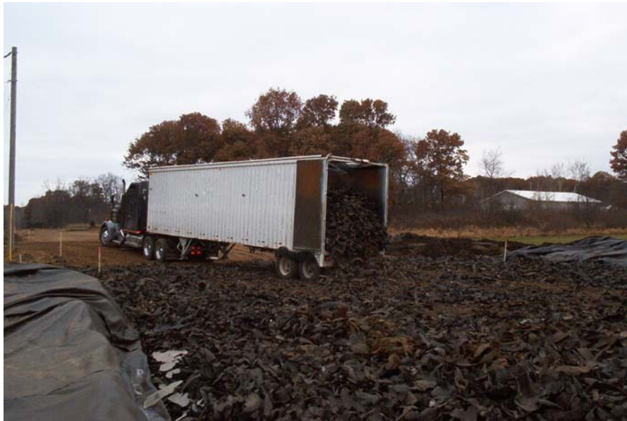
Figure 4.18 Live-Bottom Truck Delivering Tire Shreds
