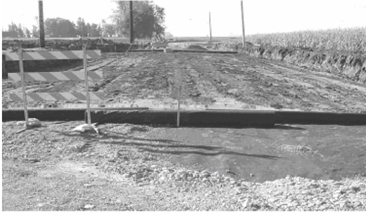
Figure 4.12 Overlapping Layers of Type V Nonwoven Geofabric Separate Granular Material from Wet, Fine Soil. 150-mm (6-in.) of Class 5 Granular Material Protects the Geofabric from the Breaker Run Material.
