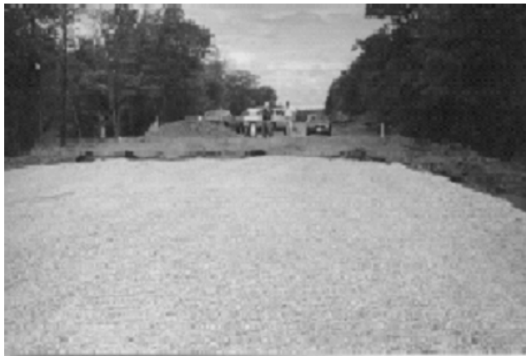
Figure 4.16 Wood Chips Placed on Geofabric
