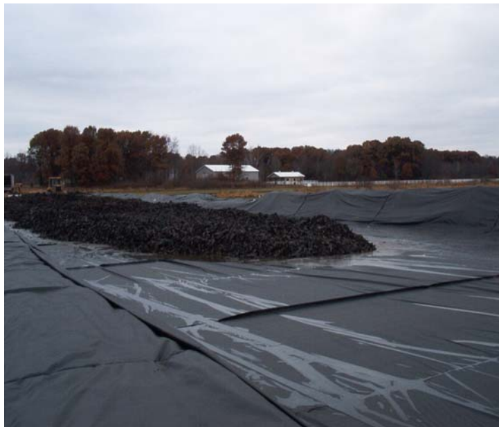
Figure 4.20 Tire Shreds Placed on Geofabric
