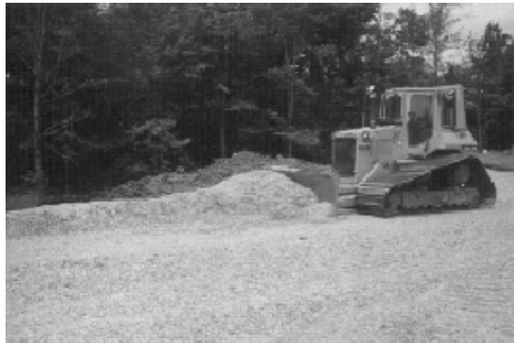
Figure 4.15 Bulldozer Spreading Lumber Mill Sawdust
