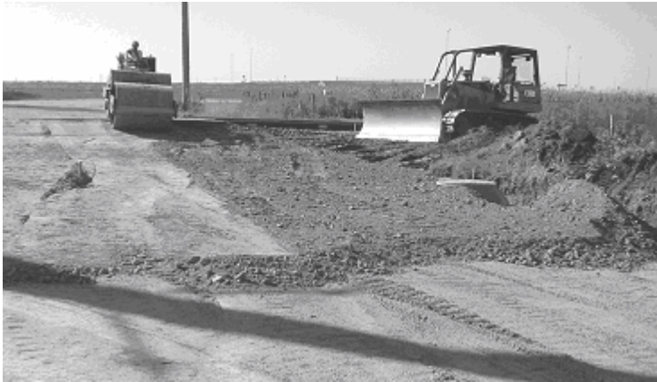
Figure 4.12 Overlapping Layers of Type V Nonwoven Geofabric Separate Granular Material from Wet, Fine Soil. 150-mm (6-in.) of Class 5 Granular Material Protects the Geofabric from the Breaker Run Material.
