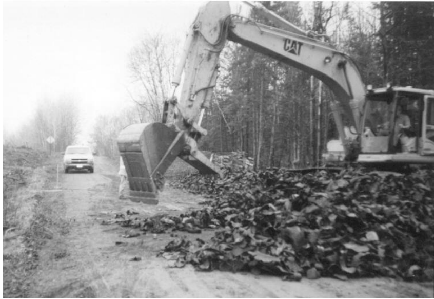
Figure 4.19 Placing Tire Shreds with “Thumb-Like Attachment
