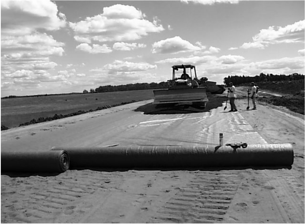
Figure 4.7 Granular Material placed on Overlapped Geofabric
