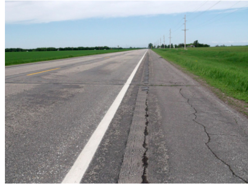
A California-style sinusoidal rumble strip, installed along a Polk County Highway.
