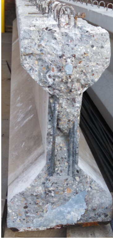
Figure F.3: Damaged end of Bridge 62834 girder (exposed stirrups)
