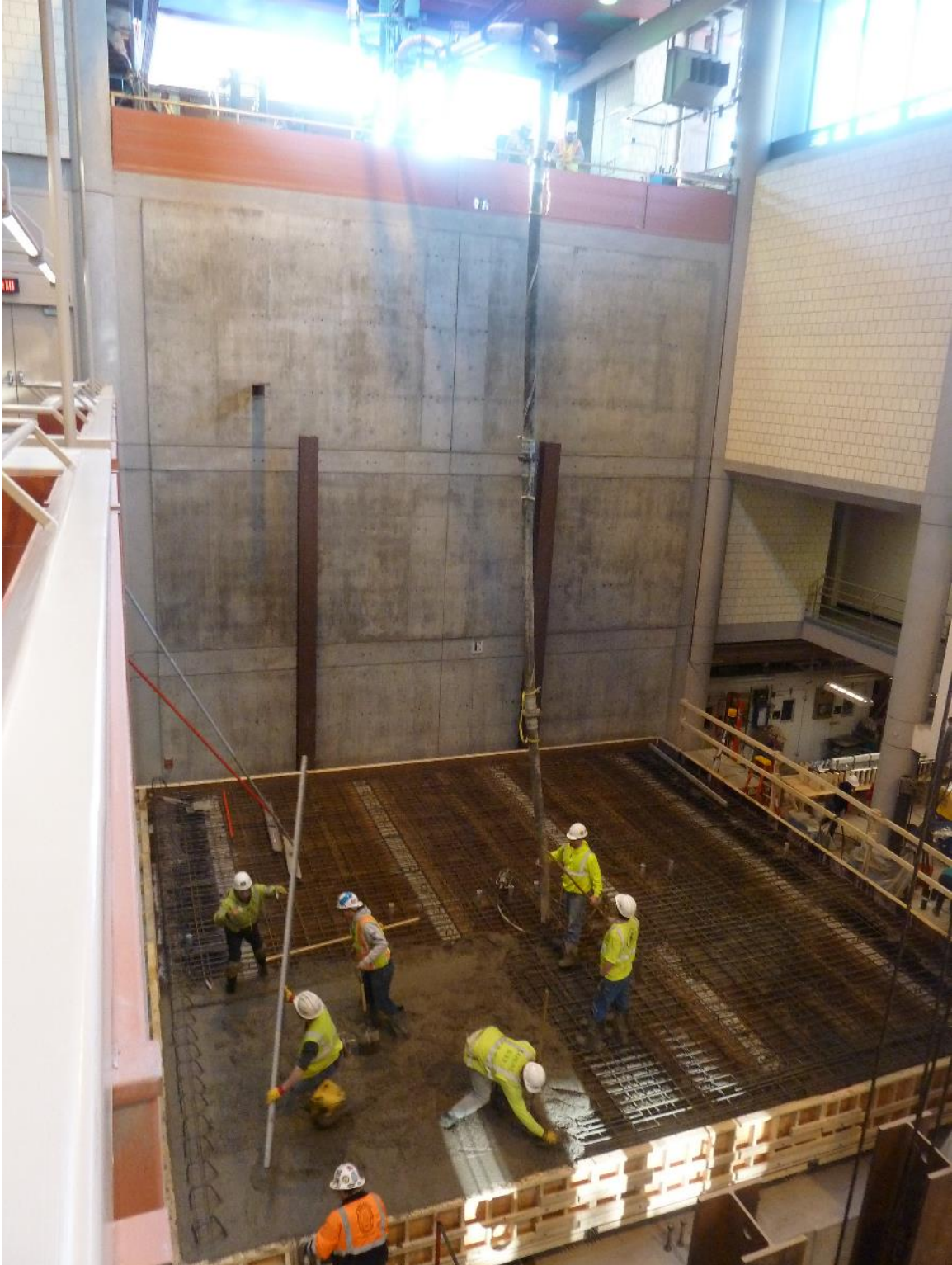
Figure 4.12: Bridge deck placement and finishing
