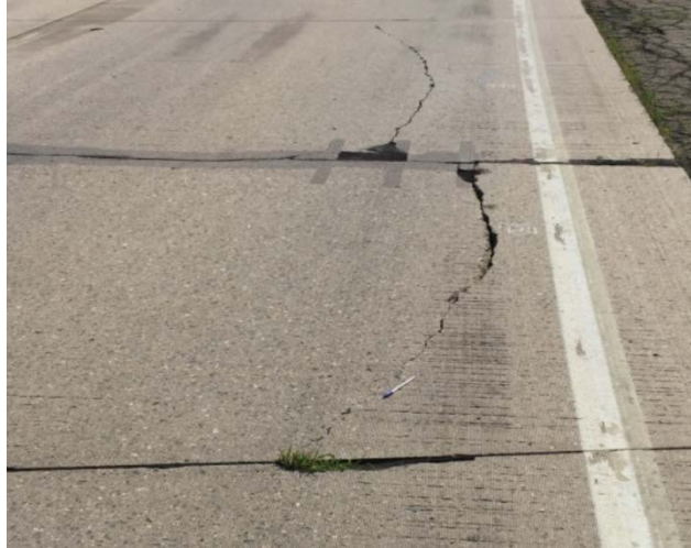
Figure 5 - Broken panels in Highway 60 East
