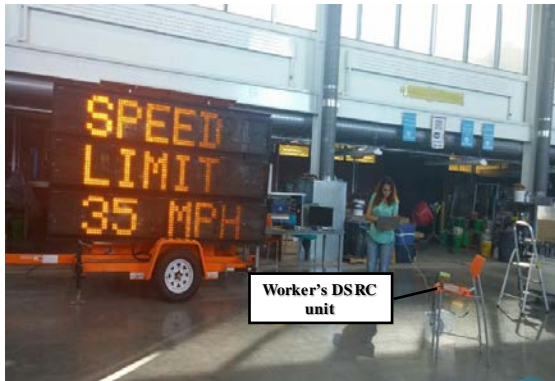
(a) DSRC unit connected to the VMS through serial connection.
