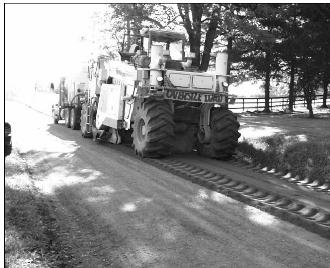
Figure 4. Full-Depth Reclaimer (Bushman et al. 2005)
