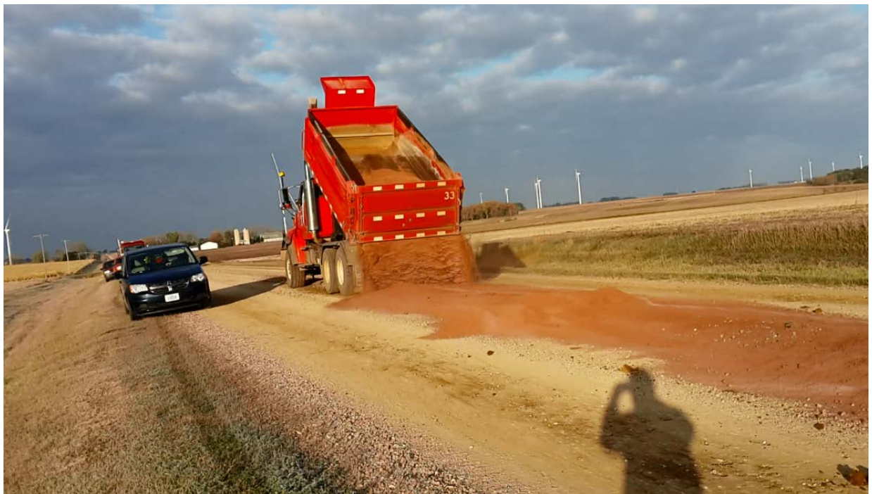
Figure 21. Spreading Additional Material at Jackson County Test Site
