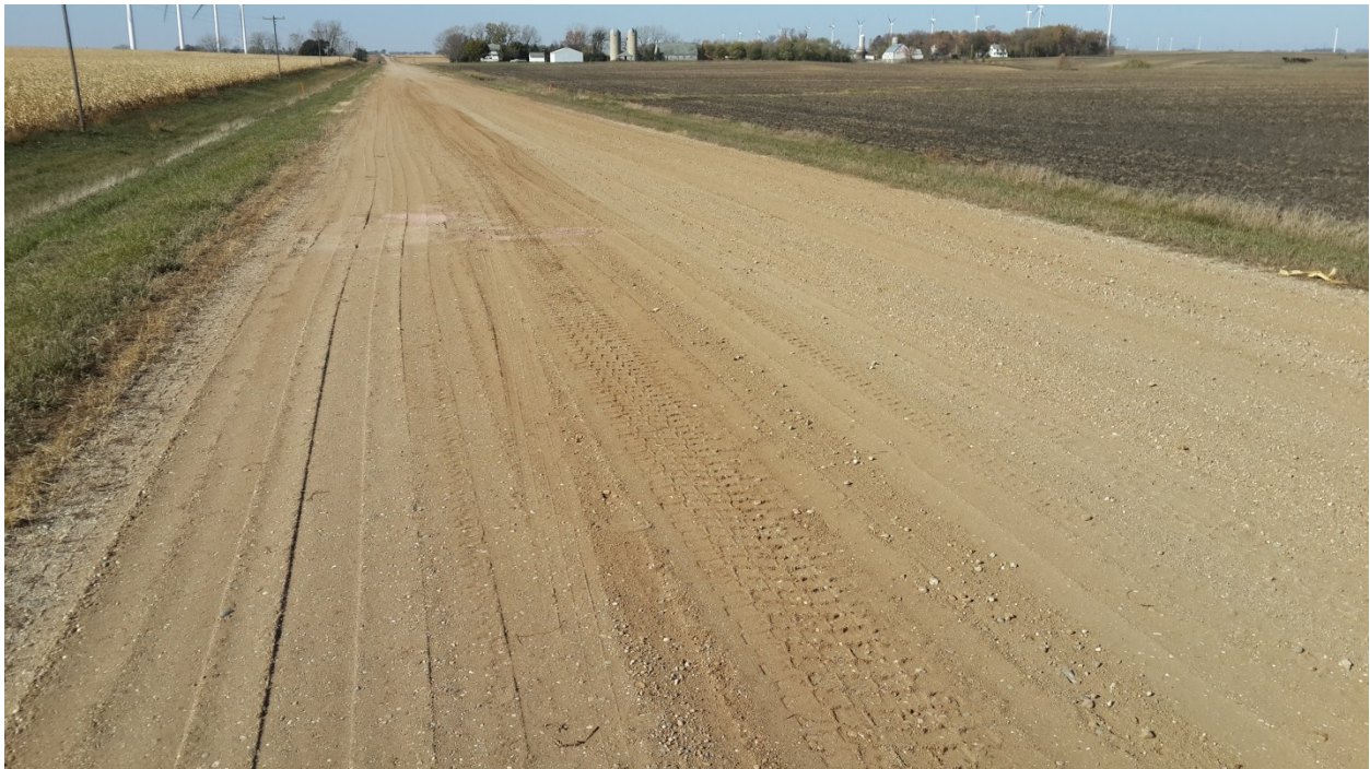
Figure 25. Jackson County CR 76 West Control Section (19 Tons of Standard Class 5 Aggregate)
