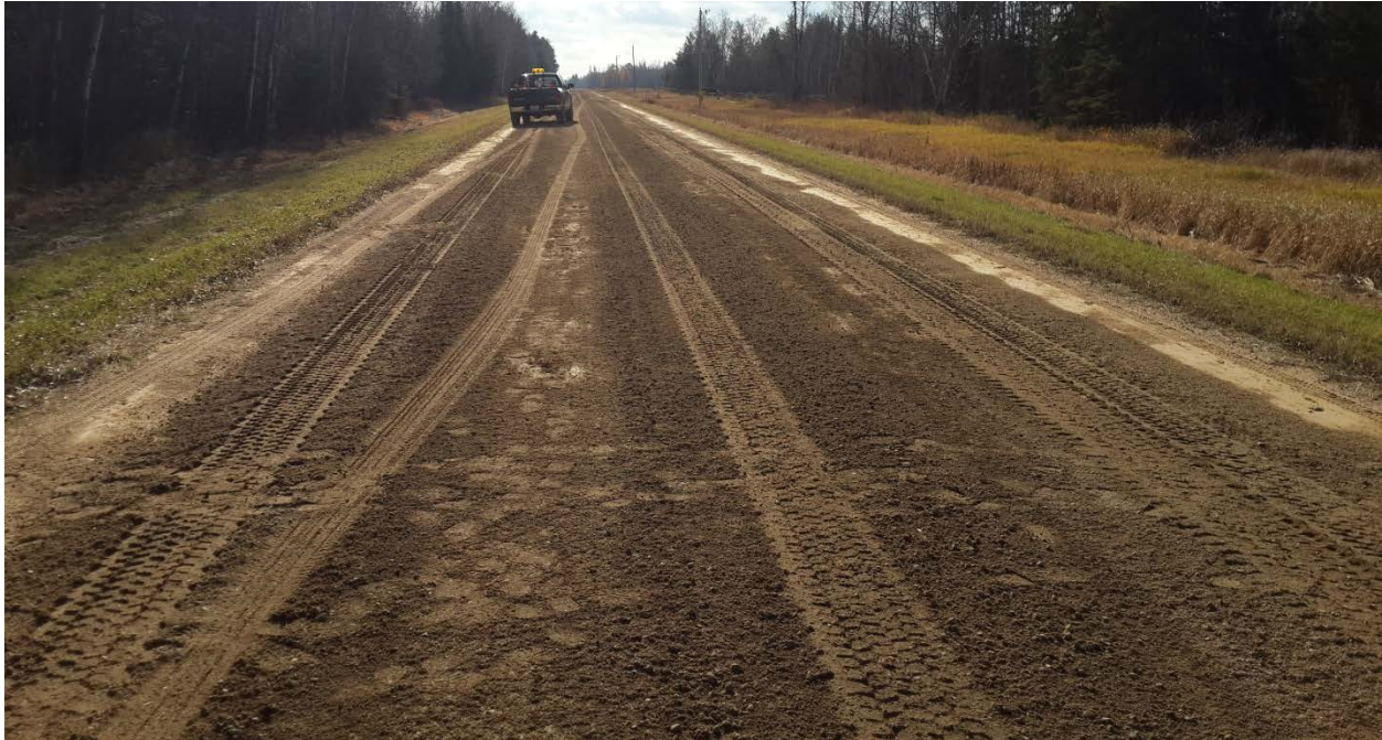
Figure 28. Beltrami County CR 23 North Control Section (166 Tons of Standard Class 1 Aggregate)
