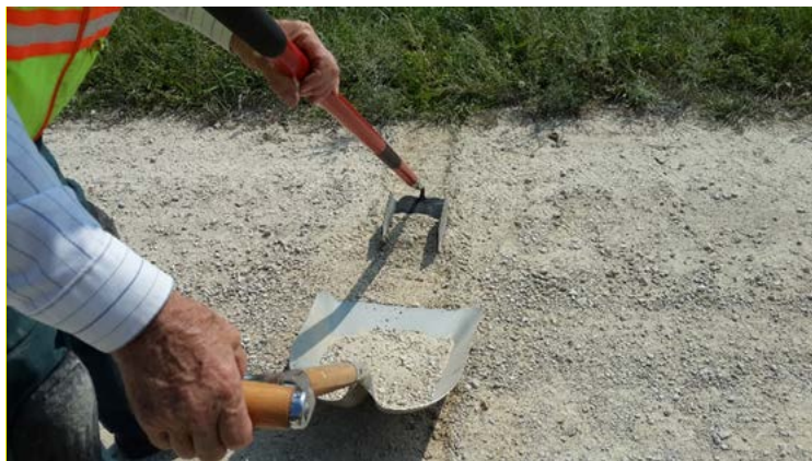
Figure 14. Loose Aggregate Collection
