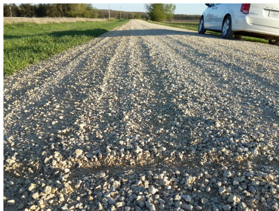
Figure 61. Extensive Floating Aggregate on the Surface of the Olmsted County CR 115 First South (Experimental) Section
