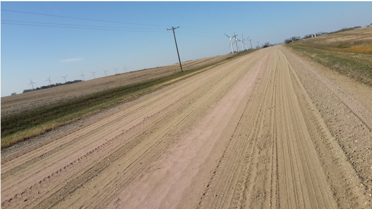
Figure 23. Jackson County CR 76 East Test Section (7 Tons of Crusher Dust)
