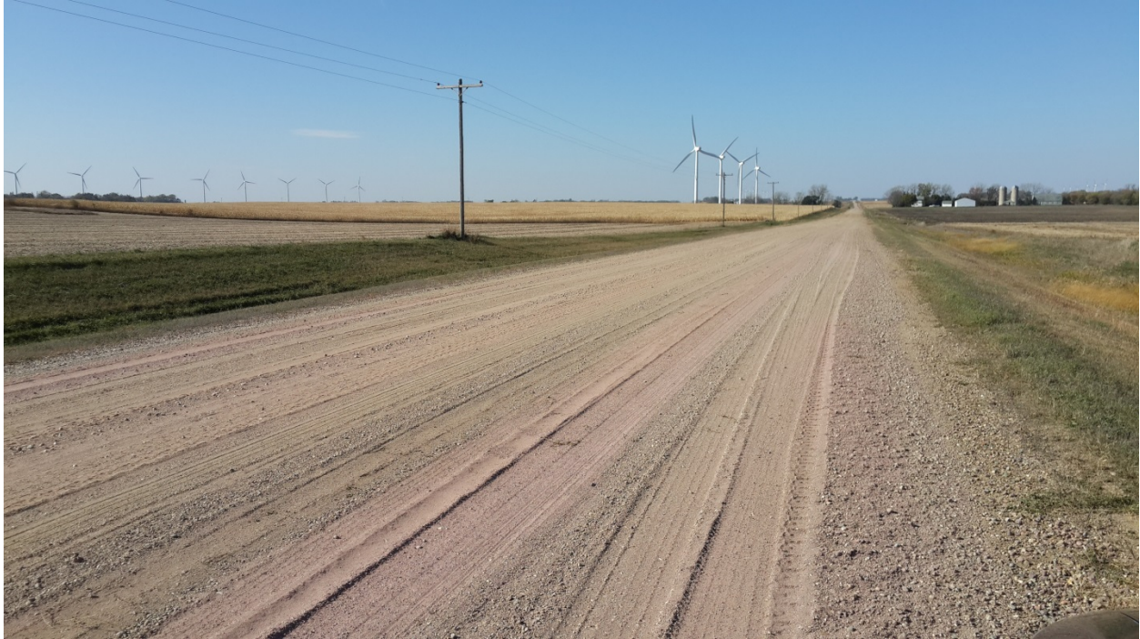
Figure 24 Jackson County CR 76 Middle Test Section (12 Tons of Crusher Dust)
