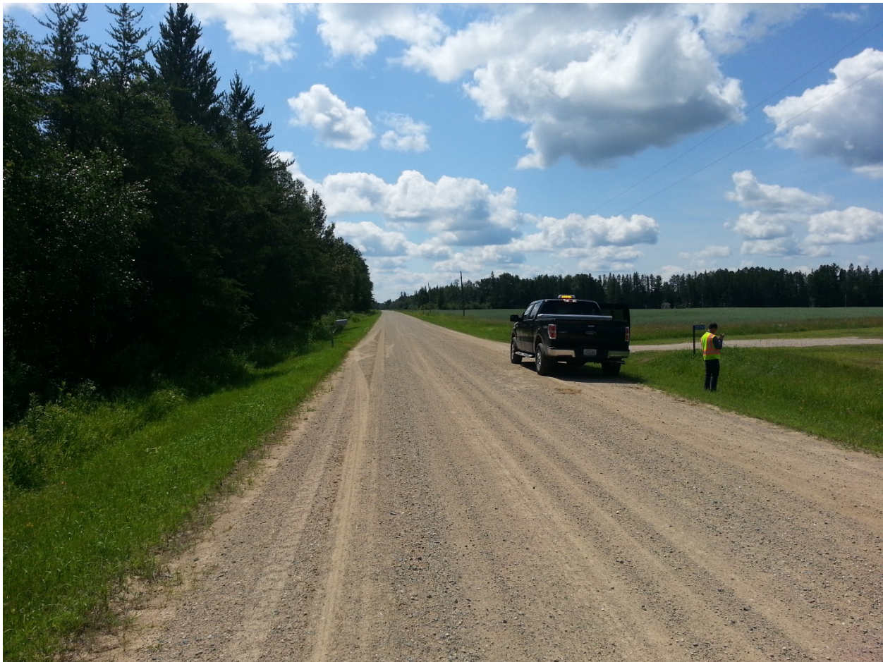
Figure 18. Beltrami County CR 23 Surface Conditions in July 2013
