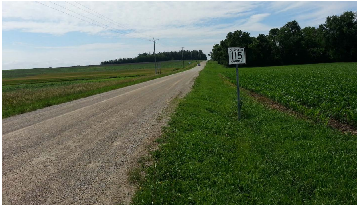
Figure 19. Olmsted County CR 115 Surface Conditions in July 2013
