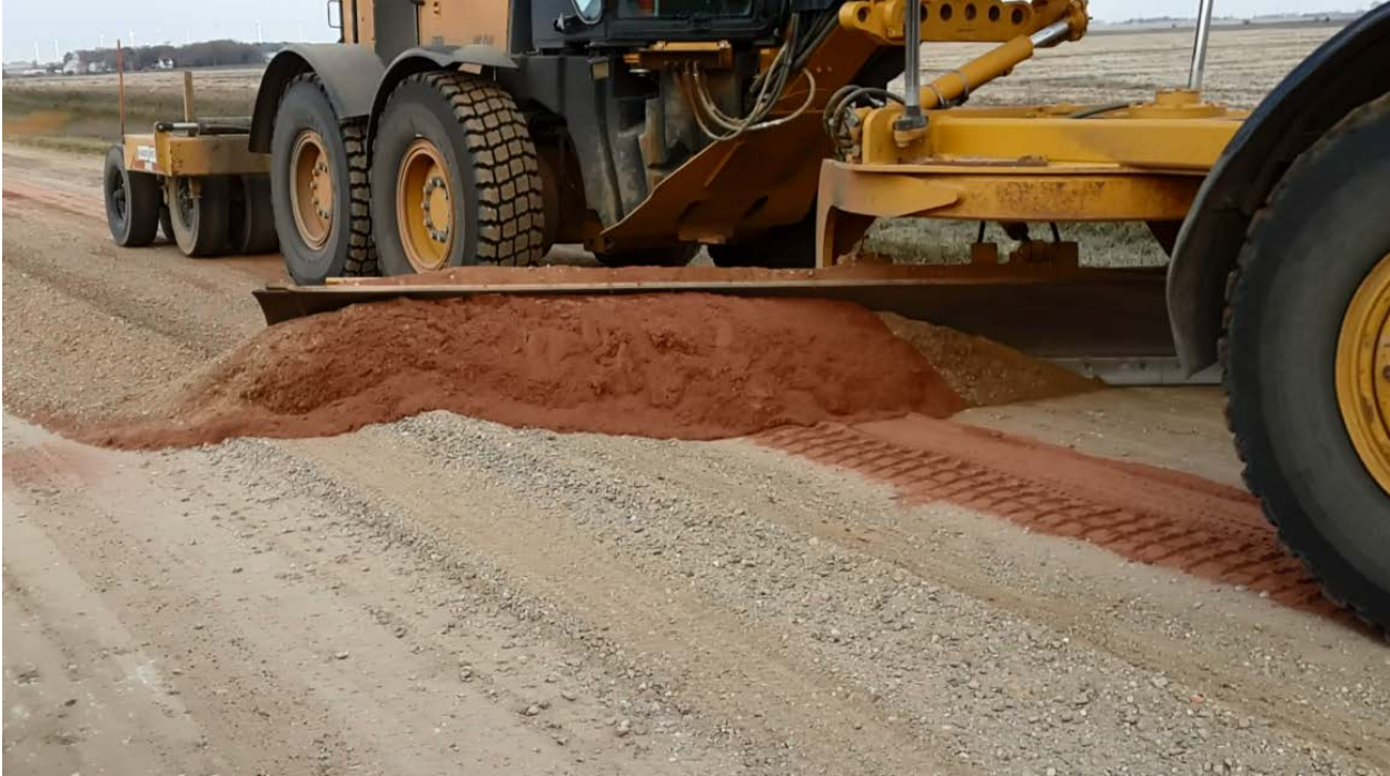
Figure 22. Blending Newly Added Material with Existing Material at Jackson County Test Site
