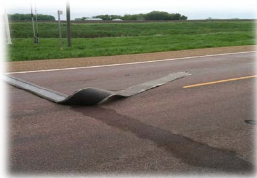
Figure 4-1: Weather Pulled Pads at Sibley County Test Location
