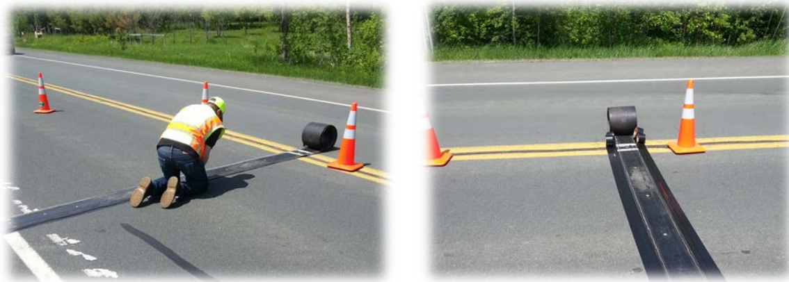
Figure 2-2: Photos of Pad Installation
