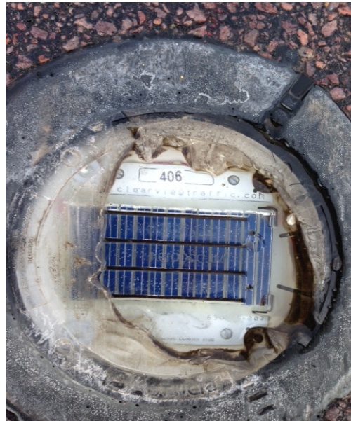
Damaged Stealth Stud
