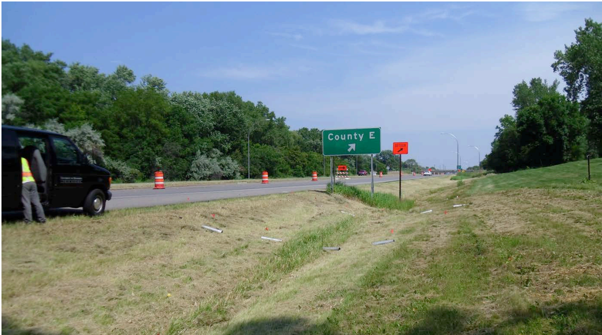
Figure 1. Roadside drainage ditch on Hwy 51 at off ramp to County Road E.
