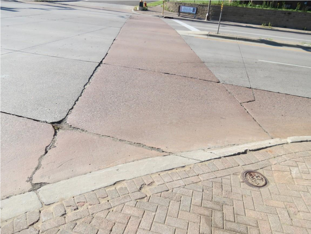
Figure 2.38 Roseville – Minor joint distress in colored concrete gutterline along Larpenteur Avenue W
