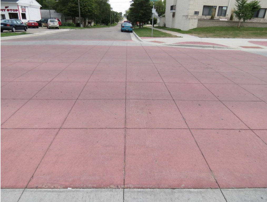
Figure 2.28 Detroit Lakes – Scraped surface, likely due to snow plow damage
