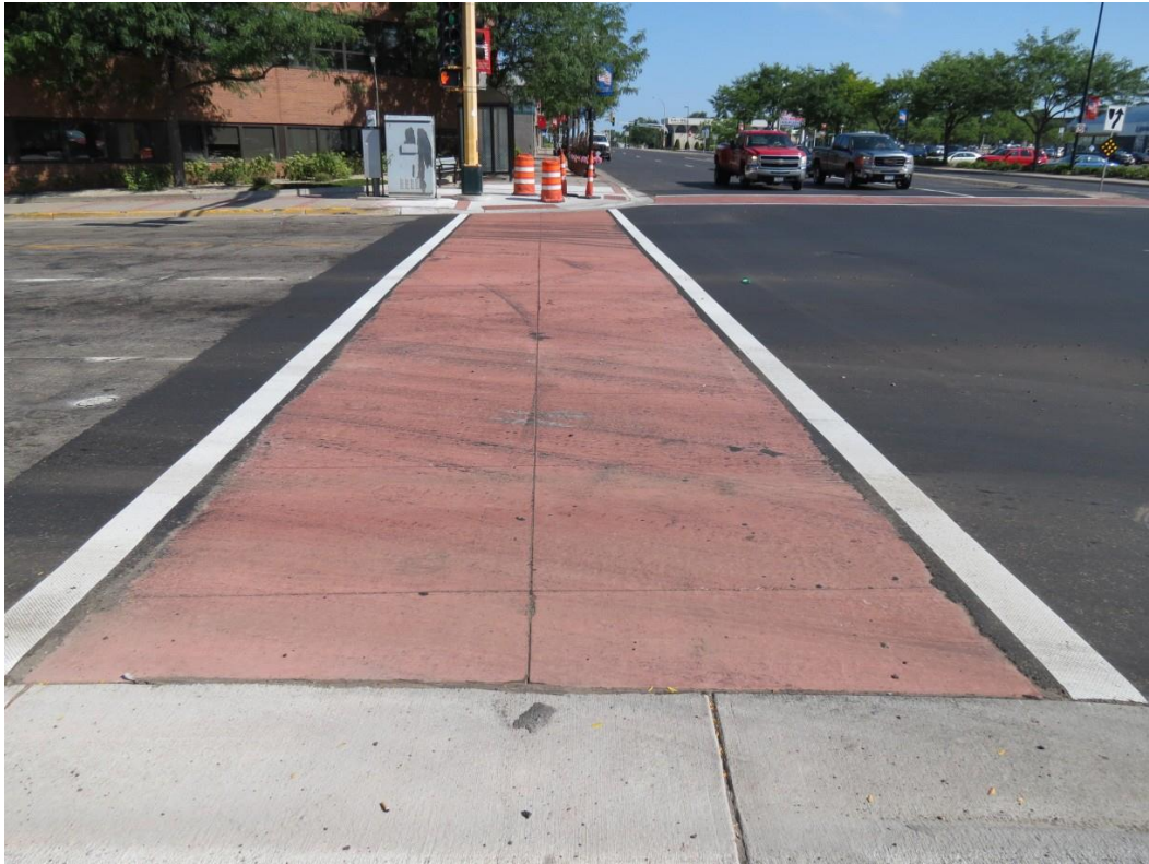
Figure 1.6 Colored concrete crosswalk in Sauk Rapids, MN
