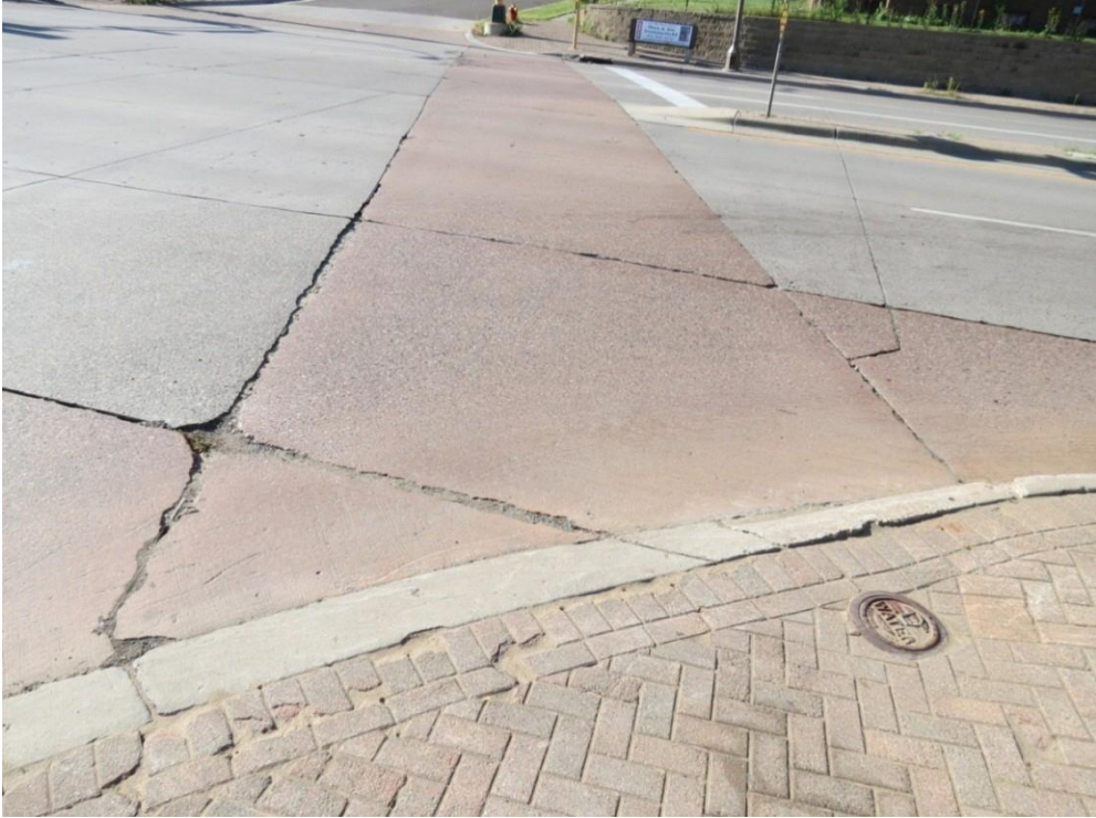
Figure 4.67 Distressed joints and panels in crosswalk at intersection of Larpenteur Avenue and N Fernwood Street
