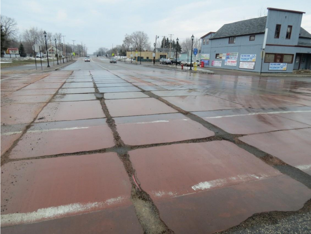
Figure 2.24 Centerville – Joint deterioration on County Road 14 at intersection with Progress Road
