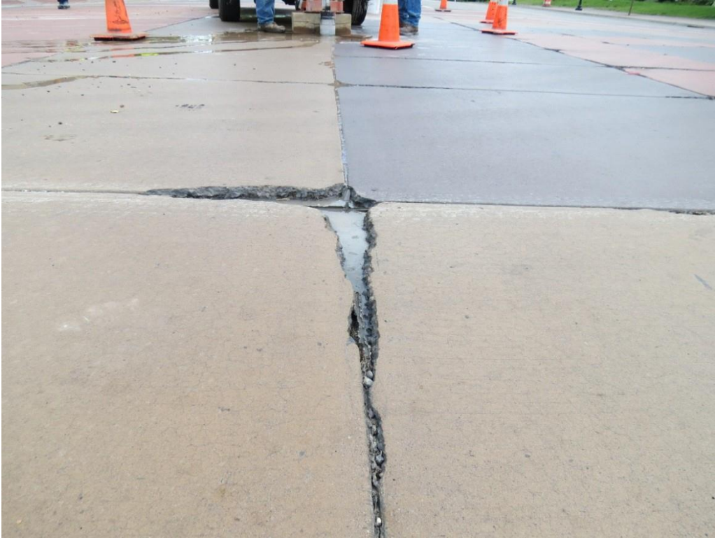
Figure 4.5 Keyed longitudinal joint between two different color sections
