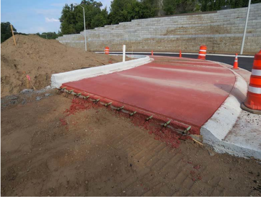
Figure 3.14 Previously placed colored concrete roundabout apron on West College Drive and 4 th Street S.W.
