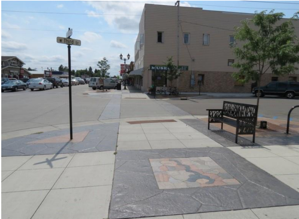
Figure 1.1 Sculpted and colored concrete sidewalks in Park Rapids, MN
