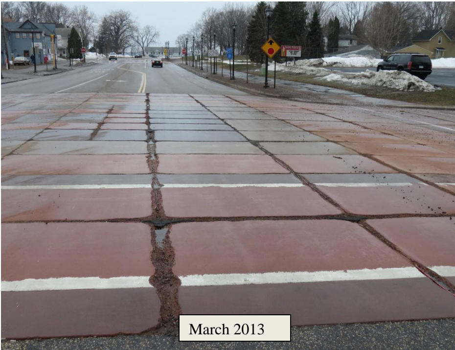
Figure 4.2 Typical joint deterioration occurring in colored concrete intersection of County Highway 14 (Main Street) and Progress Road in Centerville, MN
