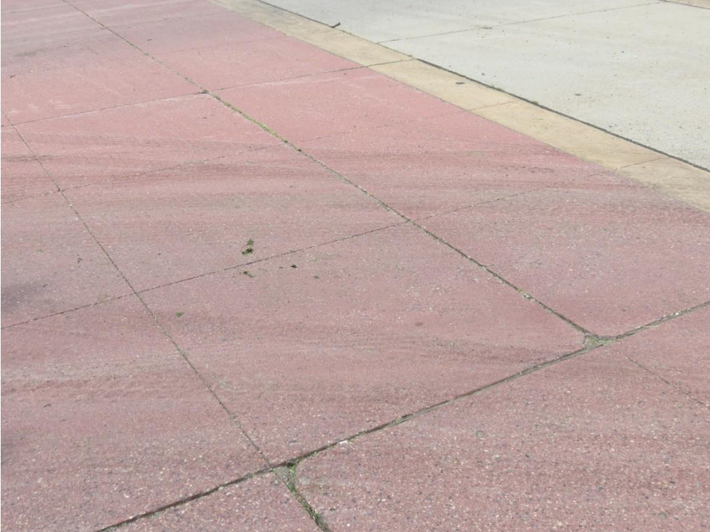
Figure 2.53 St. Paul – Joint distress in crosswalk at intersection of Shepard Road and Washington Street
