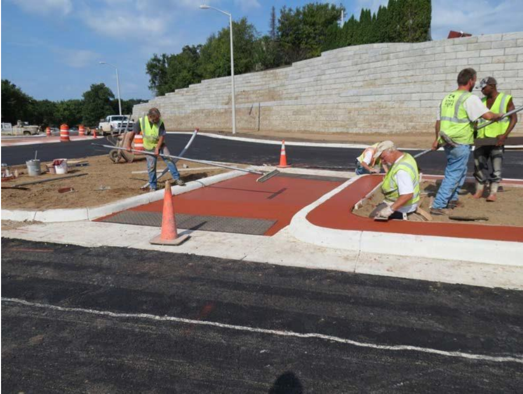
Figure 3.13 Applying broom texture to colored concrete sidewalk in Brainerd
