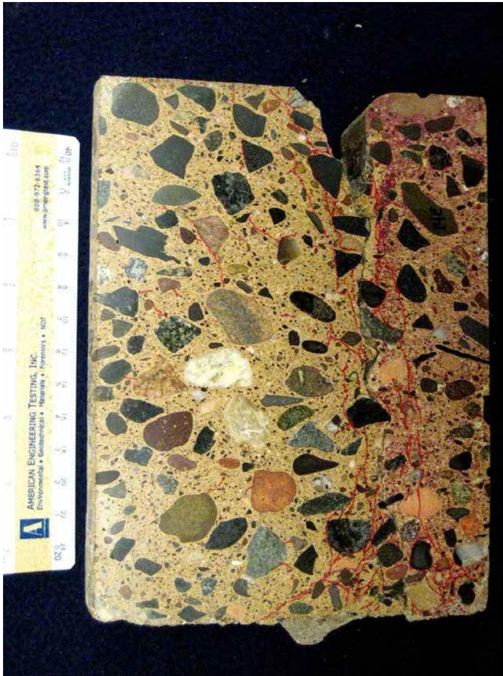
Figure 4.22 Centerville - Vertical cracking in Core 14E, highlighted by red ink
