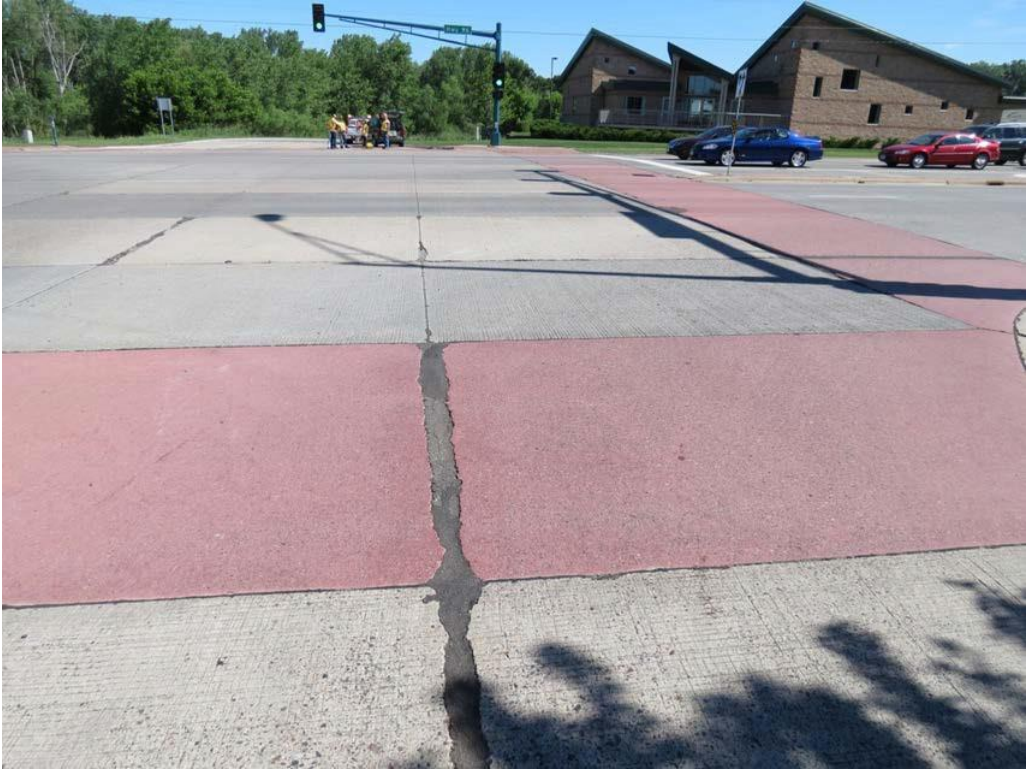
Figure 4.29 Joint and panel deterioration occurring in colored concrete crosswalks at intersection of County Highway 96 and Greenhaven Drive in Vadnais Heights, MN
