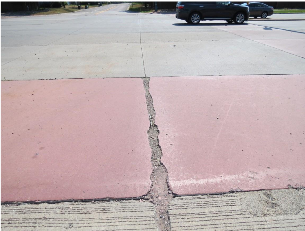
Figure 2.49 Vadnais Heights – Extensive joint distress in crosswalk at intersection of County Highway 96 West and Greenhaven Drive
