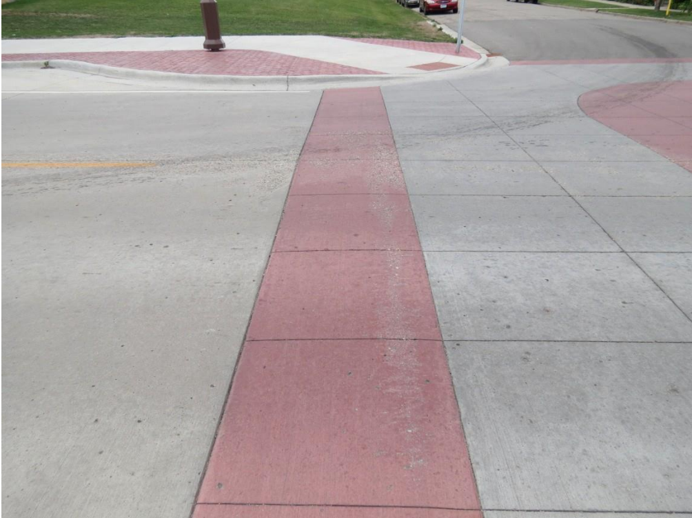
Figure 2.28 Detroit Lakes – Scraped surface, likely due to snow plow damage
