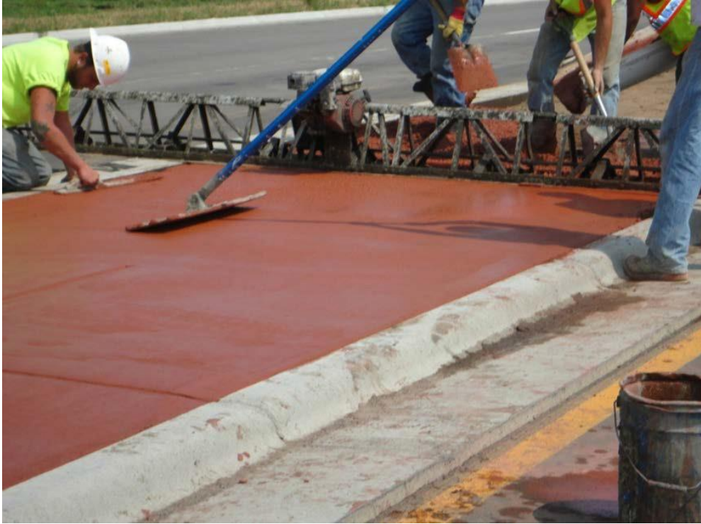
Figure 3.9 Colored concrete median construction using vibrating screed across in-place curbs
