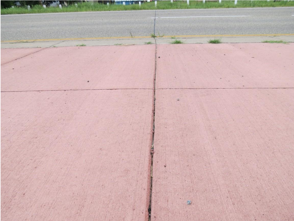
Figure 2.12 Blaine – Joints in median on Radisson Road
