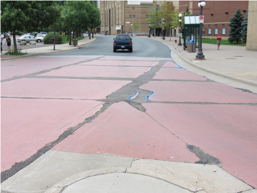
Figure 2.60 Stillwater – Panel cracking in new colored concrete crosswalk at intersection of Main Street North and Commercial Street
