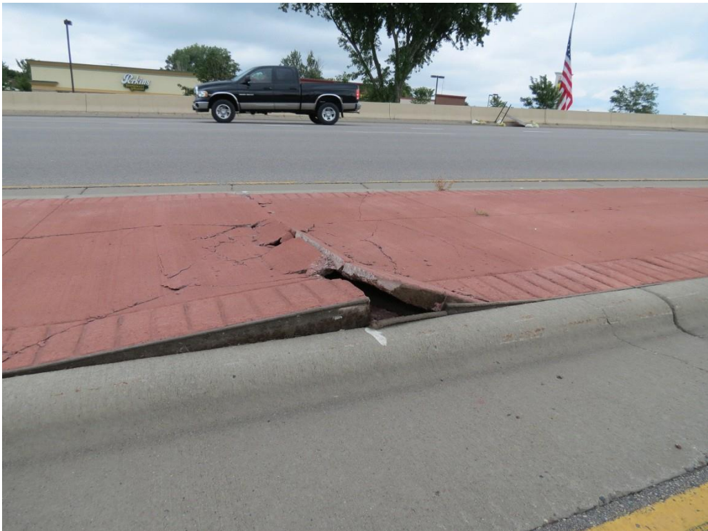
Figure 2.17 Blaine – Buckling in median within County Rd 14
