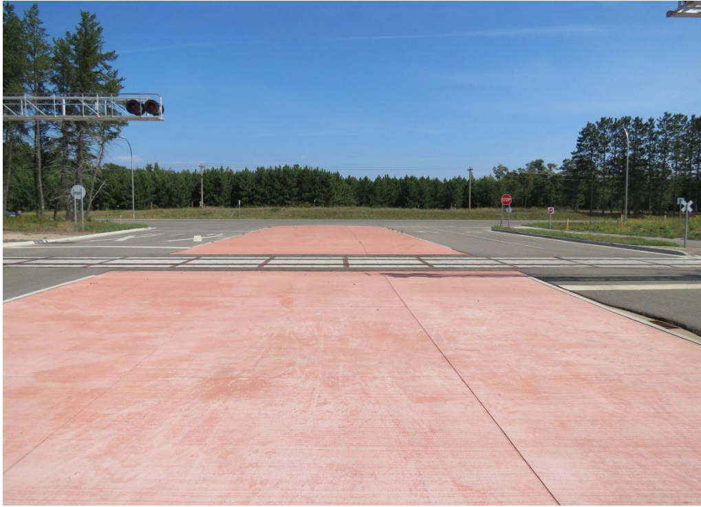
Figure 2.10 Baxter - Median near railroad crossing on Timberwood Drive and TH210
