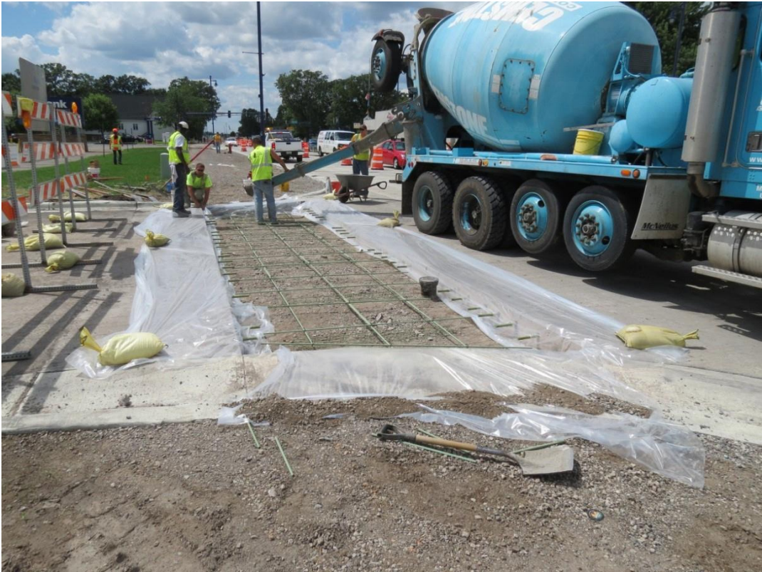
Figure 3.3 Crosswalk area prepared for placement of colored concrete
