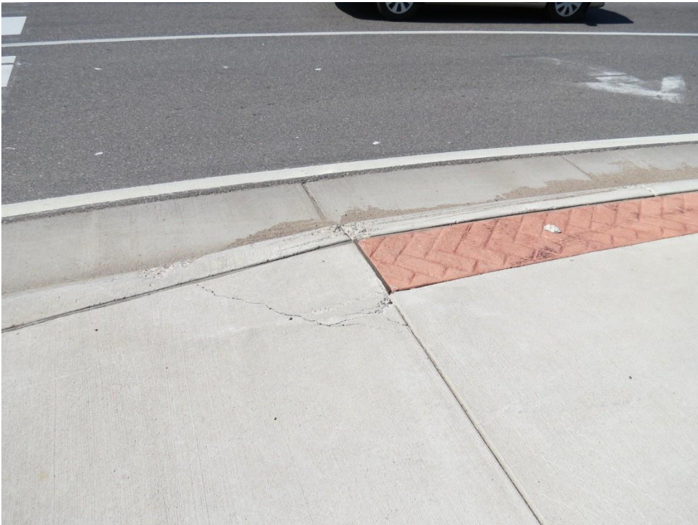
Figure 2.34 Princeton – Crack at end of colored concrete boulevard strip
