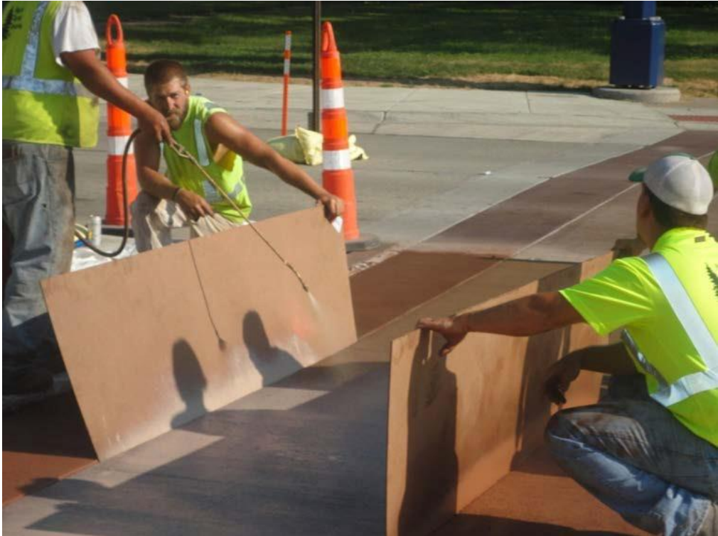
Figure 3.1 Workers holding thin board to apply Lithochrome Colorwax
