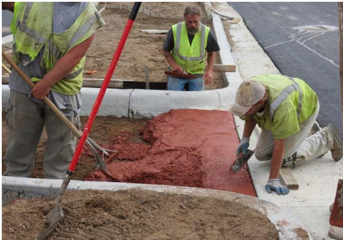
Figure 3.12 Placement of colored concrete sidewalk in Brainerd
