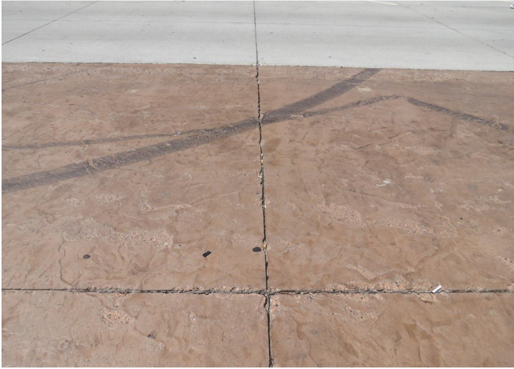
Figure 2.32 Park Rapids – Crack in sidewalk, likely due to different thermal expansion/contraction rates
