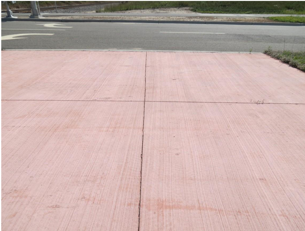
Figure 2.11 Baxter – Joints in median on Timberwood Drive
