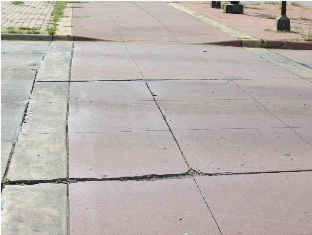
Figure 2.55 St. Paul – Joint distress in crosswalk at intersection of Shepard Road and Old Chestnut Street
