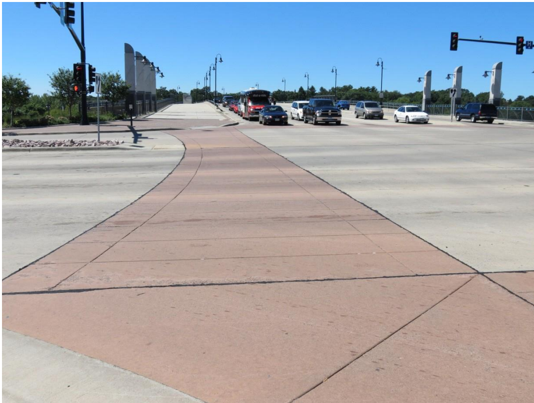
Figure 1.6 Colored concrete crosswalk in Sauk Rapids, MN
