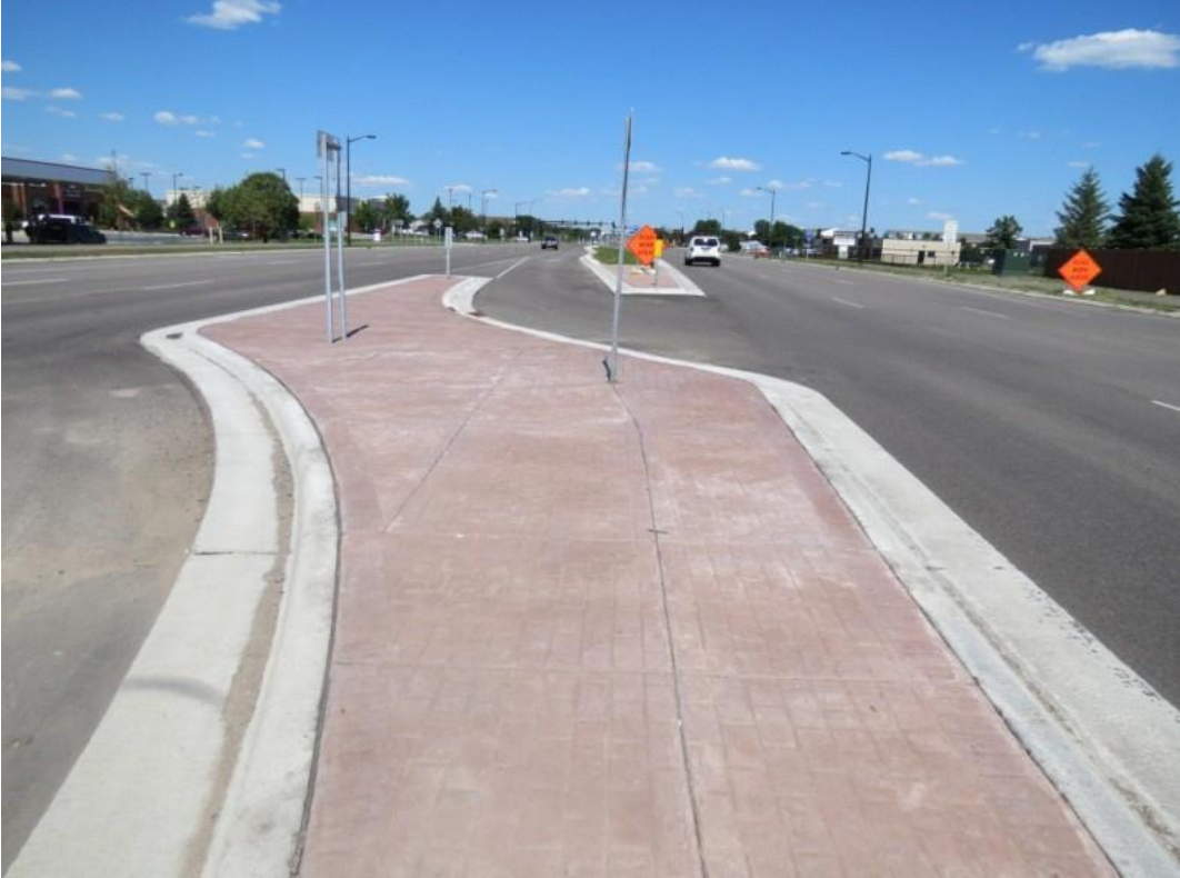
Figure 1.4 Colored concrete intersection in Centerville, MN
