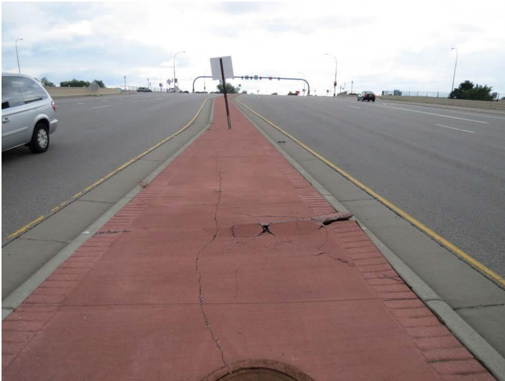
Figure 2.17 Blaine – Buckling in median within County Rd 14
