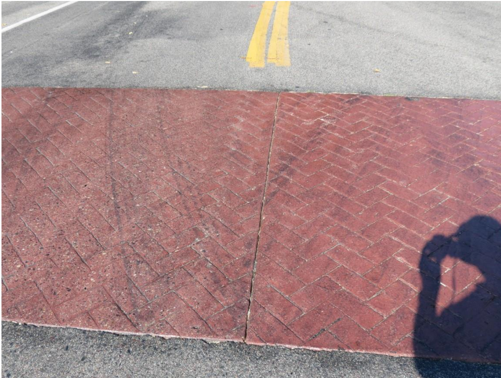
Figure 2.39 Roseville – Colored concrete crosswalk in good condition at intersection of Josephine Road and Lexington Avenue
