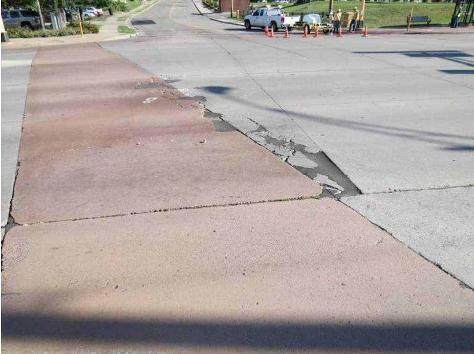
Figure 4.67 Distressed joints and panels in crosswalk at intersection of Larpenteur Avenue and N Fernwood Street
