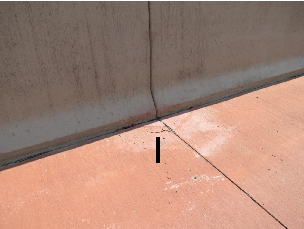
Figure 2.30 Minneapolis – Cracking, likely due to thermal expansion/restraint
