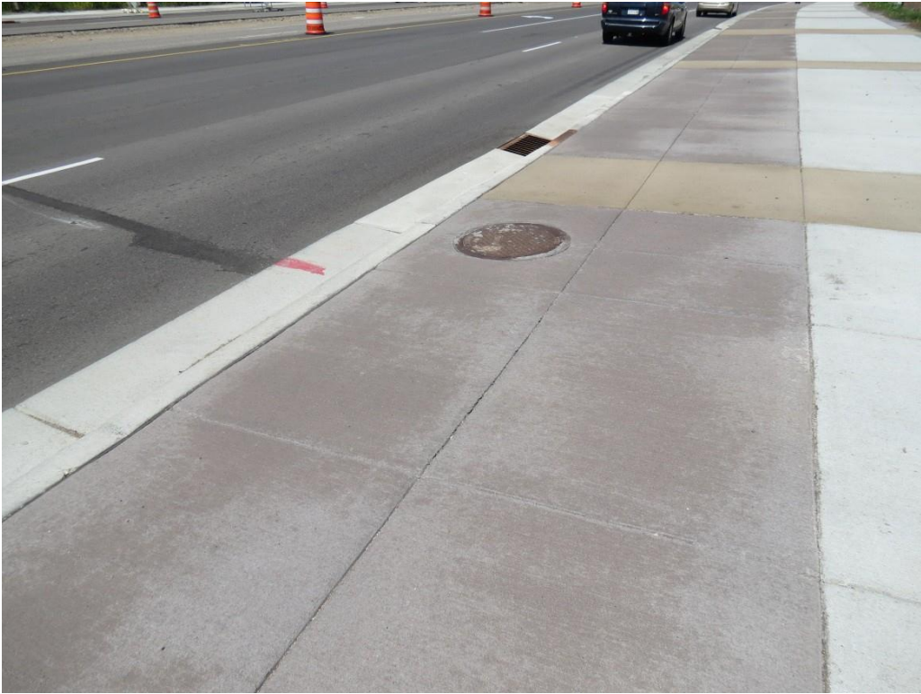
Figure 2.2 Apple Valley – Sidewalk along Cedar Avenue near 153 rd Street W
