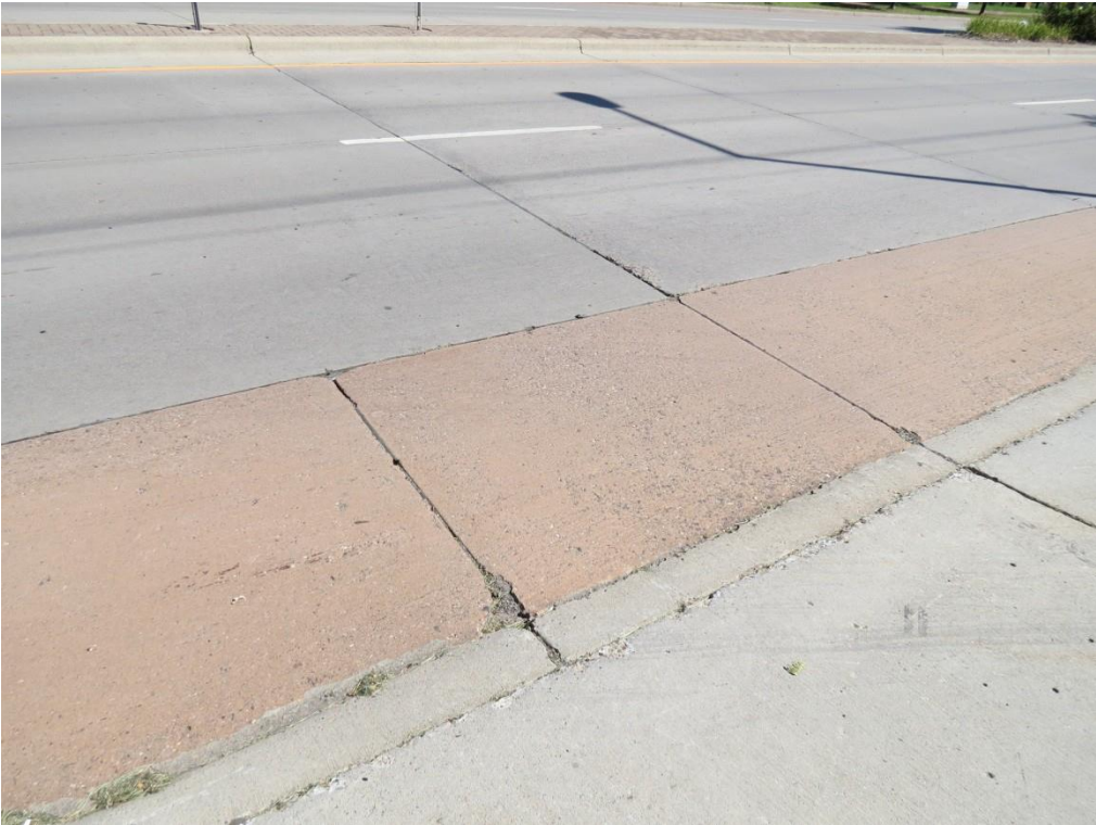
Figure 2.38 Roseville – Minor joint distress in colored concrete gutterline along Larpenteur Avenue W
