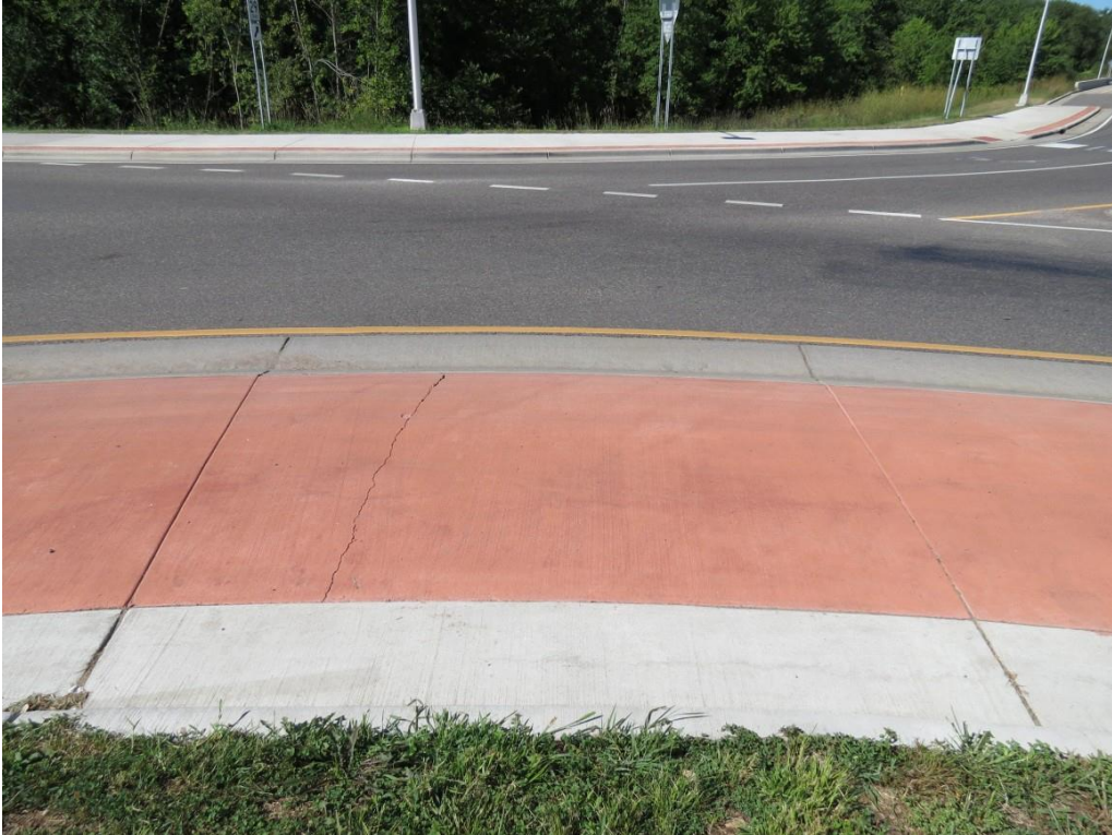
Figure 2.34 Princeton – Crack at end of colored concrete boulevard strip
