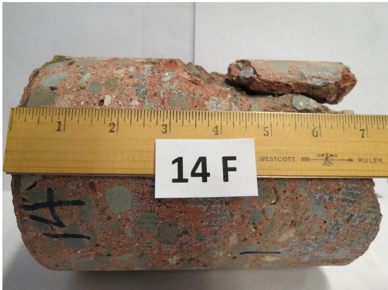
Figure 4.26 Centerville - Core sample 14F showing possible deterioration within neighboring joint
