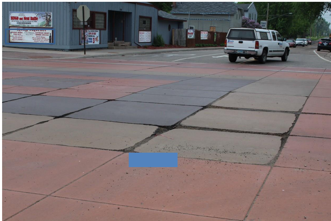
Figure 8.6 Accelerated joint deterioration occurring throughout intersection. The potential for continuing distress at new joint faces (created during repair process) necessitates full-depth slab replacement.
