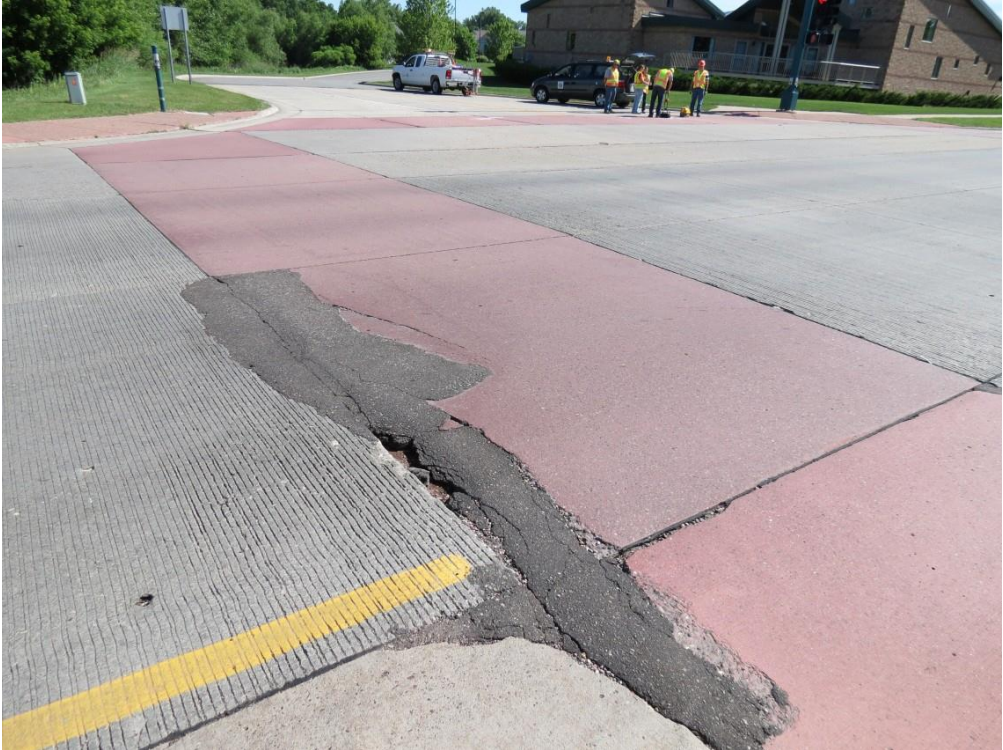
Figure 4.29 Joint and panel deterioration occurring in colored concrete crosswalks at intersection of County Highway 96 and Greenhaven Drive in Vadnais Heights, MN
