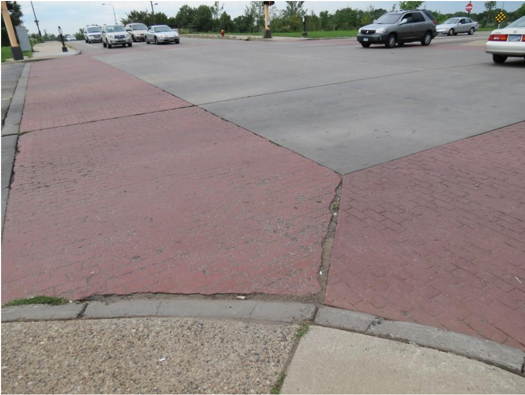
Figure 2.51 St. Paul – Noticeable wear on surface of colored concrete crosswalk at intersection of Phalen Boulevard and Payne Avenue
