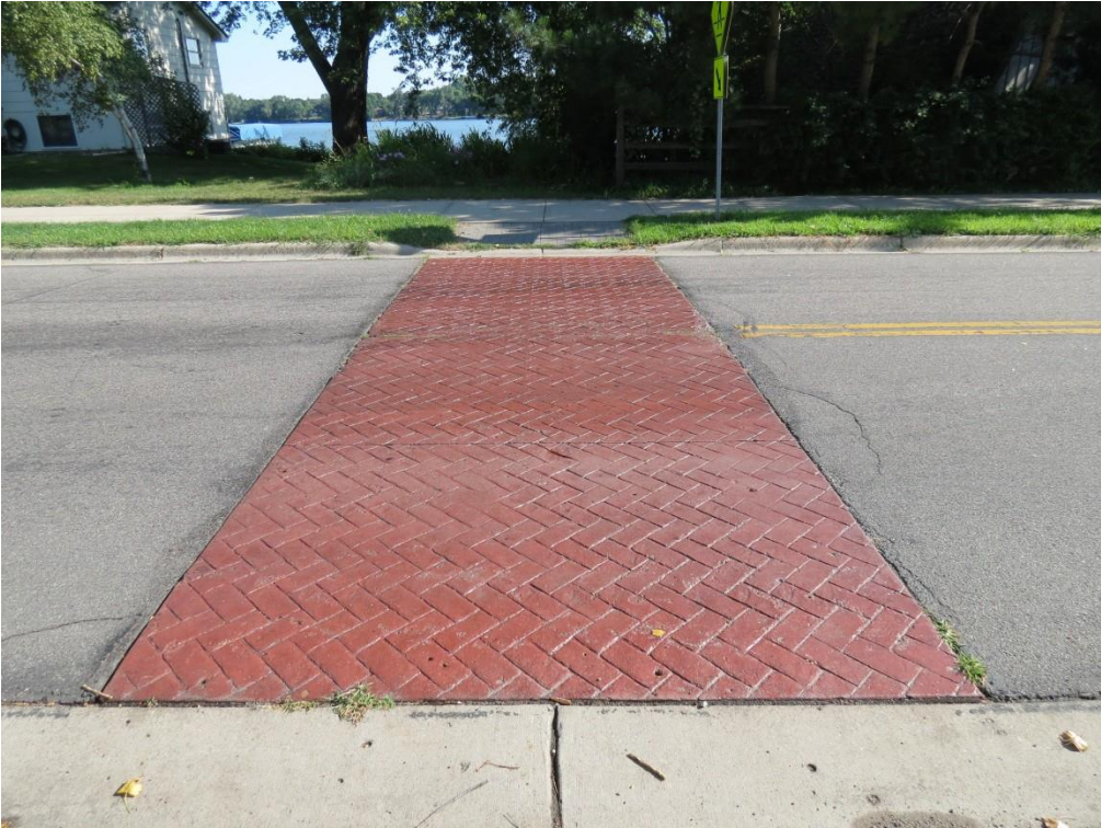
Figure 2.40 Roseville – Colored concrete crosswalk in good condition across Josephine Road near Fernwood Street N
