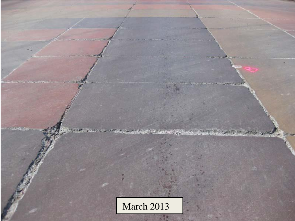
Figure 4.2 Typical joint deterioration occurring in colored concrete intersection of County Highway 14 (Main Street) and Progress Road in Centerville, MN
