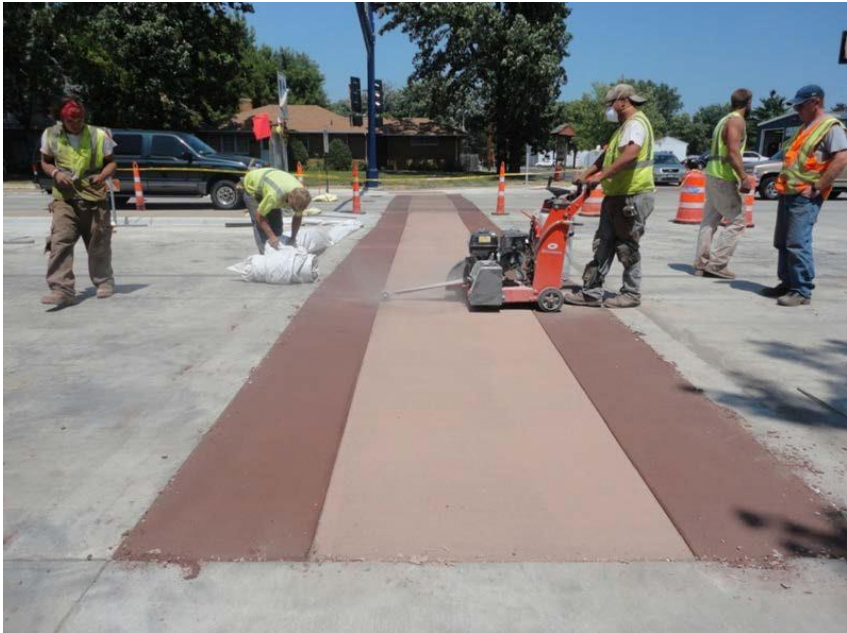
Figure 3.2 Transverse joints being sawed into colored concrete crosswalk
