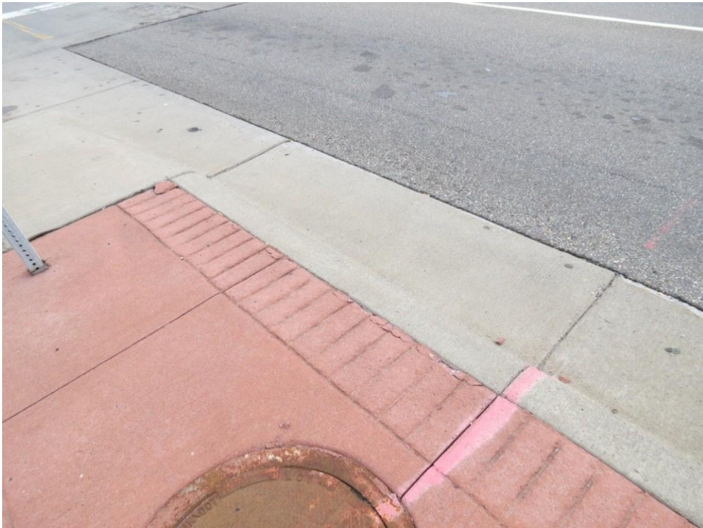
Figure 6.6 Expansion of slab near surface, due to temperature gradients, may lead to surface spalling near the edge of panels
