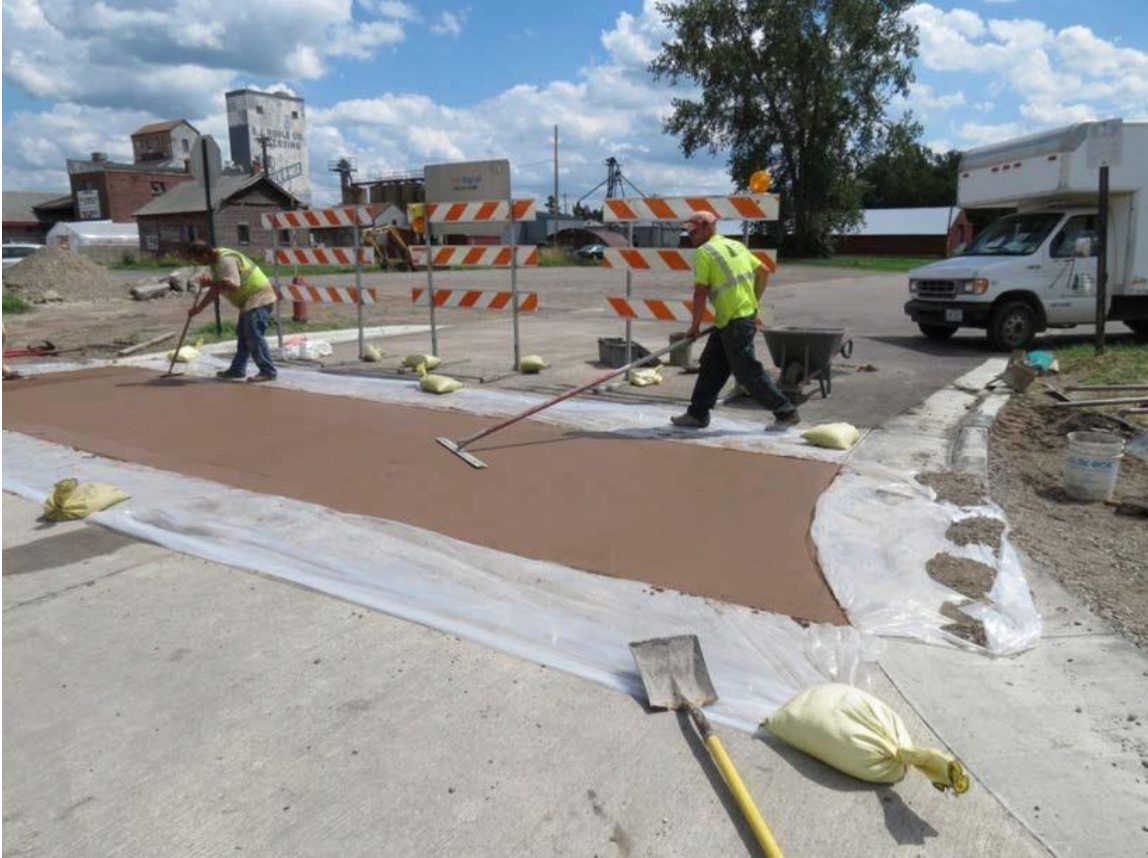
Figure 3.5 Finishing colored concrete surface (step 2 after leveling)
