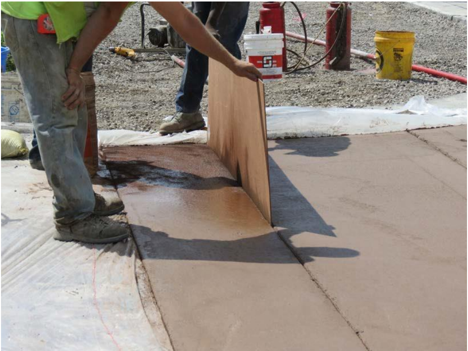
Figure 3.7 Sprinkling darker colored powdered pigment on outer portions of crosswalk
