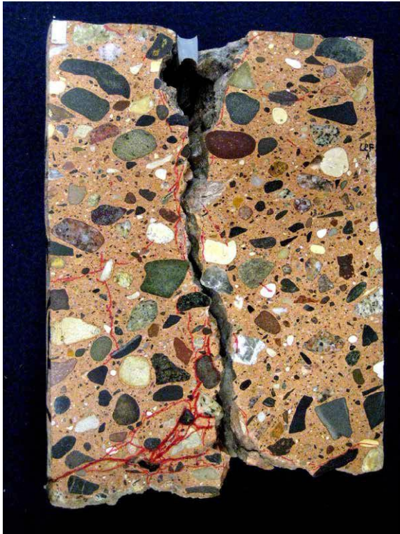
Figure 4.74 Roseville - Core sample L&F-A showing vertical and horizontal microcracking (highlighted in red ink)
