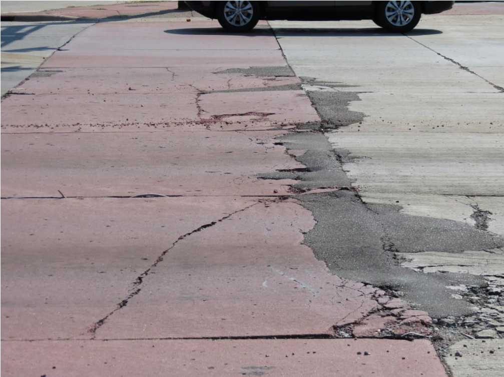
Figure 2.47 Vadnais Heights – Severe panel distress in crosswalk at intersection of County Highway 96 West and Village Center Drive
