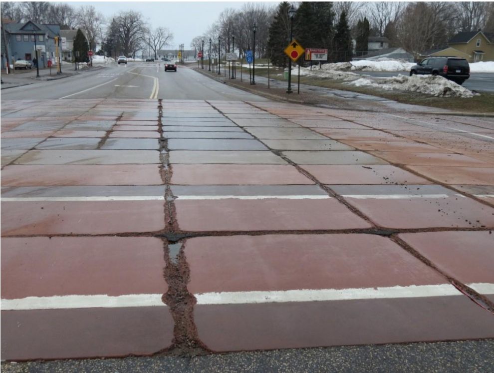
Figure 2.24 Centerville – Joint deterioration on County Road 14 at intersection with Progress Road
