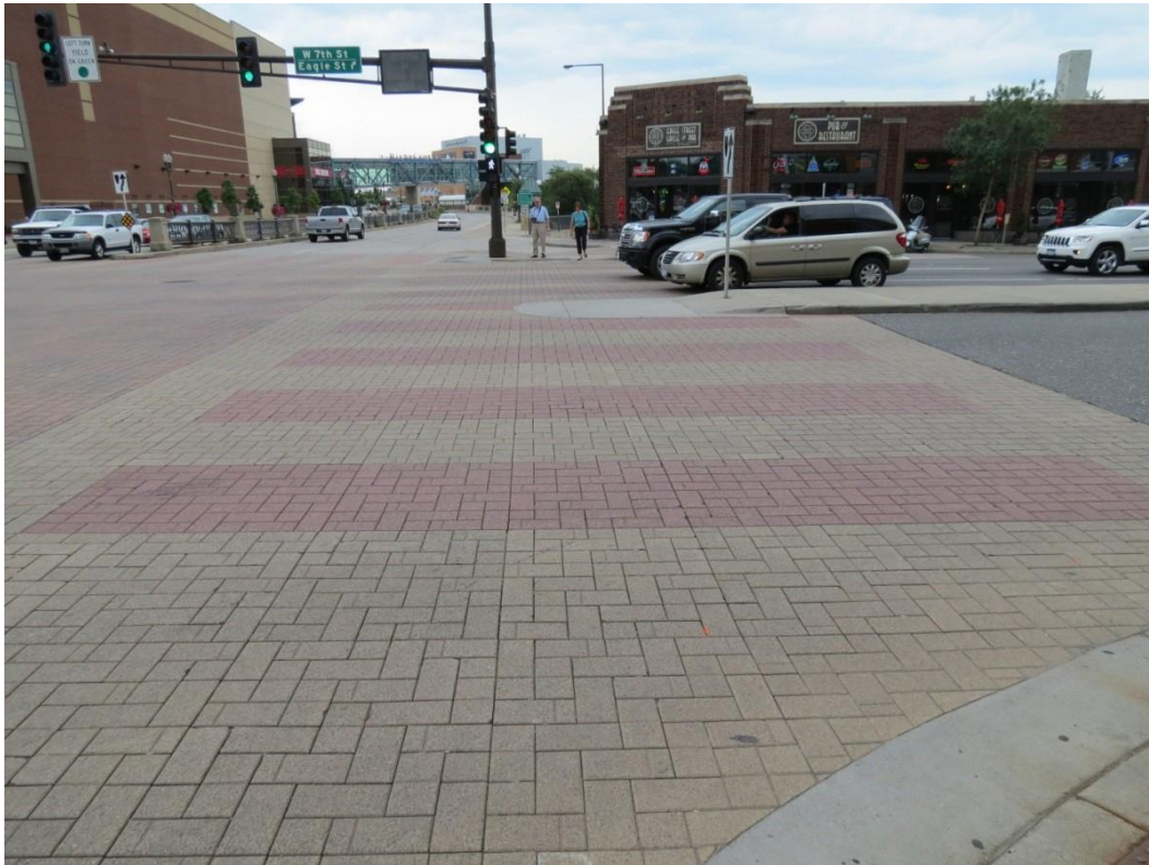
Figure 8.7 Interlocking concrete paver system in St. Paul, MN intersection.
