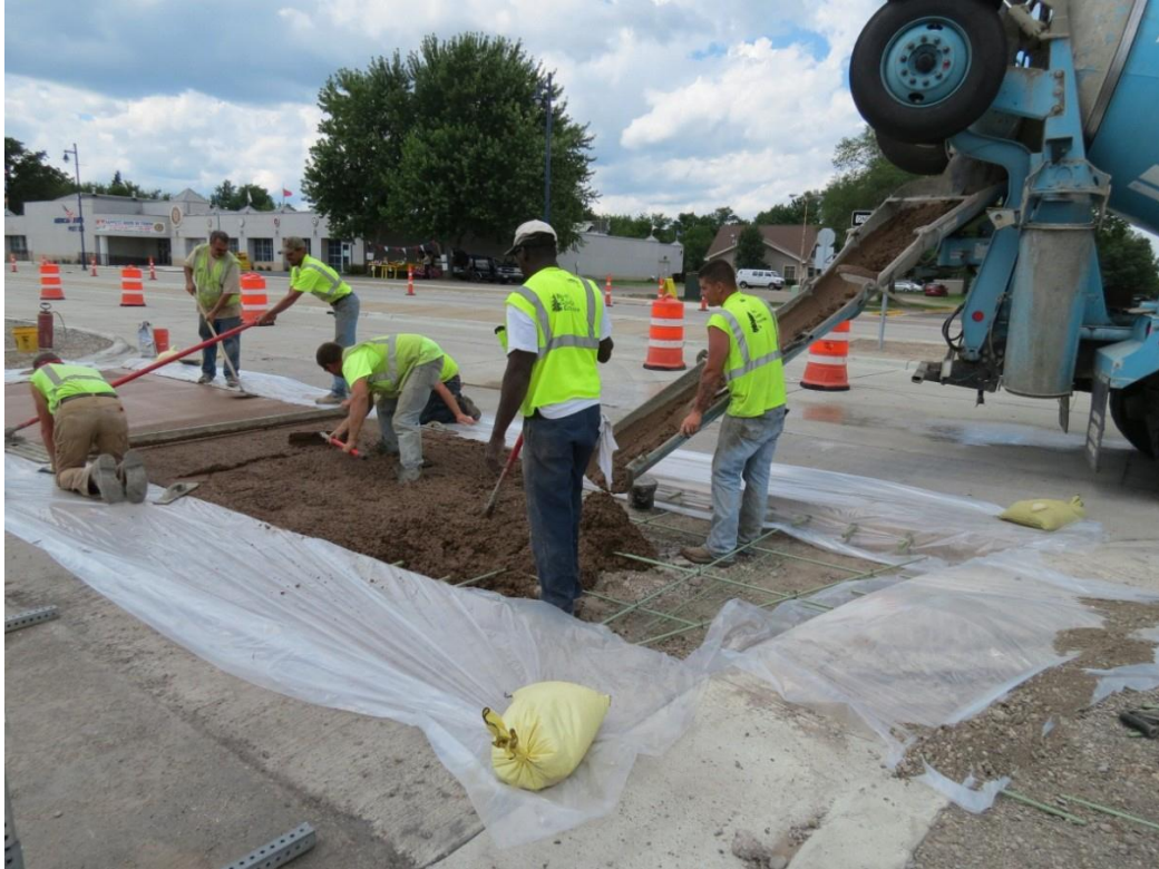
Figure 3.4 Placement of colored concrete in crosswalk area
