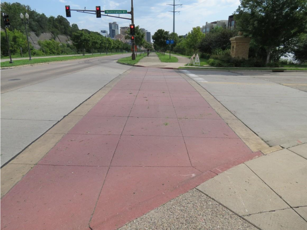
Figure 2.53 St. Paul – Joint distress in crosswalk at intersection of Shepard Road and Washington Street
