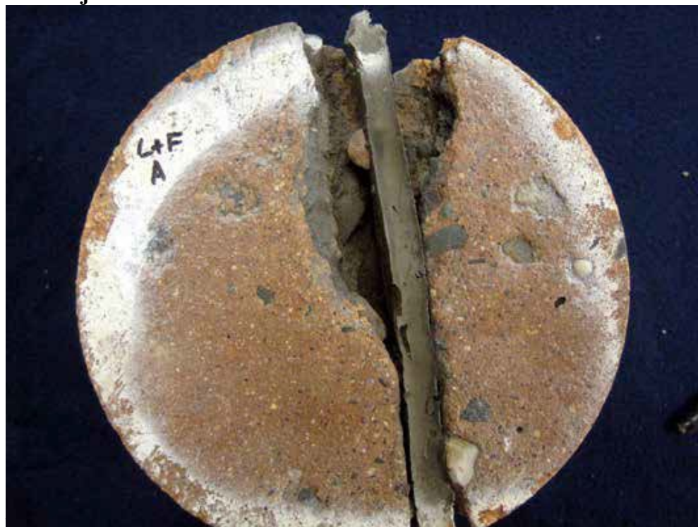
L&F A DESCRIPTION: Carbonation (unstained paste) proceeds up to 10mm depth from
