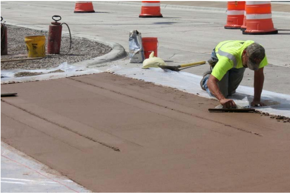
Figure 3.7 Sprinkling darker colored powdered pigment on outer portions of crosswalk
