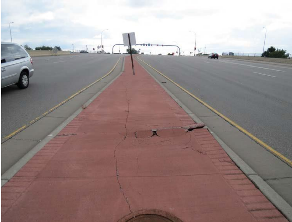
Figure 8.6 Accelerated joint deterioration occurring throughout intersection. The potential for continuing distress at new joint faces (created during repair process) necessitates full-depth slab replacement.
