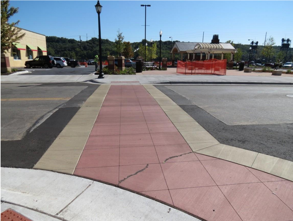
Figure 2.60 Stillwater – Panel cracking in new colored concrete crosswalk at intersection of Main Street North and Commercial Street
