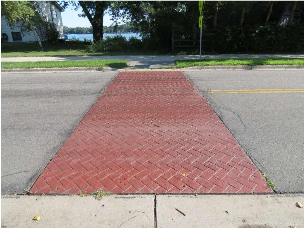
Figure 1.7 Colored concrete crosswalk in Roseville, MN
