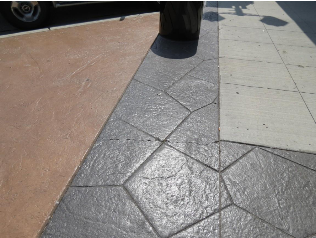
Figure 2.32 Park Rapids – Crack in sidewalk, likely due to different thermal expansion/contraction rates
