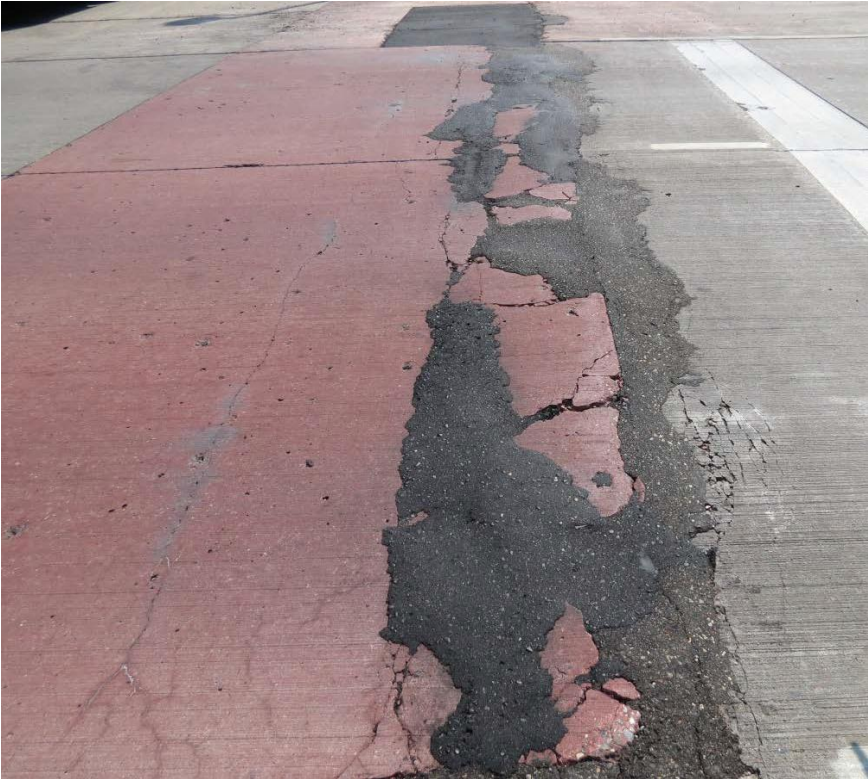
Figure 2.47 Vadnais Heights – Severe panel distress in crosswalk at intersection of County Highway 96 West and Village Center Drive
