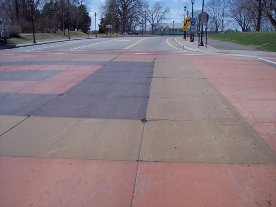
Figure 1.4 Colored concrete intersection in Centerville, MN
