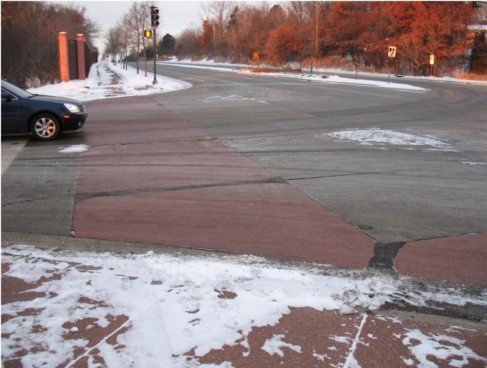
Figure 2.49 Vadnais Heights – Extensive joint distress in crosswalk at intersection of County Highway 96 West and Greenhaven Drive
