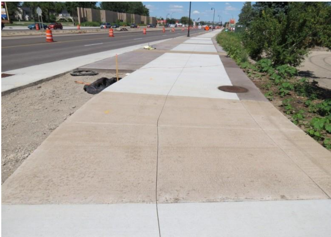
Figure 1.2 Colored concrete sidewalks in Apple Valley, MN
